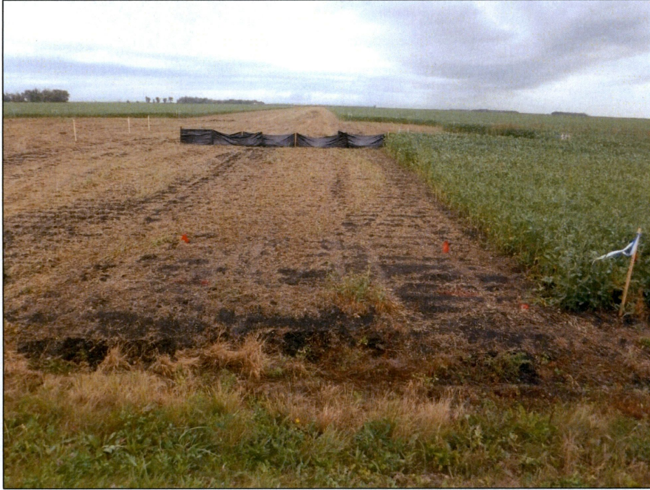
Figure 21. Silt fence installed at Station 337+00, looking north.
