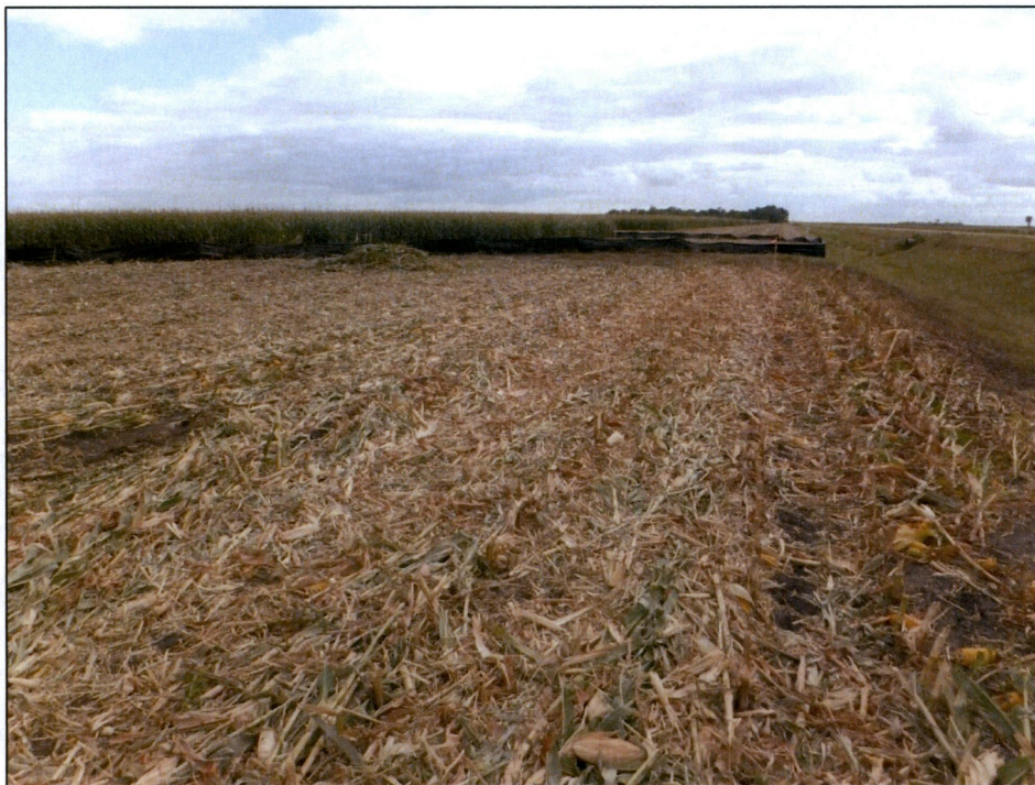
Figure 18. Outfall 008, silt fence installed at Station 233+00 (foreground), looking south.
