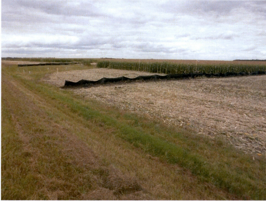
Figure 19. Outfall 008, silt fence installed at Station 236+00 (foreground), looking north.
