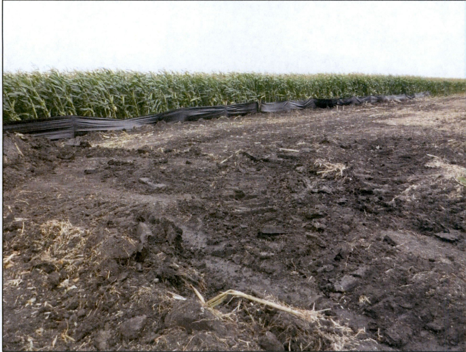
Figure 11. Silt fence installed from Station 141+00 to Station 144+00, looking southwest.
