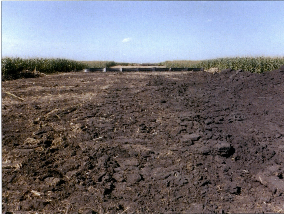
Figure 5. Outfall 002, silt fence on the south side (foreground) of the Lower Branch Rush River, looking north.
