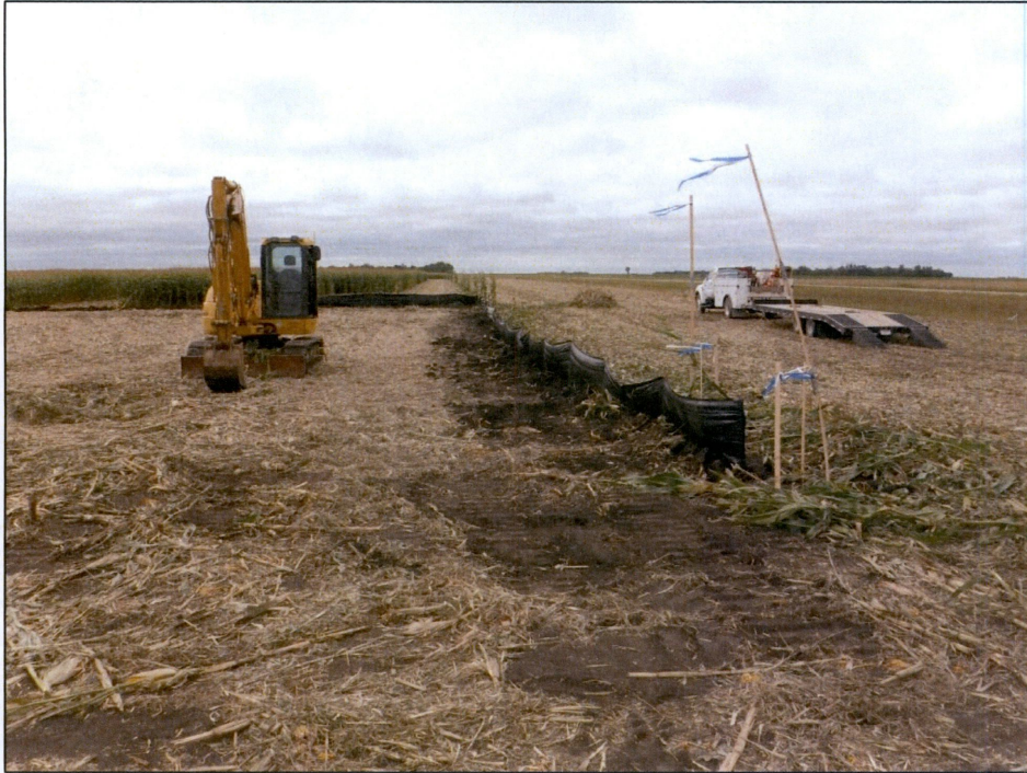
Figure 15. Outfall 007, silt fence installed at Station 225+00, looking south.
