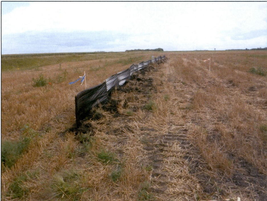
Figure 16. Outfall 007, silt fence installed at Station 224+00, looking south.
