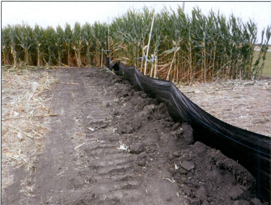
Figure 20. Outfall 009, silt fence installed at Station 289+00, looking southeast.
