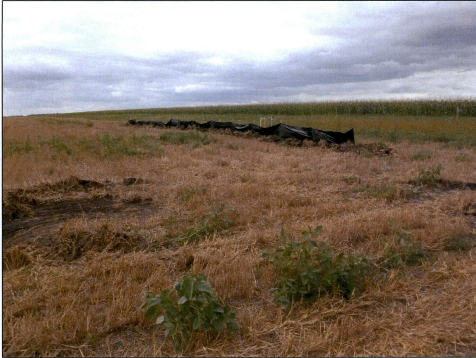
Figure 17. Outfall 007, silt fence installed at Station 224+00, looking northwest.
