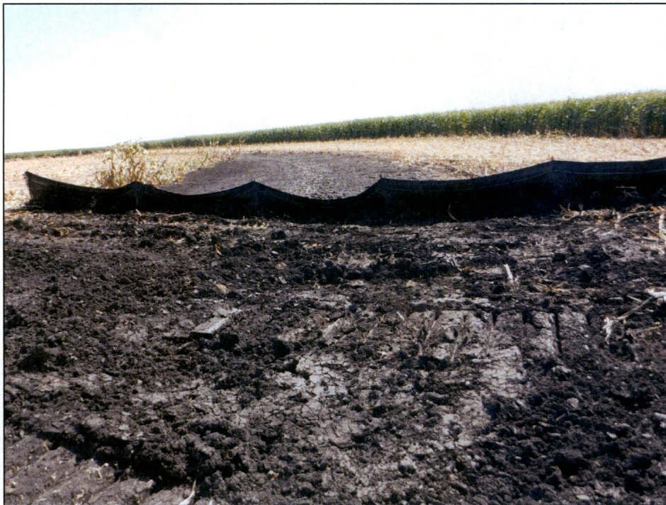
Figure 2. Outfall 001, silt fence on south side of Station 004+50, looking south.
