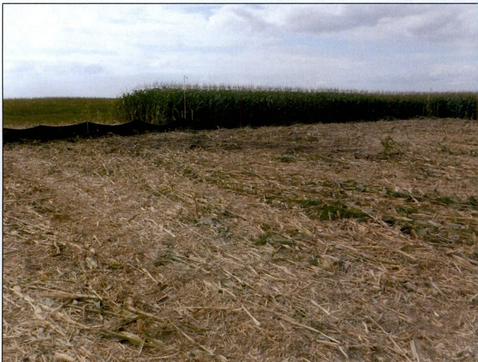
Figure 12. Outfall 006, silt fence installed on the east side of 165th Ave. SE, between Station 194+00 and Station 196+00, looking west.
