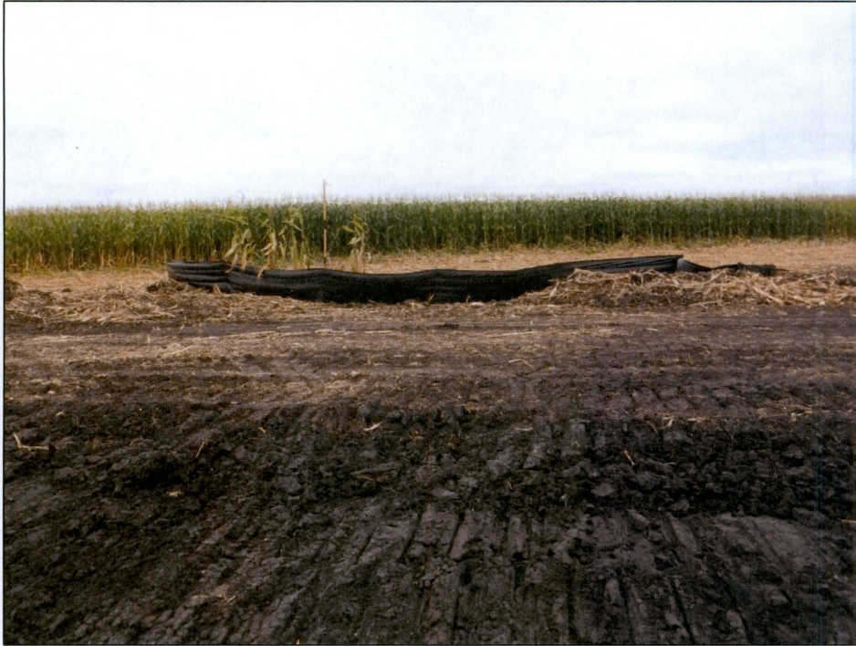
Figure 3. Outfall 001, silt fence on west side of ROW at Station 012+00.
