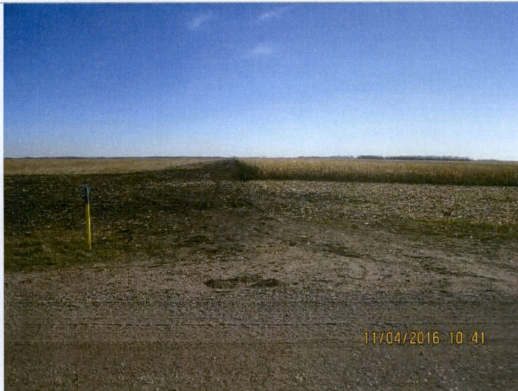
Photo 14: Alignment located at 165 th Ave SE crossing (looking east).
