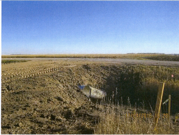
Photo 29: Approach along 165 th Ave SE.
