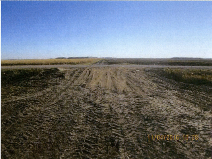
Photo 28: Approach along 165 th Ave SE.
