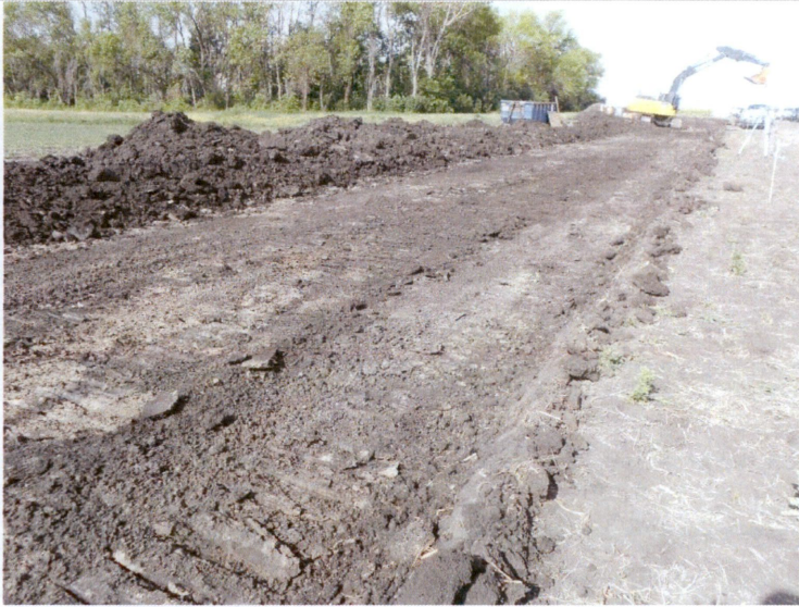
Photo 26: Topsoil separation.
