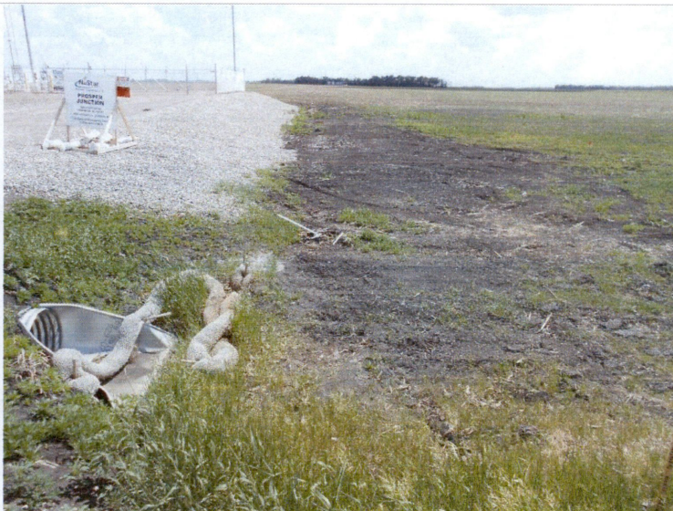
Photo 12/13: Pipeline corridor at Fargo Terminal at the intersection of 32 nd St SE and 166 th Avenue SE. Facing south. Erosion control features can be seen in the foreground near the newly installed culvert.
