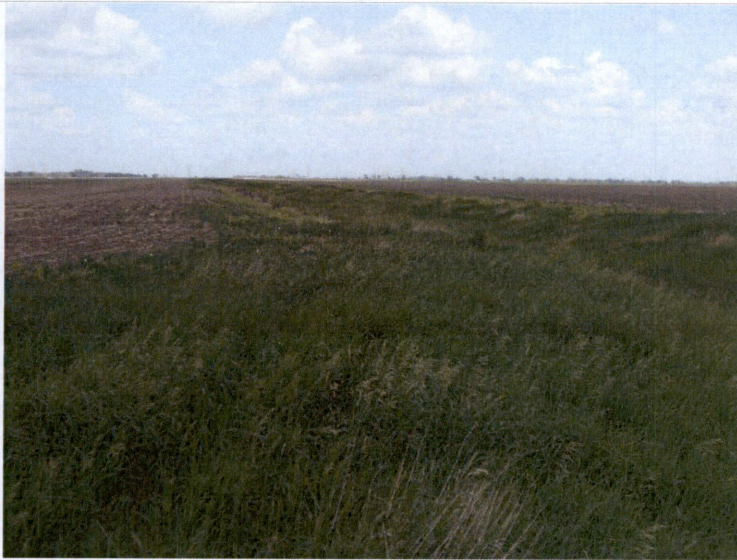
Photo 8/9: Pipeline corridor from County Road 20, facing northeast. Pipeline runs parallel to ditch on the left side of the photo.
