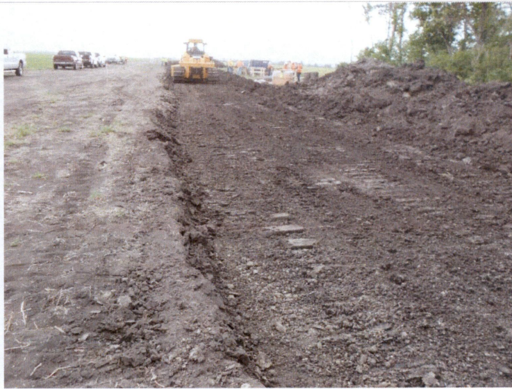
Photo 24: Topsoil separation.
