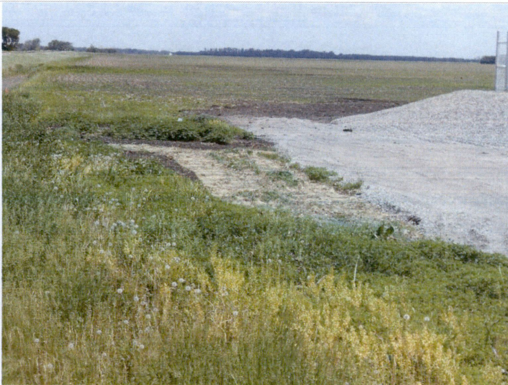
Photo 15: Fargo Terminal erosion control fiber mat erosion control.
