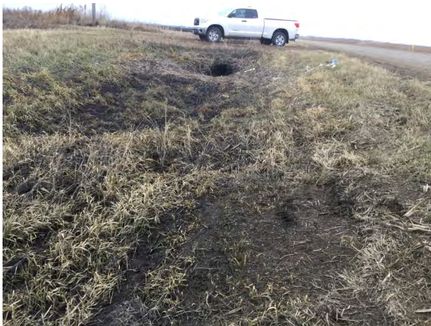
Photo 9: minor bare earth near intersection of 166 th Ave SE and 33 rd St SE (Section 15, T140N, R50W)
