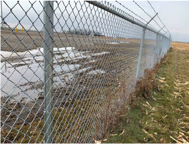
Photo 53: fence-line of new transmission facility, standing water, revegetation in progress (Section 4, T139N, R50W)
