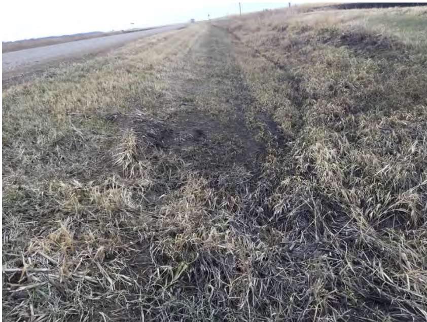
Photo 8: minor bare earth near intersection of 166 th Ave SE and 33 rd St SE (Section 15, T140N, R50W)
