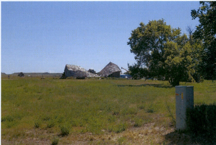
8) Dilapidated barn located 450 feet south of detector location. The barn could serve as potential roosting habitat for big or little brown bats. July 22, 2015. View south
