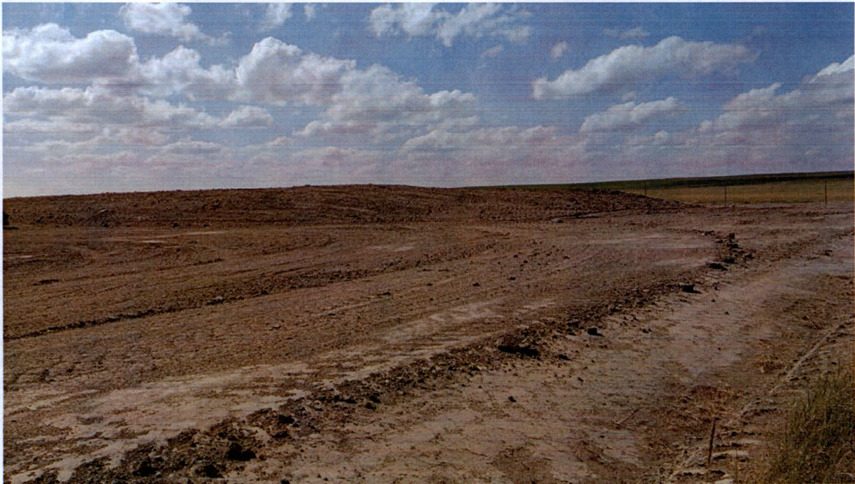
Report Photo #2 "Topsoil removal and north stockpile"
