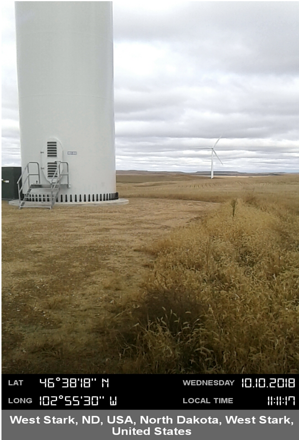
Report Photo #5: Overview of turbine construction block (T6) from South to North.
