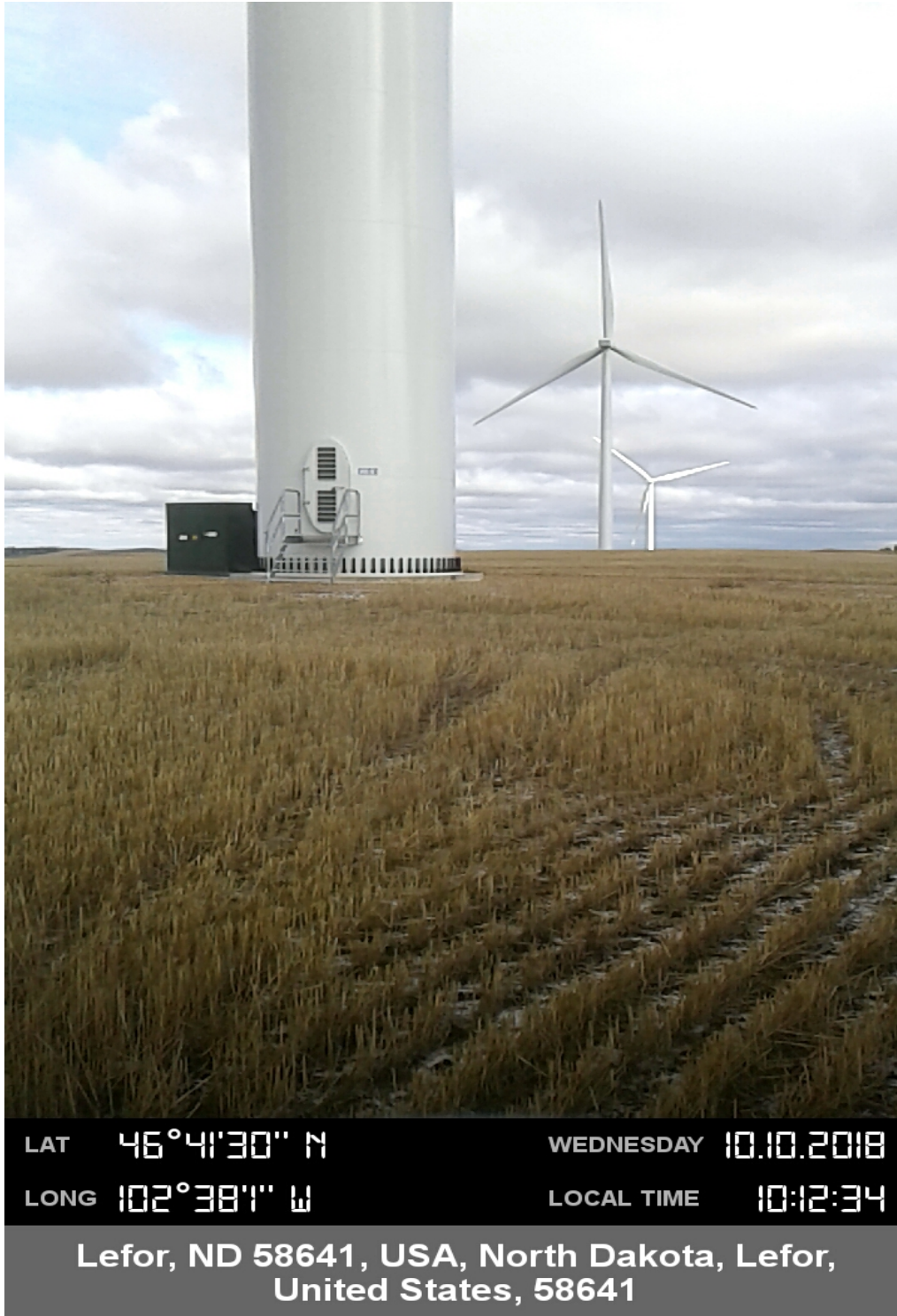
Report Photo #3: Overview of turbine construction block (T71) from South to North.
