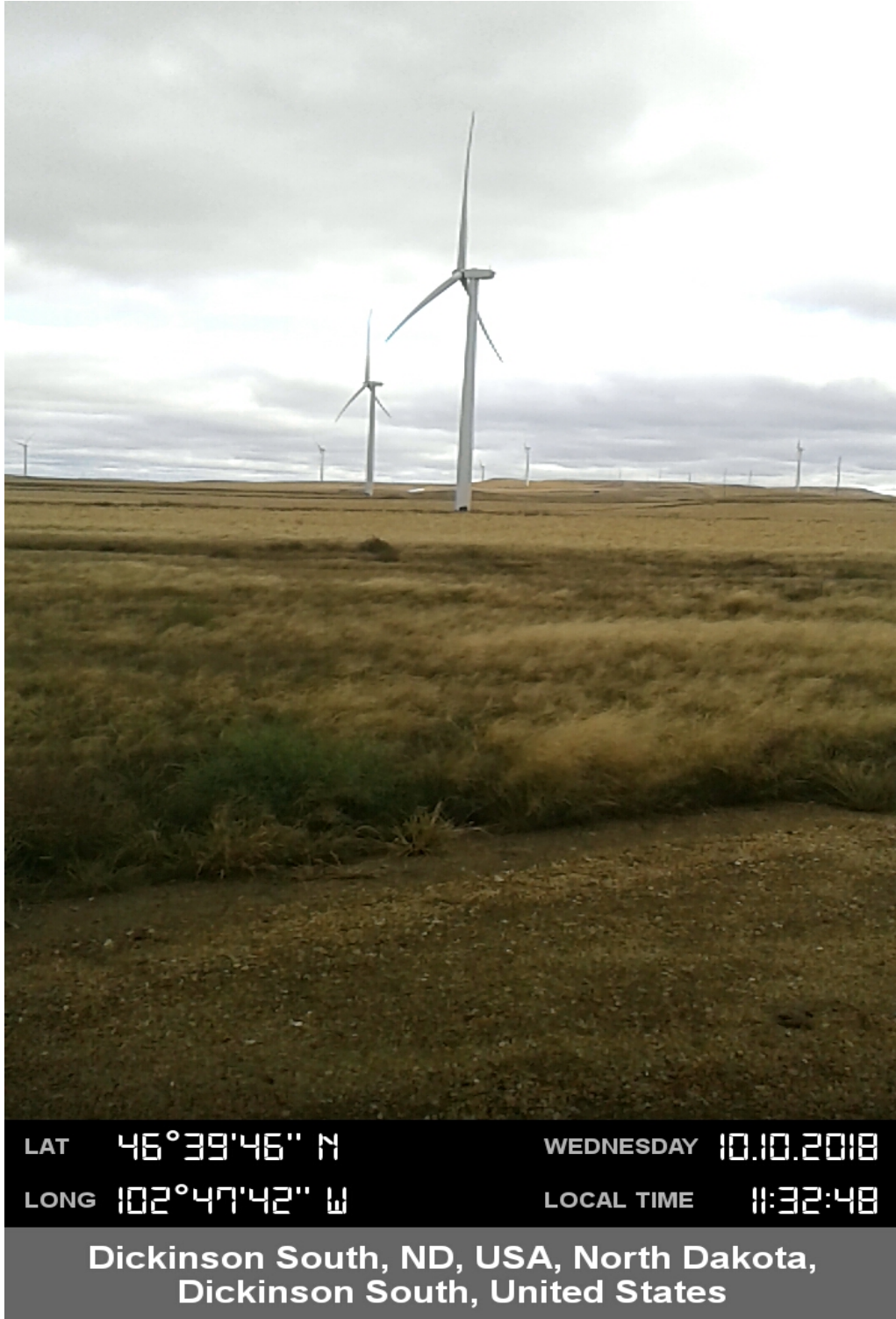
Report Photo #6: Overview of turbine array from T21 to T22. View from West to East.
