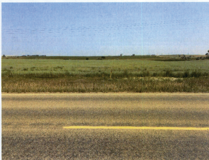
Photo No. 8 Tesoro Pipeline Station 46+00 to 42+89 Pipeline Bored under the Highway Looking East of ND Hwy 1806 July 31, 2017
