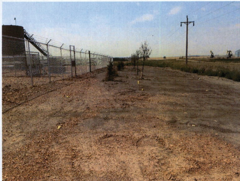
Photo No. 2 Tesoro Pipeline Station 0+57 to 2+00 PI #1 of Pipeline Project South of 40 th Street NW July 31, 2017
