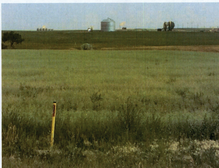
Photo No. 7 Tesoro Pipeline Station 9+69 to 42+89 Between PI #3 and PI #6 of Pipeline Project North of 40 th Street NW July 31, 2017
