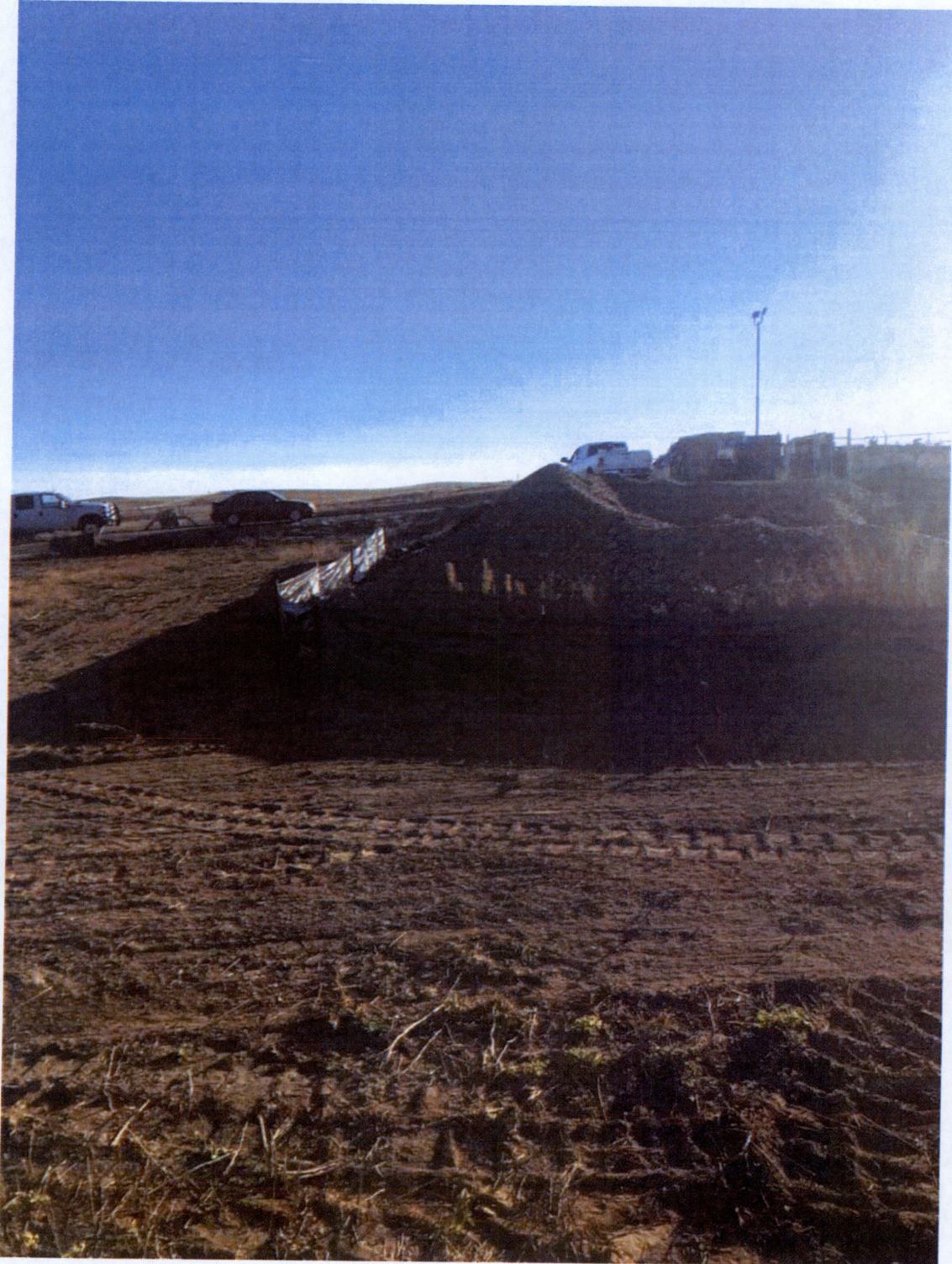
Photo 4 – BMP's added around spoils pile to help control stormwater runoff.
