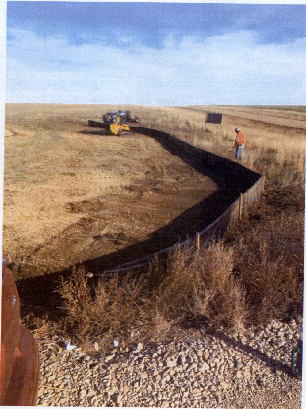
Photo 6 – New silt fence installation on East side facing North.
