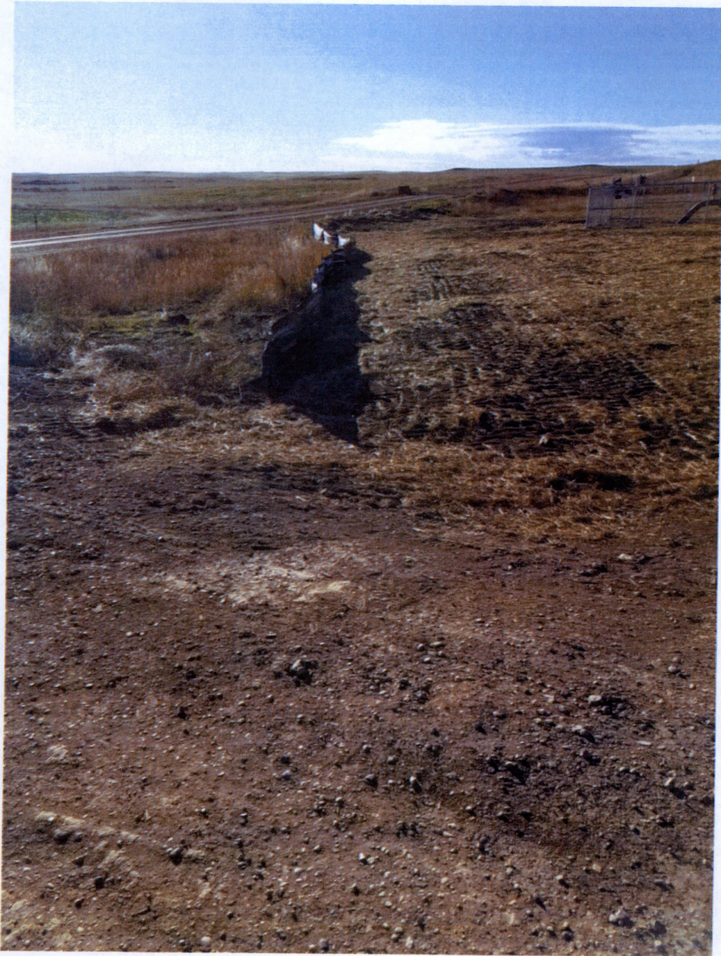
Photo 5 – East side entrance looking South.
