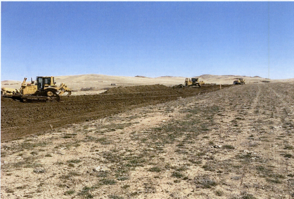
Photo 6 – Approx. Station 114+00. View of topsoil removal.
