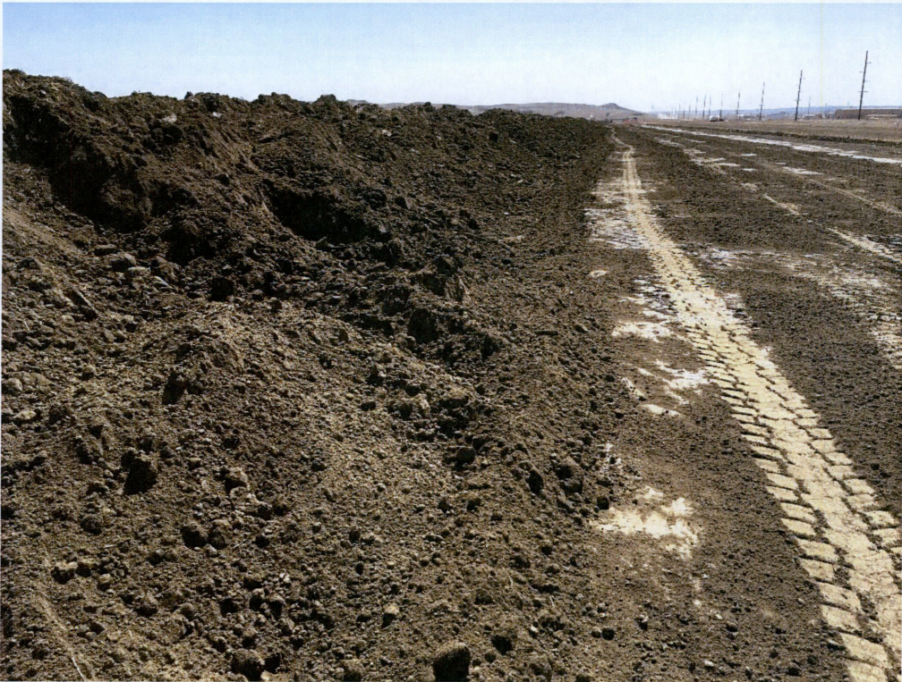
Photo 10 – Approx. Station 46+00. View of area after additional topsoil removal.
