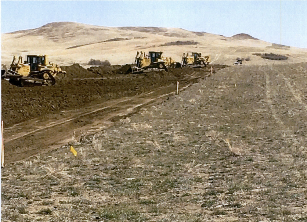
Photo 5 – Approx. Station 114+00. View of topsoil removal.
