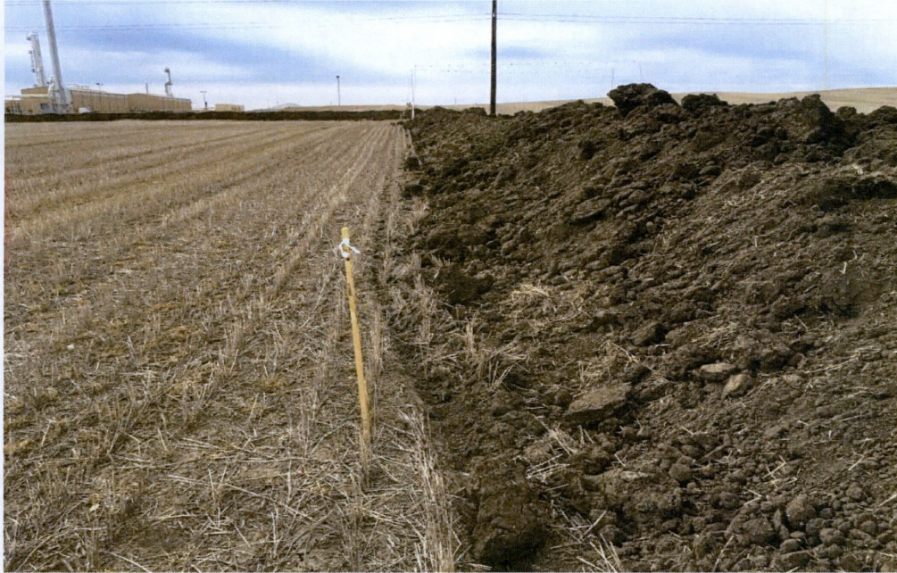
Photo 1 – Approx. Station 7+00. View of topsoil pile inside the boundaries of the approved corridor.
