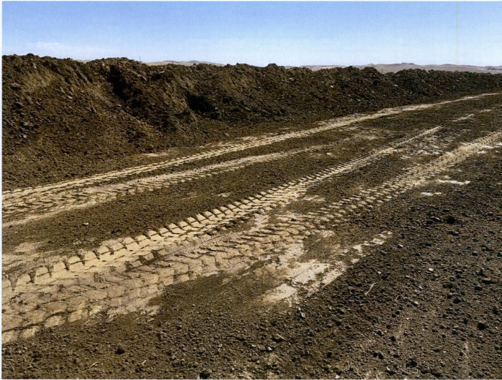
Photo 9 – Approx. Station 46+00. View of area after additional topsoil removal.
