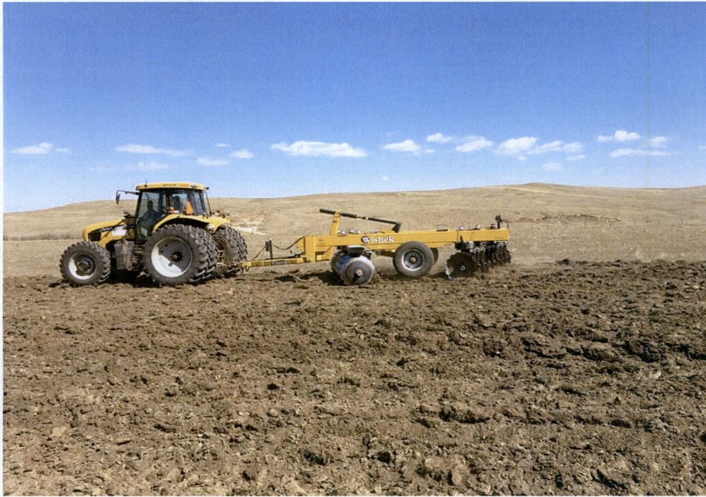
Photo 3 – Approx. Station 128+00. View of discing activities.
