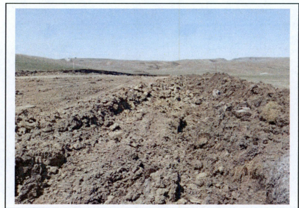
4. Spoil piles Sta#438+00 looking NW
