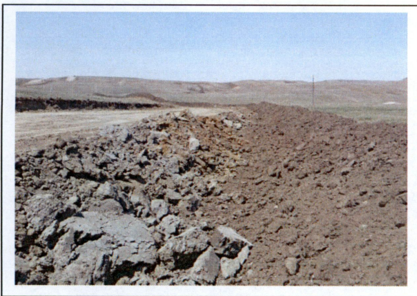
5. Spoil piles Sta#436+00 looking NW
