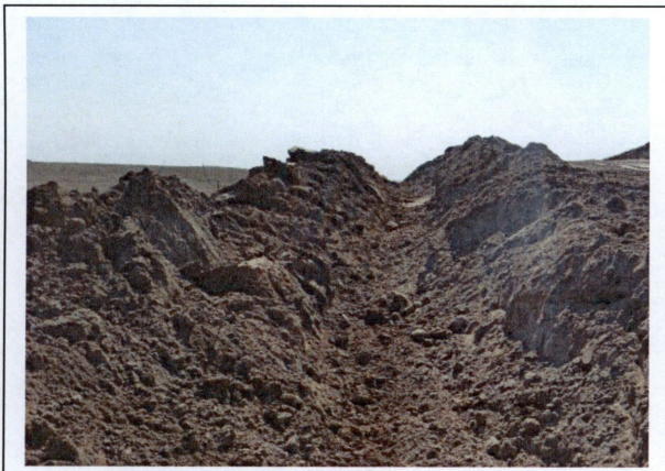
3. Spoil piles Sta#453+00 looking E
