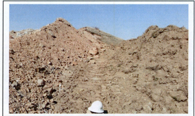
2. Spoil piles Sta#343+00 looking W
