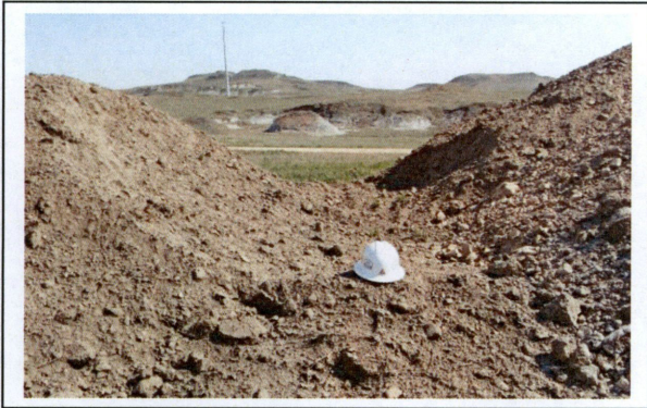
1. Spoil piles Sta#343+00 looking E
