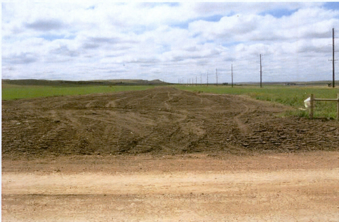
Photo 2 – Approx. Station 70+00. View of rough grade along the first 4 miles.
