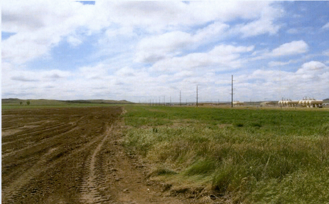
Photo 3 – Approx. Station 79+00. View of rough grade area with removed right of way stakes.
