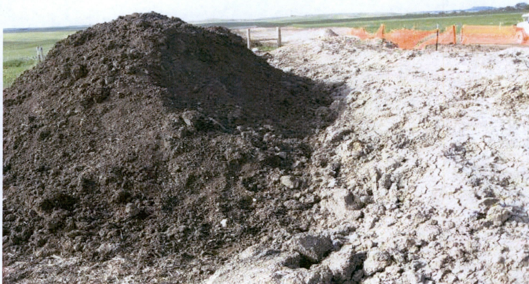
Photo 18 – Approx. Station 630+00. View of mixing topsoil and subsoil piles.
