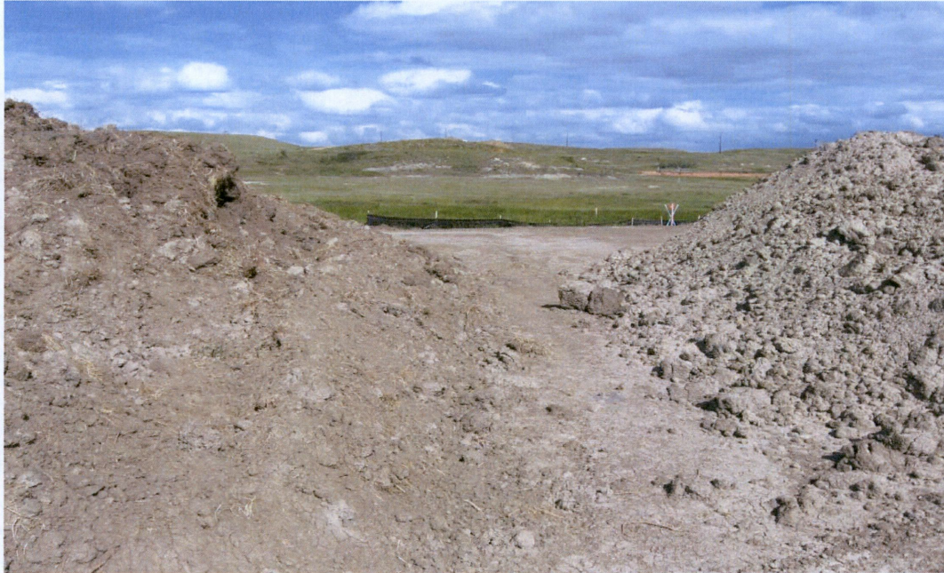
Photo 19 – Approx. Station 526+76. View of separated topsoil and subsoil piles.
