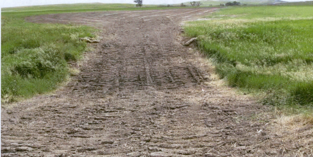
Photo 7 – Approx. Station 93+00. View of slope and wetland; inspector recommended erosion control.
