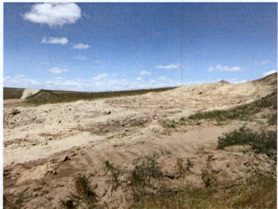
View W; St. 210; subsoil rough-graded, topsoil spoils piles remain segregated
