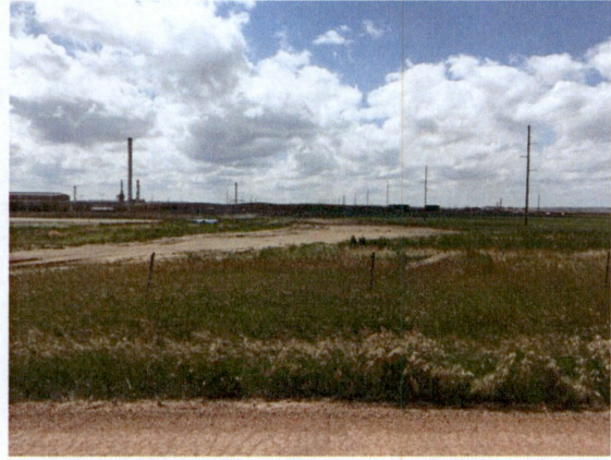
View W; St. 40; topsoil replaced, rough-graded on ROW
