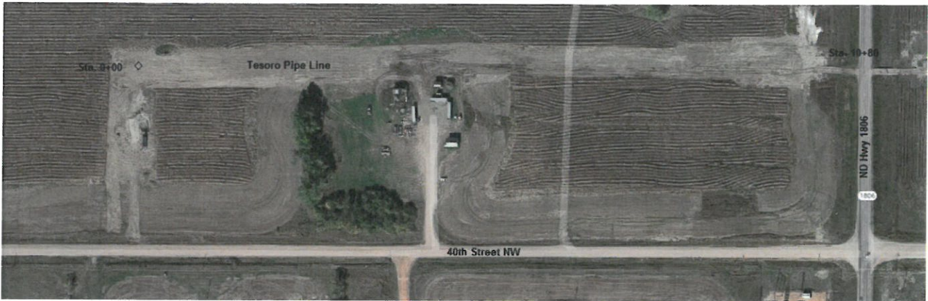
Station 0+00 to 10+80 Aerial Photo #1 Top Soil placed over the Tesoro Pipe Line Trench West of Highway 1806 September 2016
