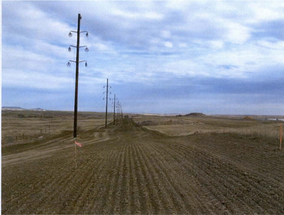
Photo 11 – Approx. Station 894+00. View of restoration, adjacent power line, and stakes for an unrelated project.
