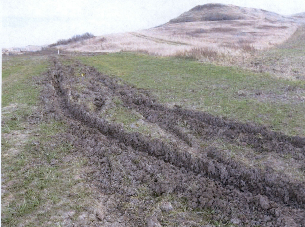
Photo 12 – Approx. Station 921+00. View of rutting in the right of way.
