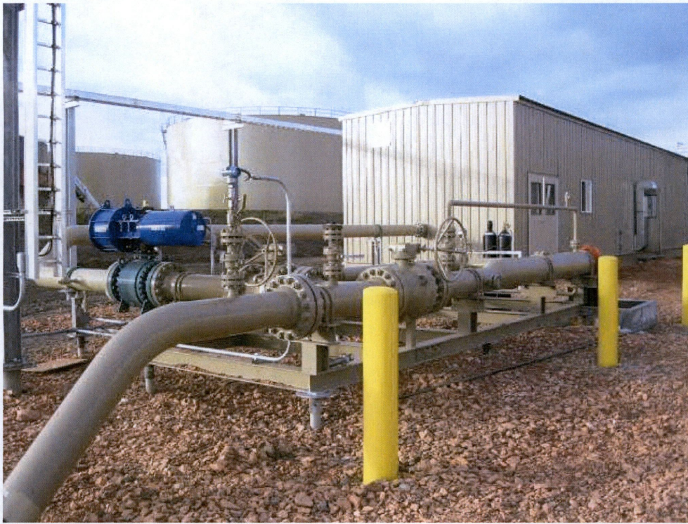
Photo 1 – Approx. Station 0+00. View of interconnect with pump house.
