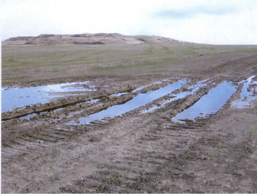
Photo 9 – Approx. Station 753+00. View of minor rutting in right of way.
