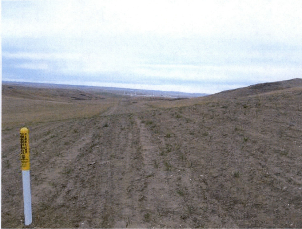
Photo 5 – Approx. Station 140+00. View of restoration.
