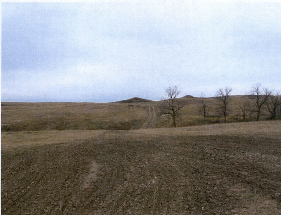
Photo 6 – Approx. Station 228+00. View of restored HDD workspace.
