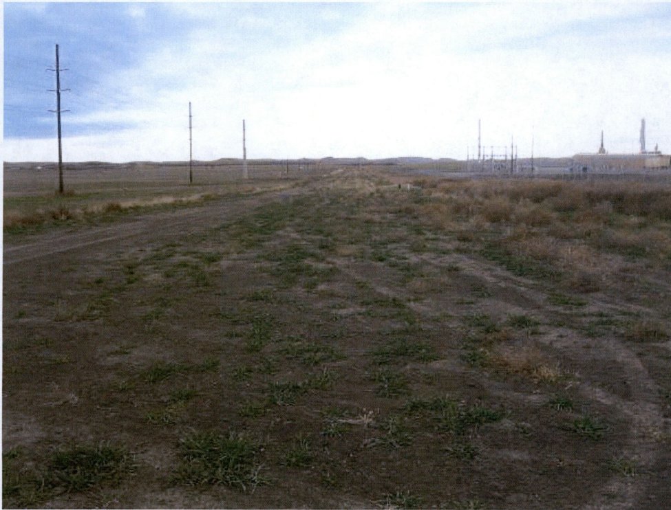
Photo 2 – Approx. Station 17+00. View of restored right of way and revegetation.
