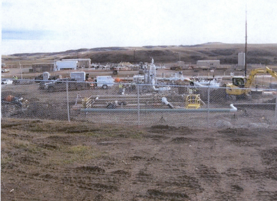
Photo 14 – Approx. Station 983+00. View of the interconnect valve site.
