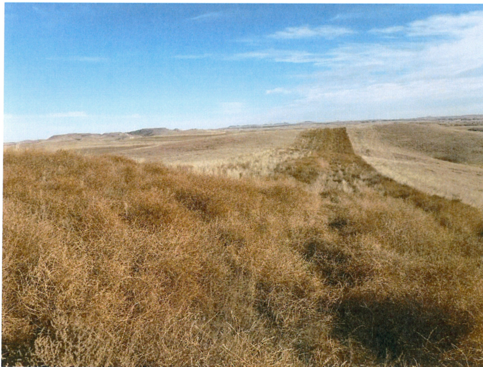
Photo 20 – Approx. Station 267+00. View of the right of way showing successful revegetation.
