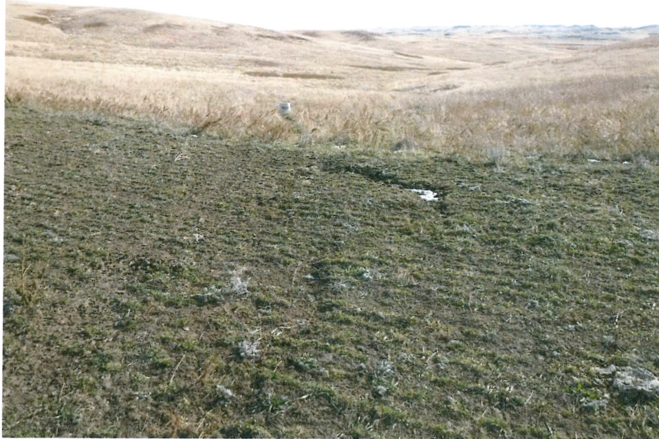
Photo 19 – Approx. Station 261+00. View of minor erosion.
