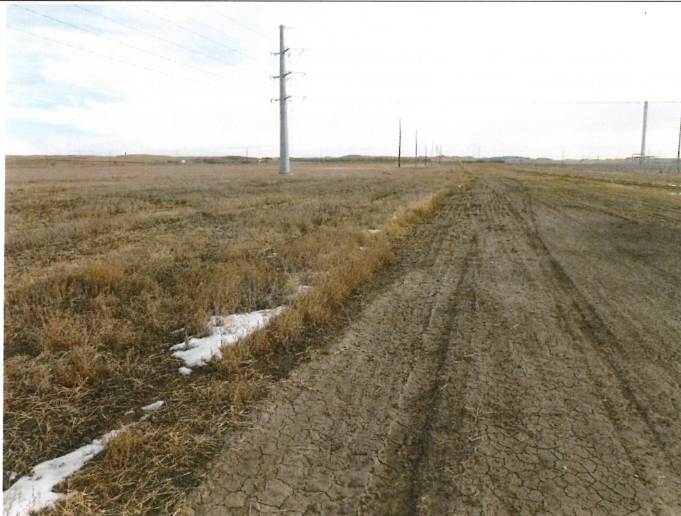
Photo 6 – Approx. Station 38+00. View of right of way requiring additional seeding.
