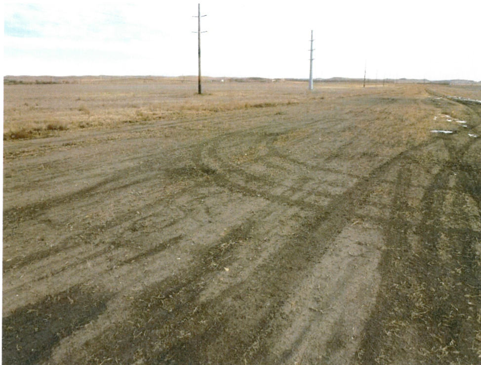
Photo 5 – Approx. Station 30+00. View of right of way requiring additional seeding.
