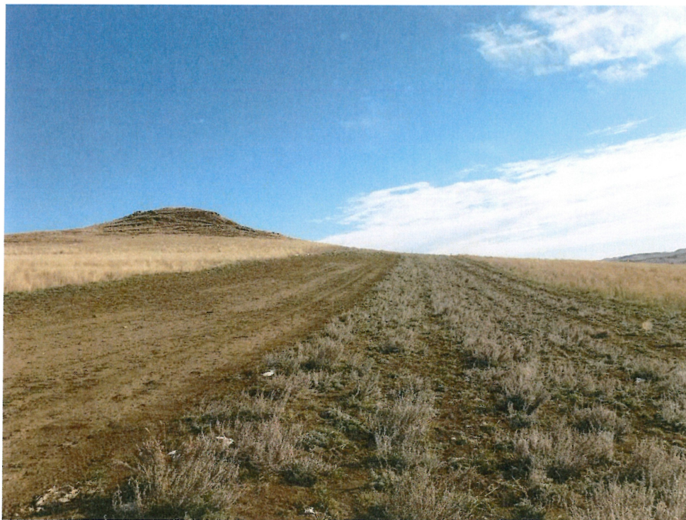
Photo 16— Approx. Station 200+00. View of half right of way revegetation, half requires seed.
