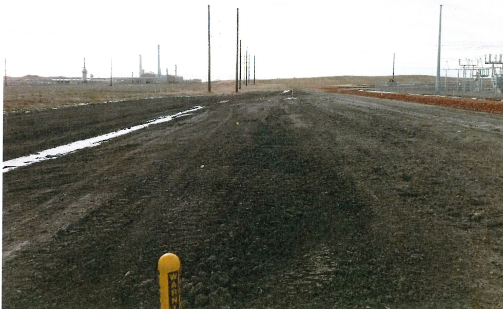
Photo 2 – Approx. Station 6+00. View of portion of right of way requiring additional seeding.
