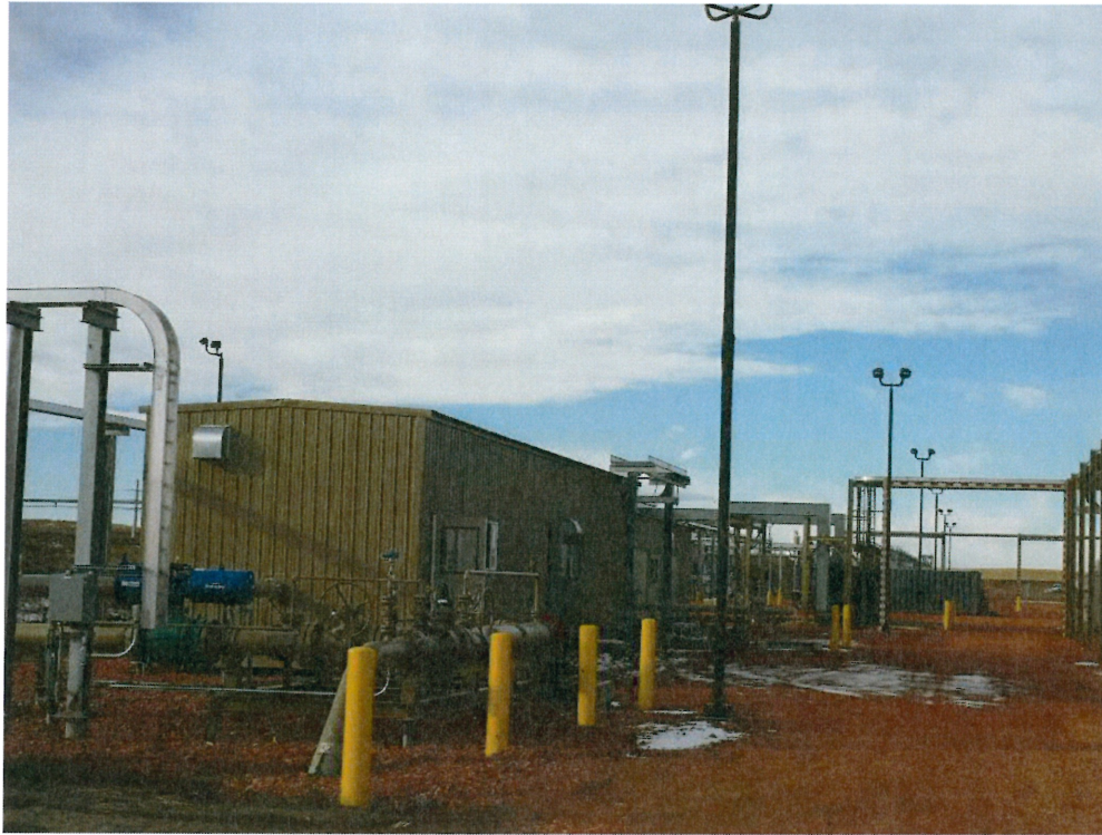
Photo 1 – Approx. Station 0+00. View of interconnect with pump house.
