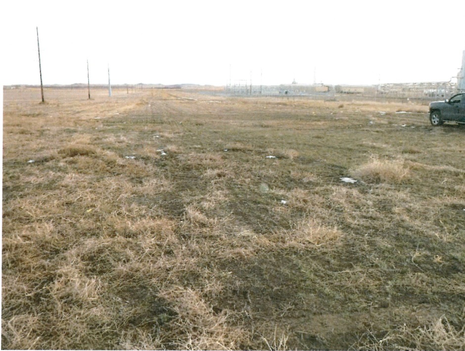
Photo 3 – Approx. Station 15+00. View of right of way requiring additional seeding.
