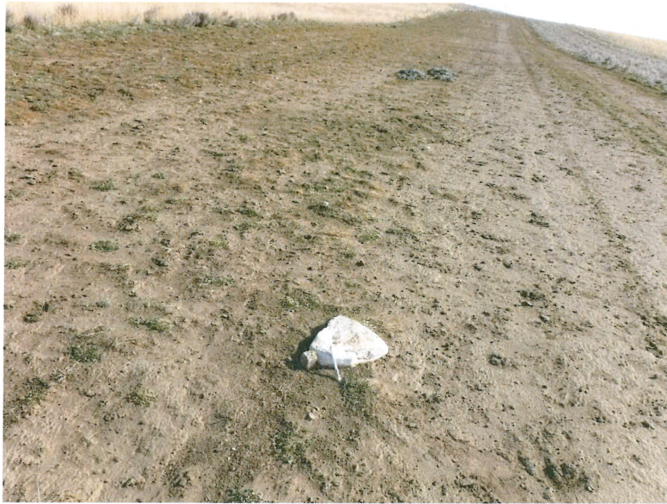
Photo 15— Approx. Station 190+00. View of rock to be removed from the right of way.
