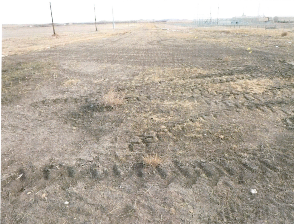
Photo 4 – Approx. Station 21+00. View of right of way requiring additional seeding.
