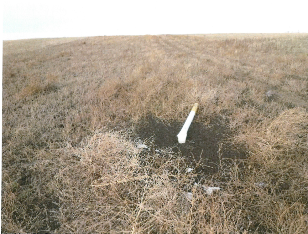
Photo 24 – Approx. Station 611+00. View of pipeline marker needing repair.
