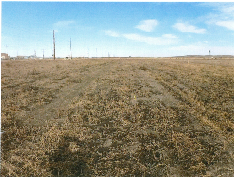
Photo 8 – Approx. Station 75+00. View of right of way requiring additional seeding
