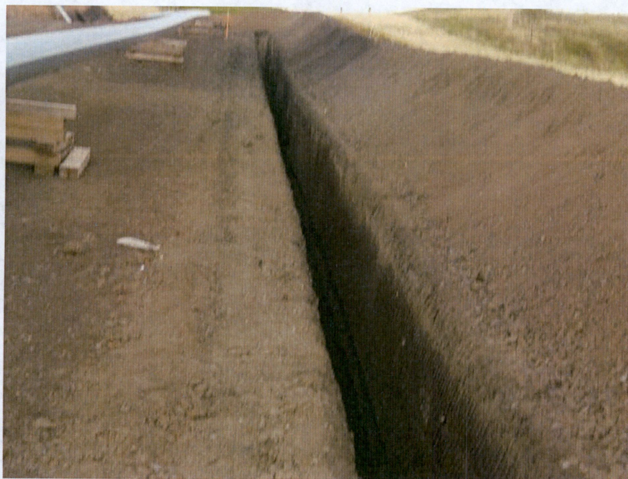
Photo 14: Located at station 146+00, showing Right of Way direction looking west with Right of Way graded. Right of Way has been trenched with subsoil located on right side of trench. Topsoil is pushed off Right of Way located on left side of photo not shown. Pipe is welded, sitting on skids ready to place in trench.
