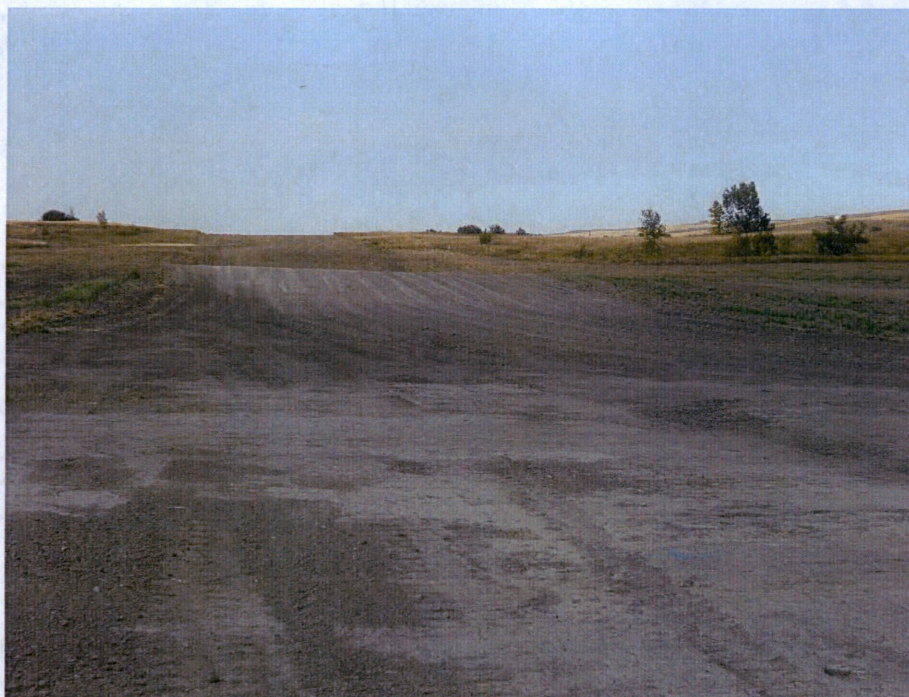
Photo 3: Located at station 213+00, showing graded Right of Way headed north.
