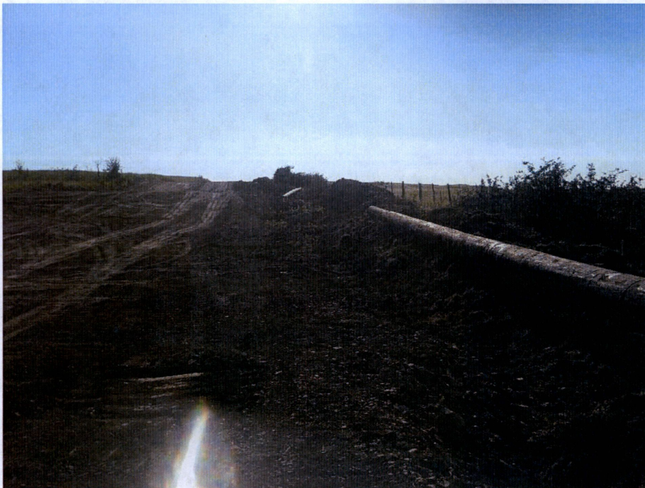
Photo 8: Located at station 93+00, showing Right of Way direction looking east with graded topsoil pushed to edge of Right of Way. Power pole is shown laying on topsoil located on right side of photo.
