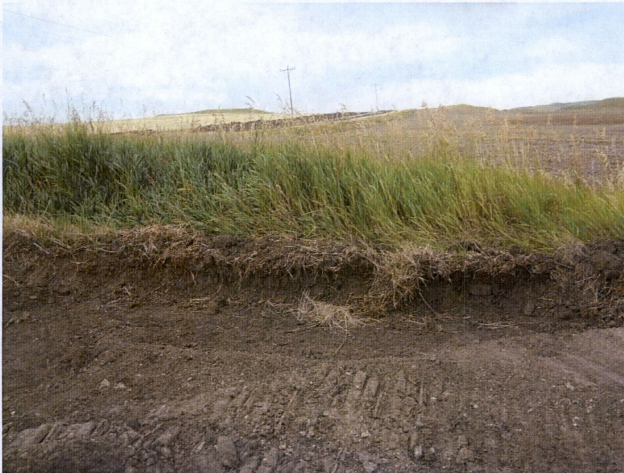
Photo 10: Located at station 132+00, photo showing stripped Right of Way at approximate topsoil depth of 12 inches. Photo is showing west side of Right of Way.
