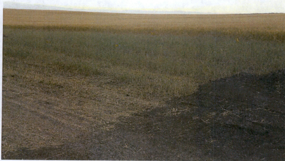
Photo 13: Located at station 146+00. Photo showing flagged location of existing Hess lines which is approximately 700 ft. east of actual Hess line location hit during trench excavation.
