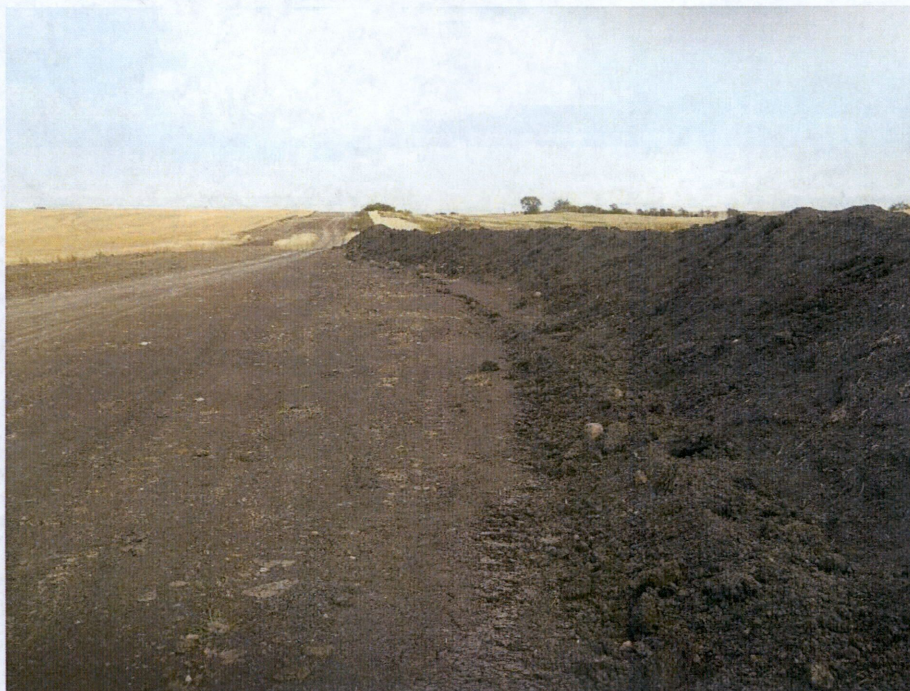
Photo 6: Located at station 240+00, showing graded Right of Way direction looking north. Topsoil is pushed off and placed in edge of Right of Way on the west side.
