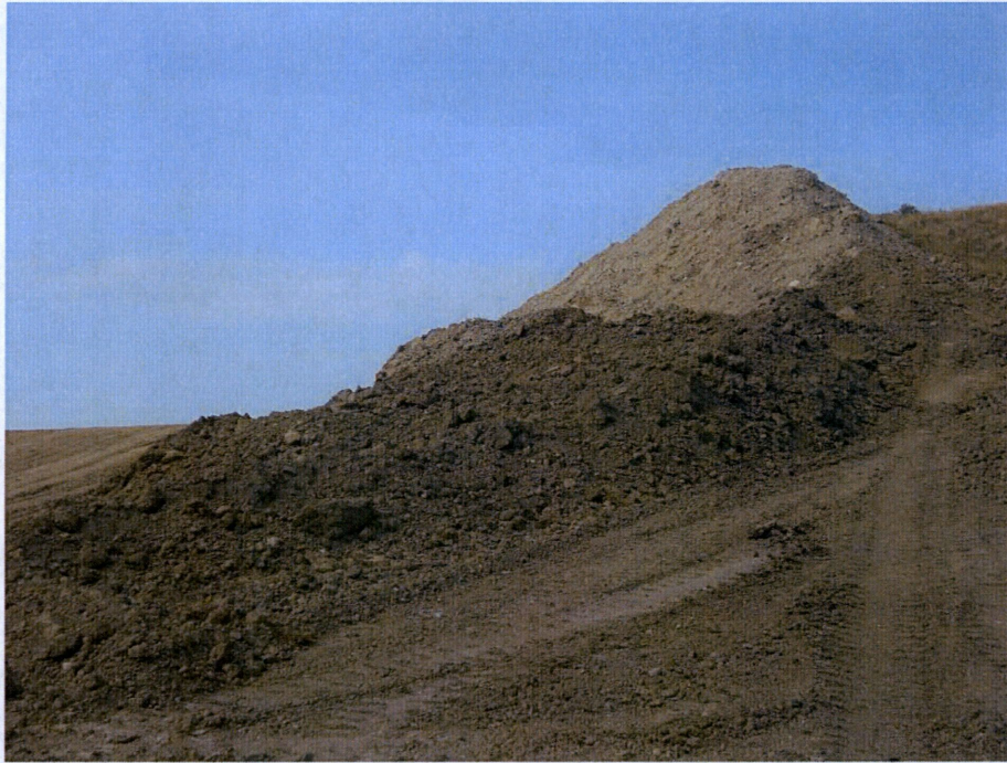
Photo 19: Located at station 459+00, showing topsoil placed along edge of Right of Way. Topsoil needs to be regraded and levelled over Right of Way to original condition.
