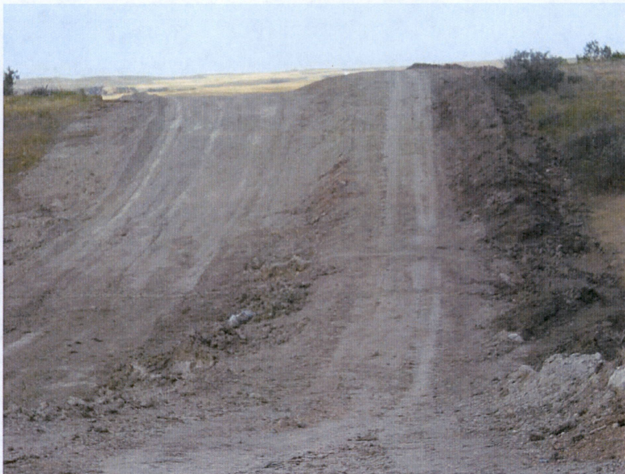
Photo 26: Located at station 510+00, looking north of Right of Way, showing piping installed in trench and backfilled. Topsoil shown on right side along Right of Way. Grading work has not been started yet.
