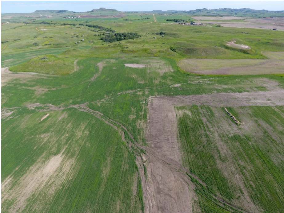
Location 9, Looking North (47.819866, -102.877708) Scar visible from recent/adjacent work on a different pipeline
