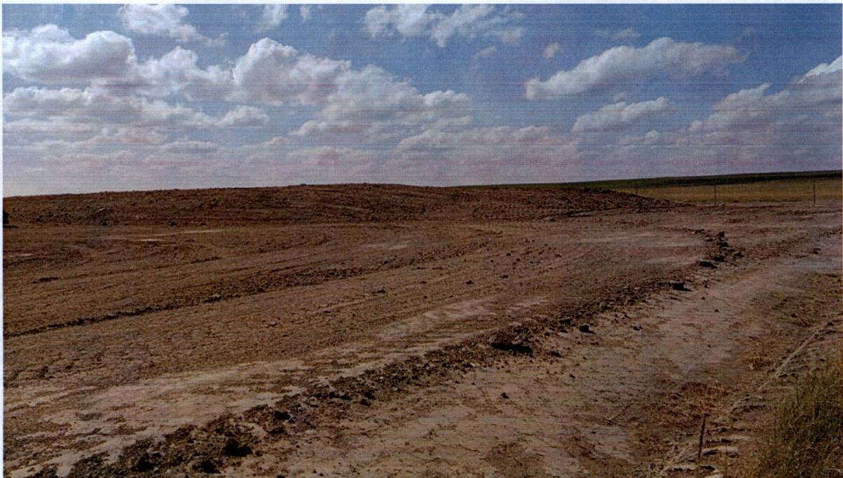
Report Photo #2 "Topsoil removal and north stockpile"
