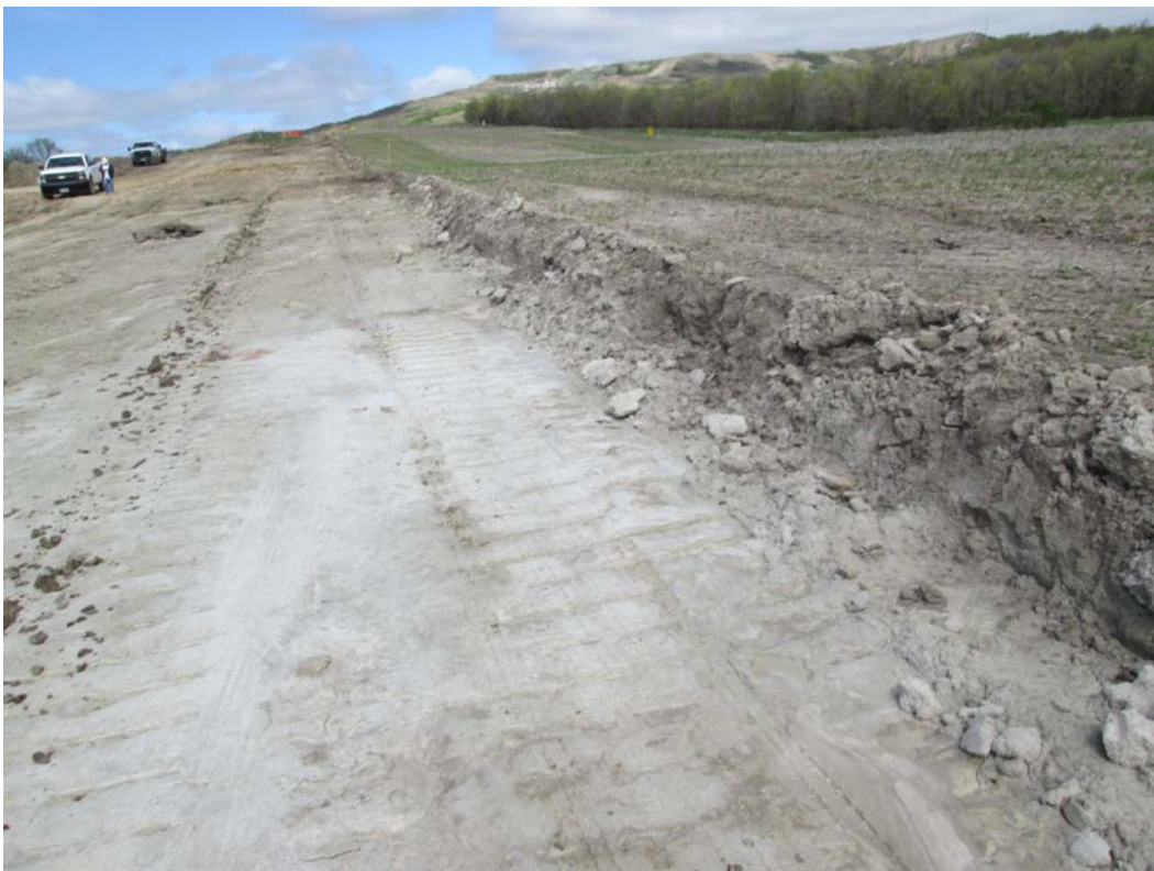
Below: Photo 6 (pt. 273) – Direction looking north. Topsoil stripped; small zone of light, white coloring on soil, appeared calcareous.
