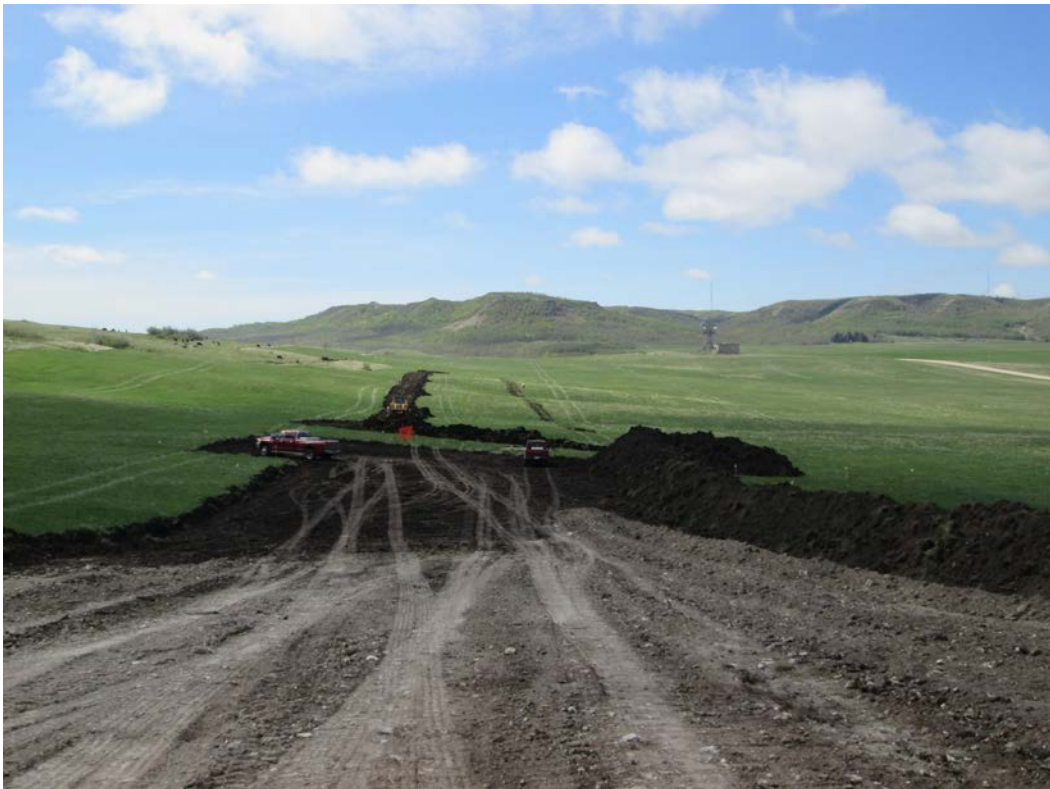
Below: Photo 8 (pt. 275) – Direction looking south. View on top of two-tone area, pushed some subsoil downhill, angled down to level out area after 12-in topsoil was taken. Extended ROW for bore location, boring under other line. Dozer stripping topsoil.
