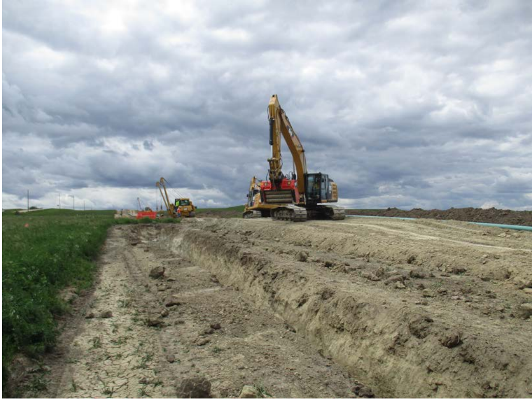
Above: Photo 21 (pt. 442) – Direction looking west. Subsoil pile from trench is flattened for work area.
