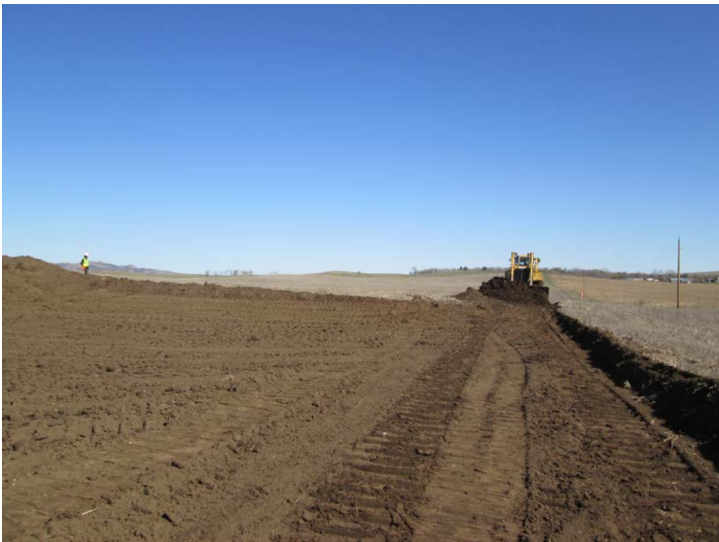
Below: Photo 2 (Point 267) – Direction looking north. Start of topsoil stripping.
