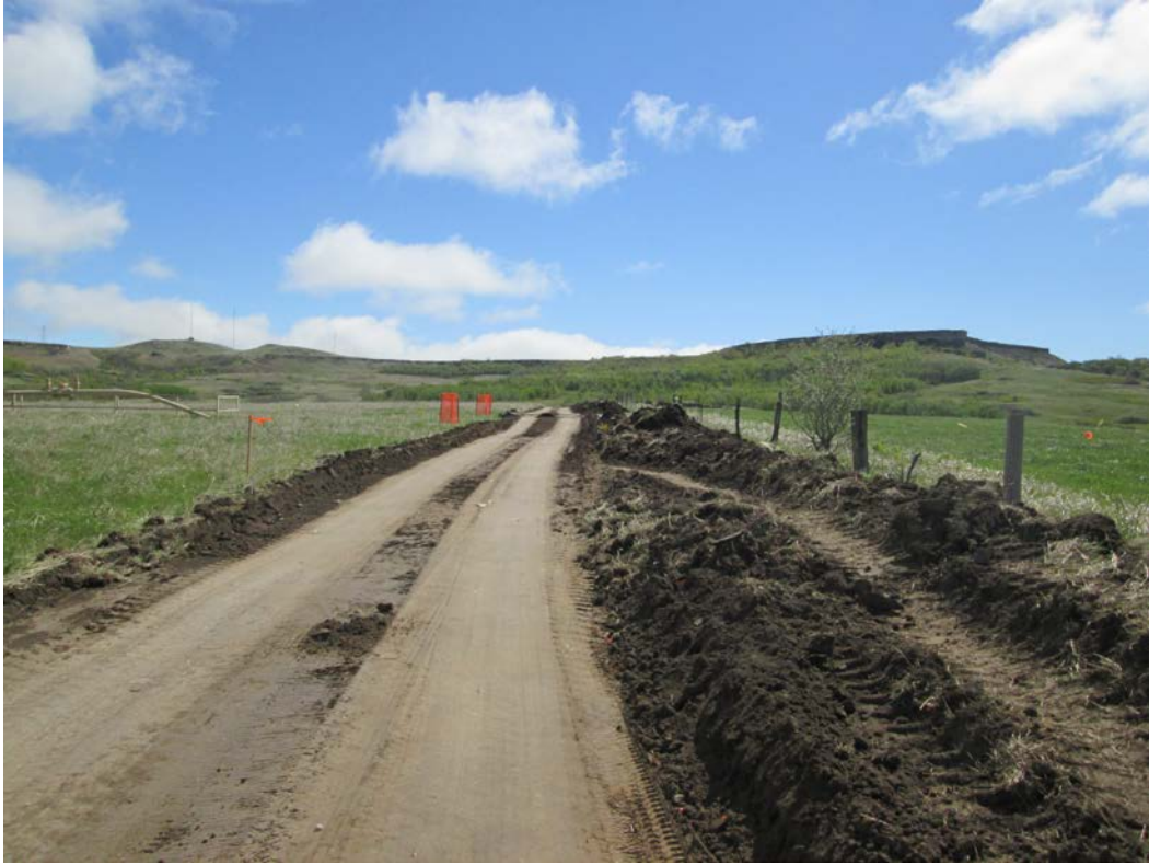
Above: Photo 7 (pt. 274) – Direction looking east. Topsoil stripped for access road.
