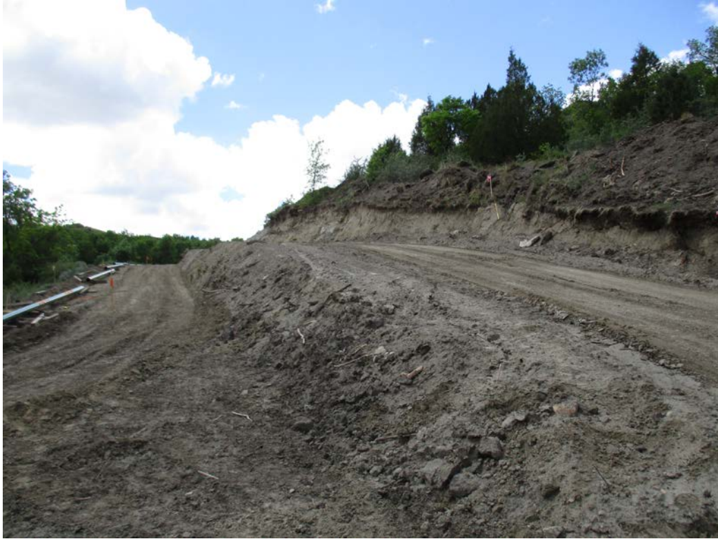
Above: Photo 19 (pt. 441) – Steep slope, with little topsoil. Two-tone area. Topsoil to the far right of photo.
