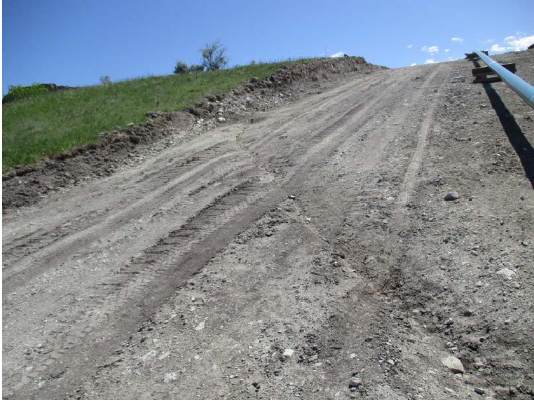
Above: Photo 13 (pt. 435) – Slope breaker on ROW.
