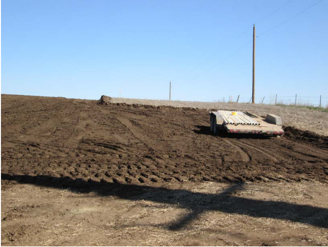
Above: Photo 3 (pt. 267) - Direction looking north. Extended ROW to 125-ft for additional work space for road bore.
