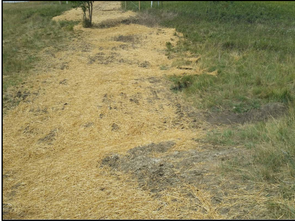
Photo 17. (GPS Point #459) – Gully forming in drainage area. No erosion control device was in place but it was stated by H2 Enterprises that an erosion control device will be placed here.
