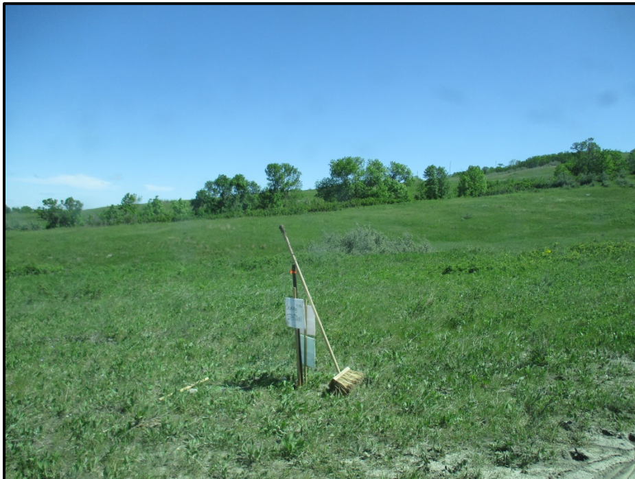
Photo 4. – Cleaning station set up near edge of ROW. This could be used when going into environmentally sensitive areas, etc., to prevent spread of weeds.
