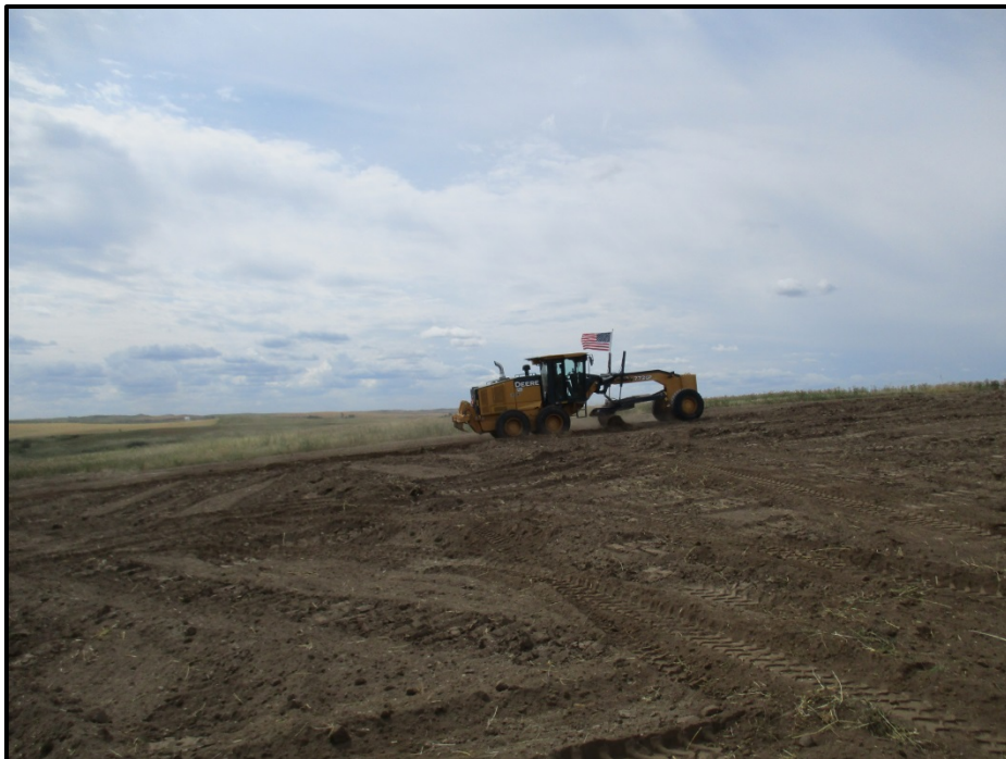
Photo 14. (GPS Point #457) – Motor grader shown smoothing out ROW.
