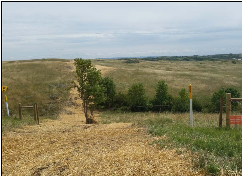
Photo 18. (GPS Point #459) – Pipeline ROW, drainage area and road bored. Bore pit was at the top of the hill, area in between was driven on to access bore area. Note signs and pipeline markers along fence line with fence gate. Direction: Southeast.
