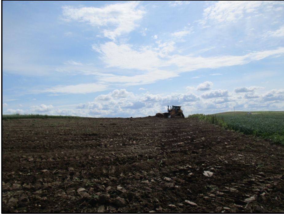
Photo 15. (GPS Point #456) – Dozer spreading topsoil out on the ROW.
