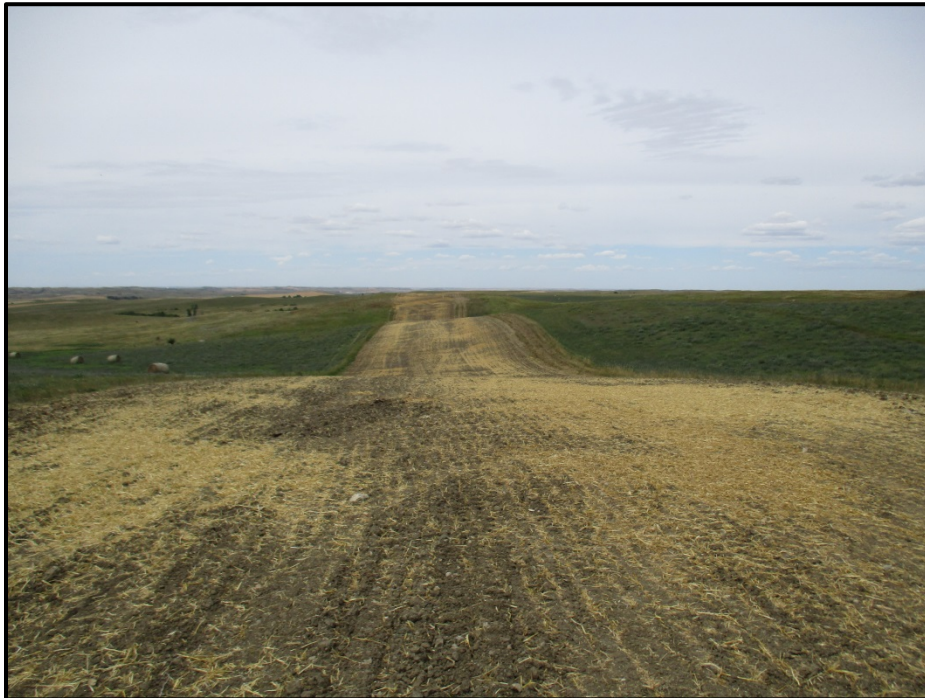
Photo 16. (GPS Point #458) – Pipeline ROW, reclamation done by local contractor (not H2 Enterprises). ONEOK/H2 Enterprises stated that they thought it had been re-seeded (a second seeding) the week before. Direction: Northwest.
