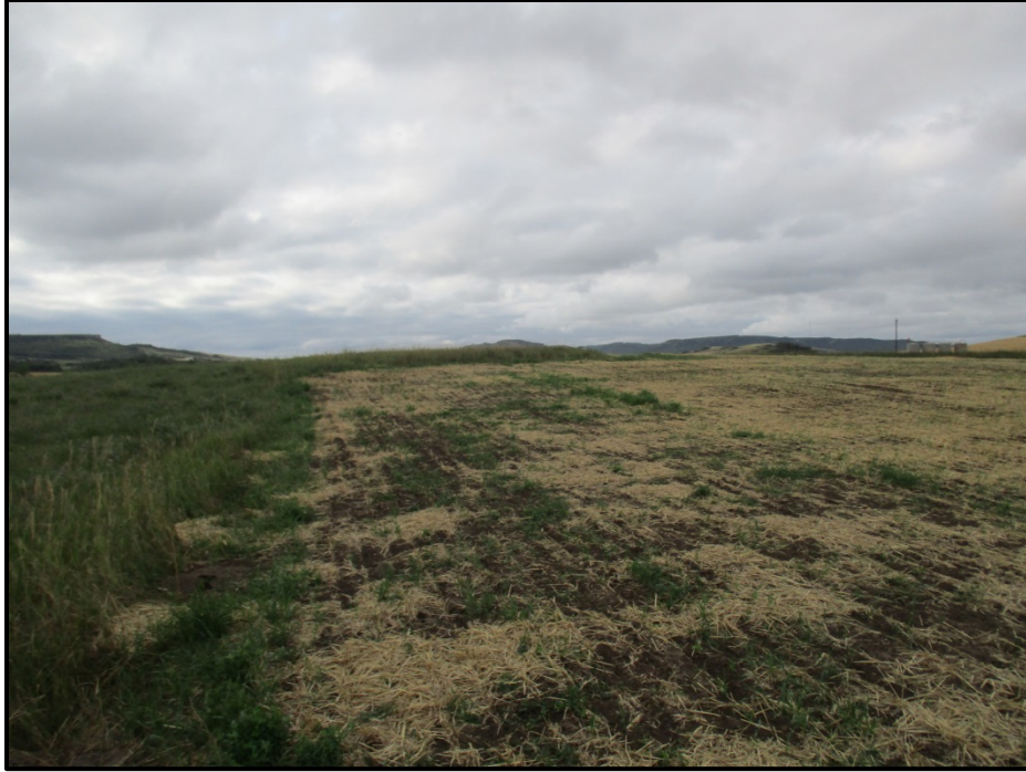
Photo 7. (GPS Point #451) - Topsoil had been replaced back on the ROW. Straw mulch was laid down with seeding. Some vegetation had already started to grow.
