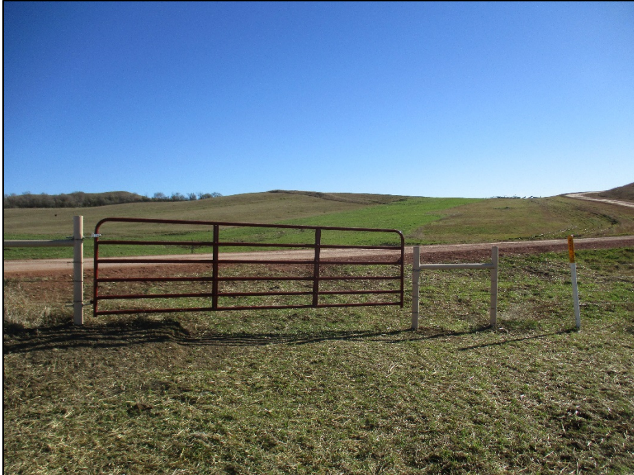
Photo 12. (GPS Point #502) – Pipeline ROW with fence gate and pipeline marker. Area was seeded and mulched. Grasses are growing. Direction: East.
