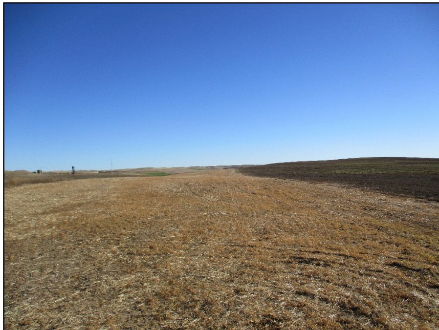
Photo 22. (GPS Point #506) – Pipeline ROW through field. Area mulched and seeded. The area did have grasses growing previously. It appears that it was potentially sprayed, or when the adjacent field was sprayed the wind carried the herbicide over to this area. Direction: Southeast.
