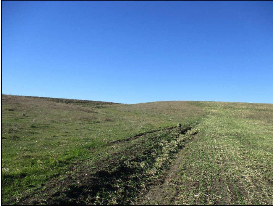
Photo 5. (GPS Point #498) –Grasses starting to grow within the pipeline ROW. The waterbar (shown to the left center of photo) helps divert or slow water from the drainage area away from the pipeline ROW. Direction: West.
