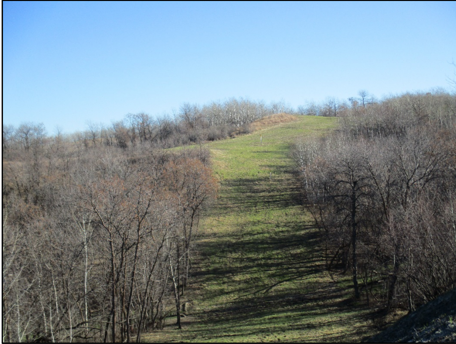
Photo 7. (GPS Point #499) – Ravine area, with pipeline markers. Trees and shrubs were removed. Direction: East.
