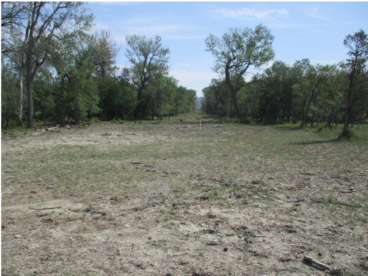
Photo 8. (Point 541) Facing: East. View across the cut of the ROW through the wooded floodplain toward the Little Missouri River (the route was bored but woody vegetation was cut to ground level within permanent ROW). The foreground shows the reclaimed workspace for the bores to the west and east from this point. The planted species were coming in across the area but cover was fairly low at 10-25%; species observed were western wheatgrass, slender wheatgrass, and green needlegrass. Yellow sweetclover and prostrate vervain ( Verbena bracteata ) were common. Bare ground was over 75%. In the cut area between woodland, native shrubs were growing back from cut stems and native woodland sedges (likely Carex sprengei ) and wood violet were growing back. The noxious weed Canada thistle ( Cirsium arvense ) was scattered in this area; it was common in the adjacent woodland.
