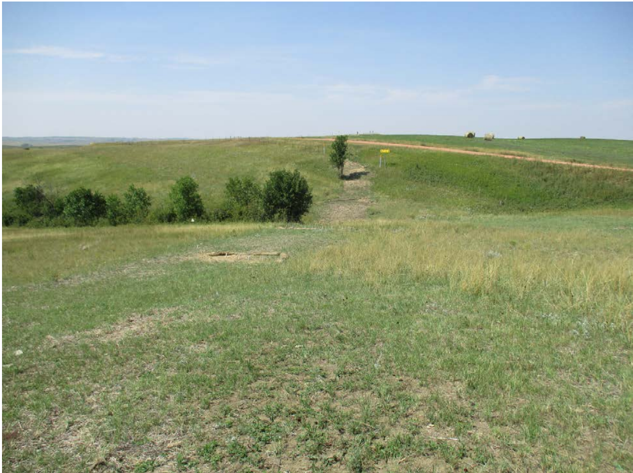
Photo 10. (Point 545) Facing: Northwest. View of an upland drainage crossing. This particular drainage had several spots of bare ground, but overall the planted grasses were coming in, erosion control was in place, and drainage flows had been reestablished.
