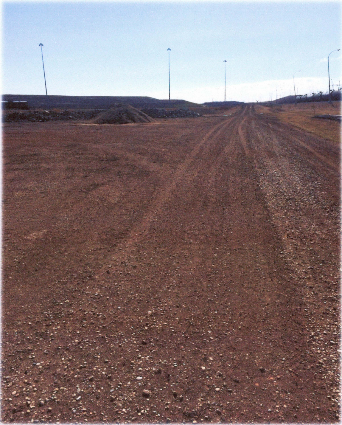
Figure 7: Overview of the survey corridor running along the southern edge of the Plant showing the work space (at left) and Northern Pacific Rail Road (at right). Photo taken from the center of the APE, view to the Southeast.
