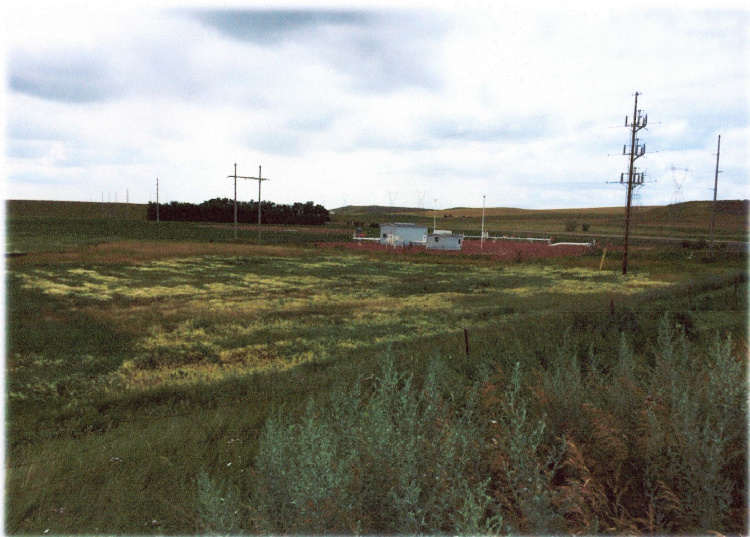
Figure 10: Overview of hay field and the meter station at the southern end of the survey corridor. Photo taken from the center of the APE, view to the southeast.
