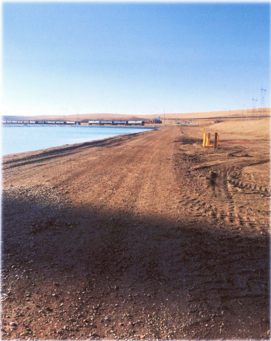
Figure 4: Overview showing the evaporation pond, existing pipeline, monitoring wells, and large berm which all intrude into the right-of-way. Photo taken from the center of the APE, view to the South.
