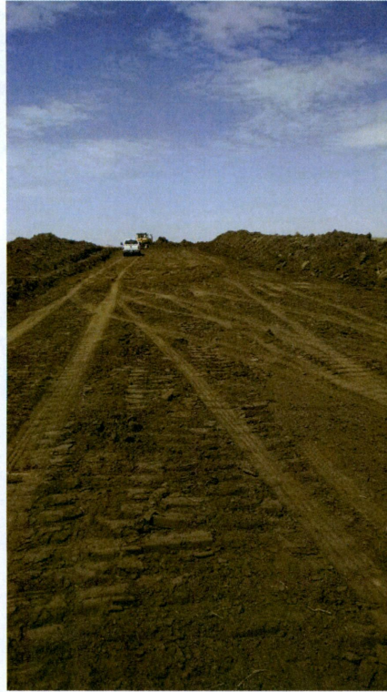
Photo 24: Station 1726+75, looking North at right-of-way being stripped and topsoil pile right
