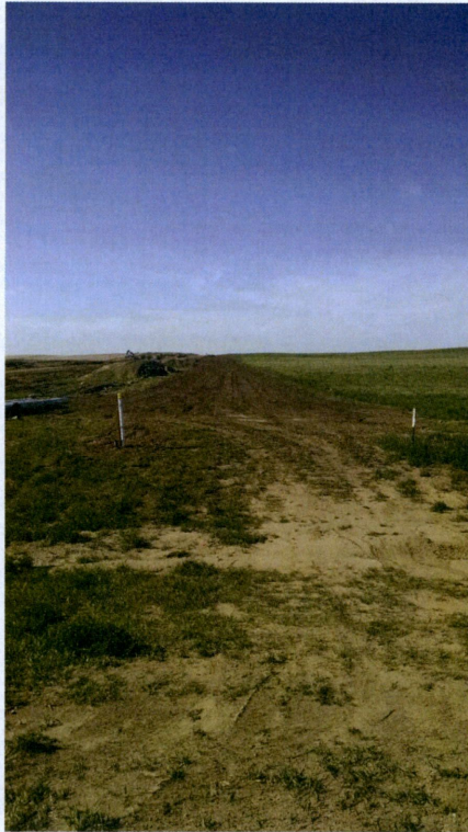
Photo 115: At 34th Street, looking North at completed right-of-way
