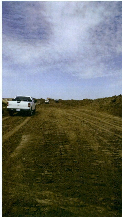
Photo 20: Station 1730+75, looking North at right-of-way being stripped
