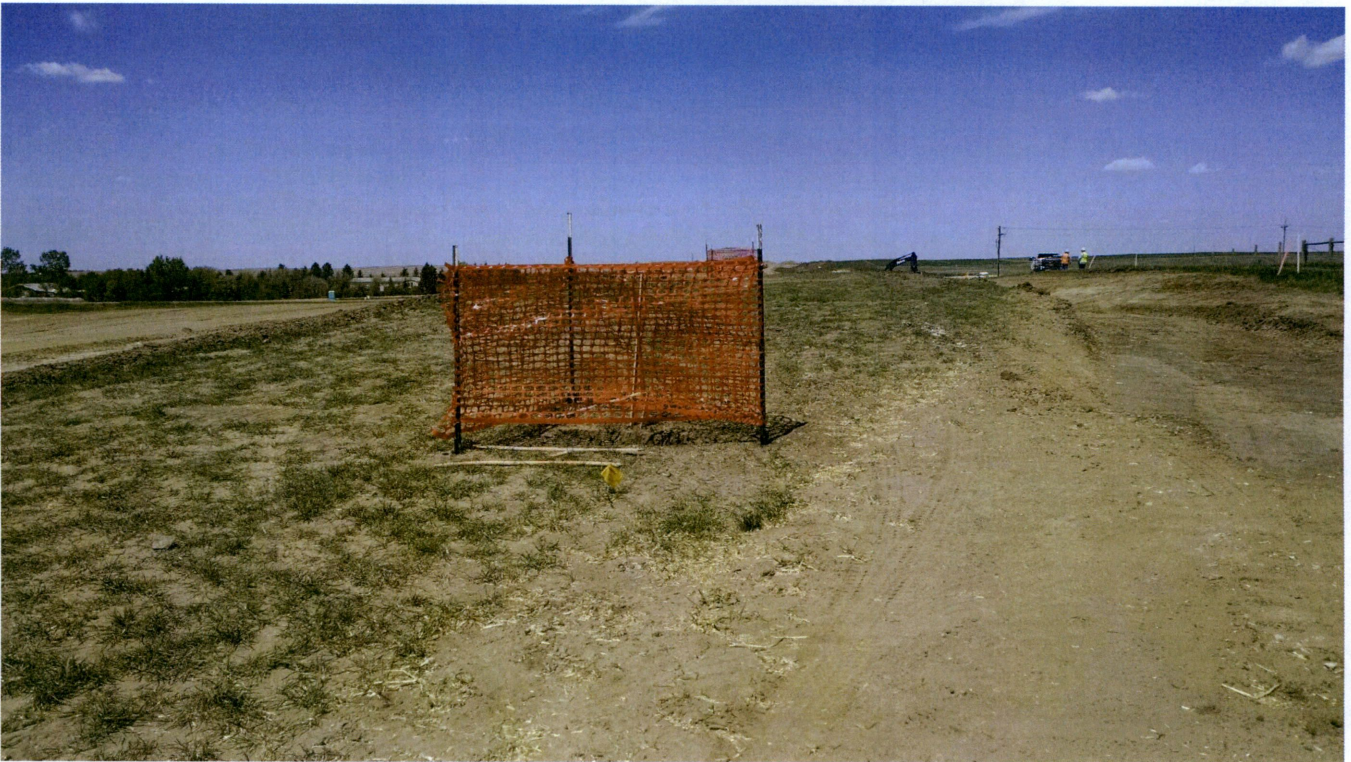
Photo 44: Station 1742+75.10, pot hole with fence
