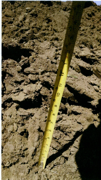
Photo 39: Station 1710+89.93, topsoil stripped, approximate depth of 12"
