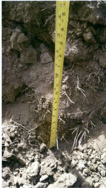
Photo 23: Station 1726+75, topsoil stripped, approximate depth of 12"
