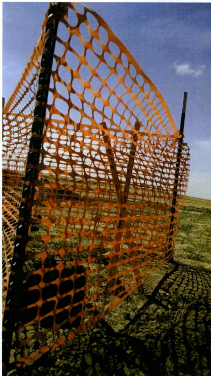
Photo 56: Station 1742+75.10, fence around pot hole
