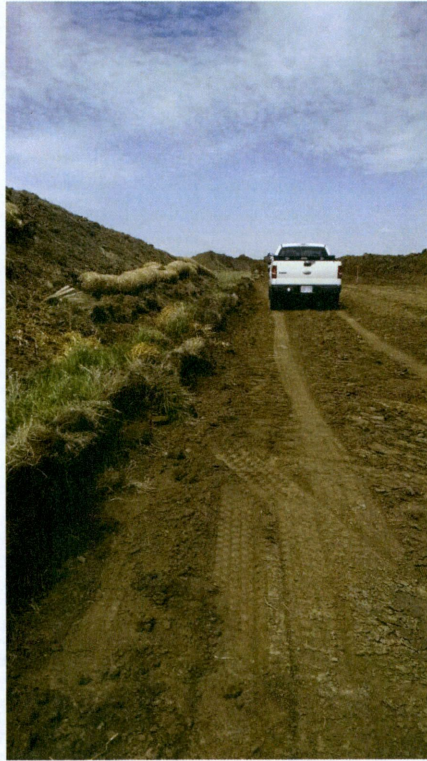
Photo 19: Station 1730+75, looking North at right-of-way being stripped and topsoil pile right
