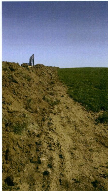
Photo 37: Station 1715+87.29, looking North at topsoil pile
