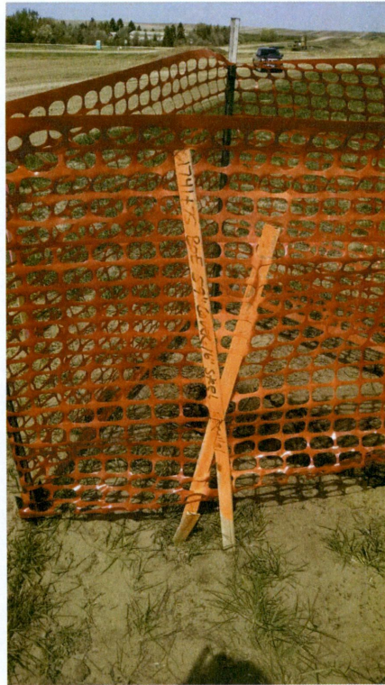
Photo I1: Station 1741+75, stake next to pot hole
