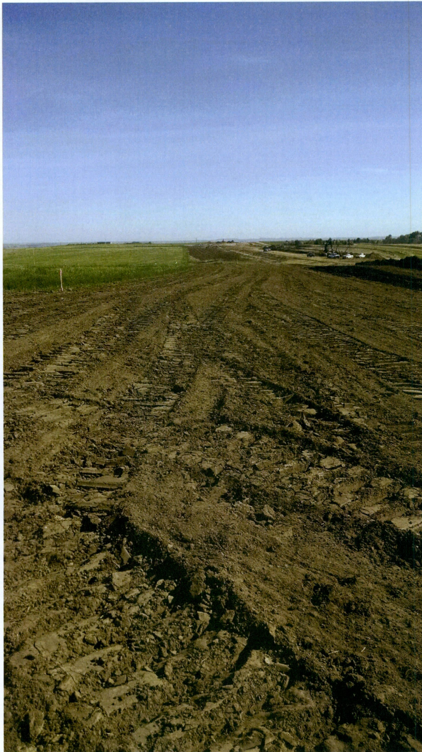
Photo 113: Station 1710+89, Looking South at completed right-of-way
