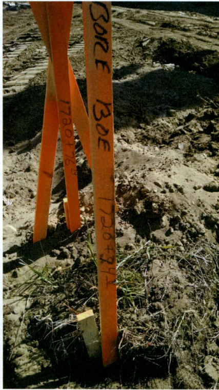
Photo 51: Station 1720+74.08, stake for centerline of pipeline, end bore
