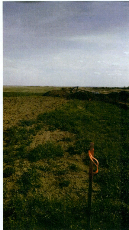
Photo 31: Station 1710+39.62, looking South at right-of-way being stripped
