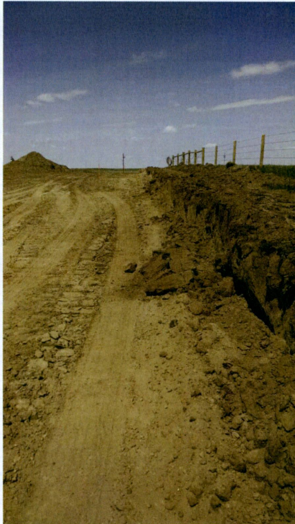
Photo 60: Station 1742+75.10, looking North at right-of-way being stripped
