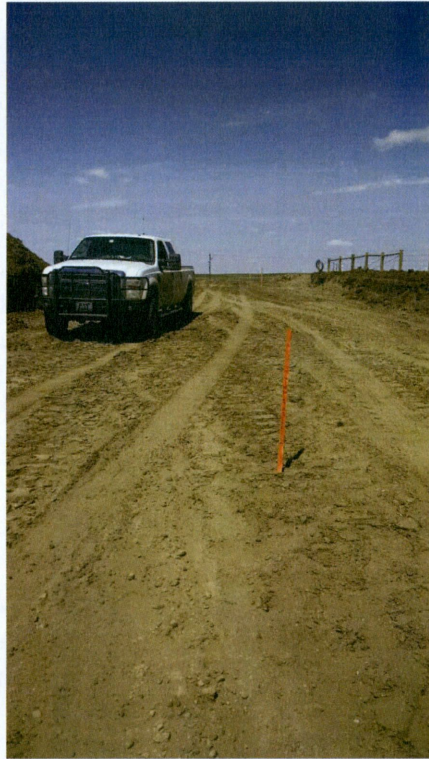
Photo 58: Station 1742+75.10, looking North at stake for centerline of reroute
