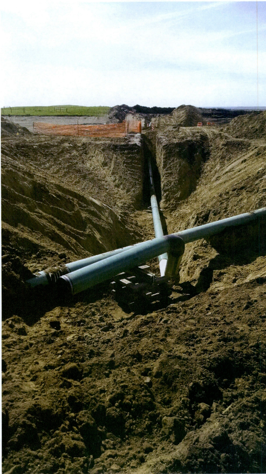
Photo 108: Station 0+00, Looking east at tie-in to mainline
