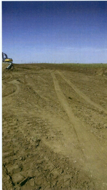
Photo 117: Station 36+91.76, Looking South at completed right-of-way over end of reroute
