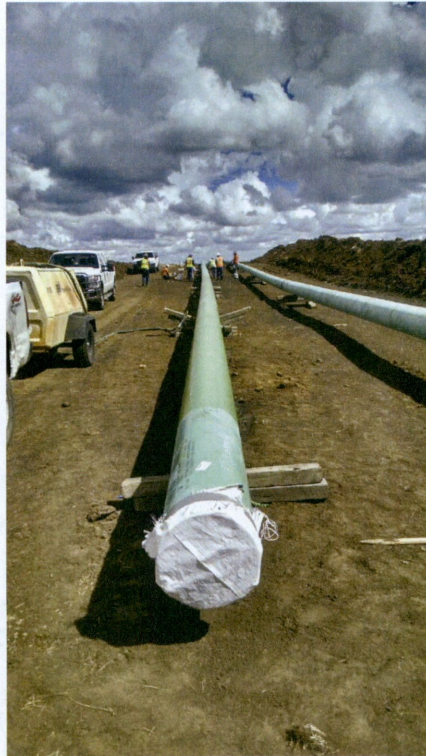
Photo 95: coating bore pipe for creek bore
