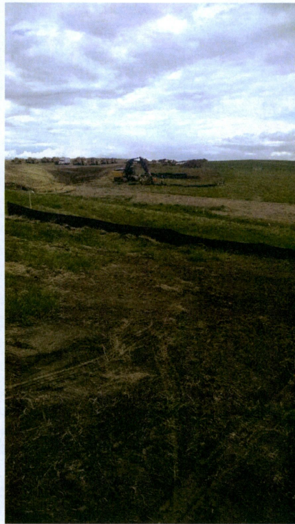
Photo 103: Station 13+85, looking North at silt fences at creek bore
