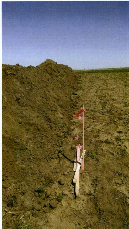
Photo 42: Station 1710+89.93, looking North at topsoil pile, contained within right-of-way
