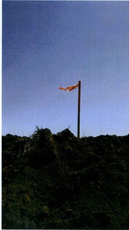
Photo 38: Station 1710+89.93, stake for centerline of pipeline
