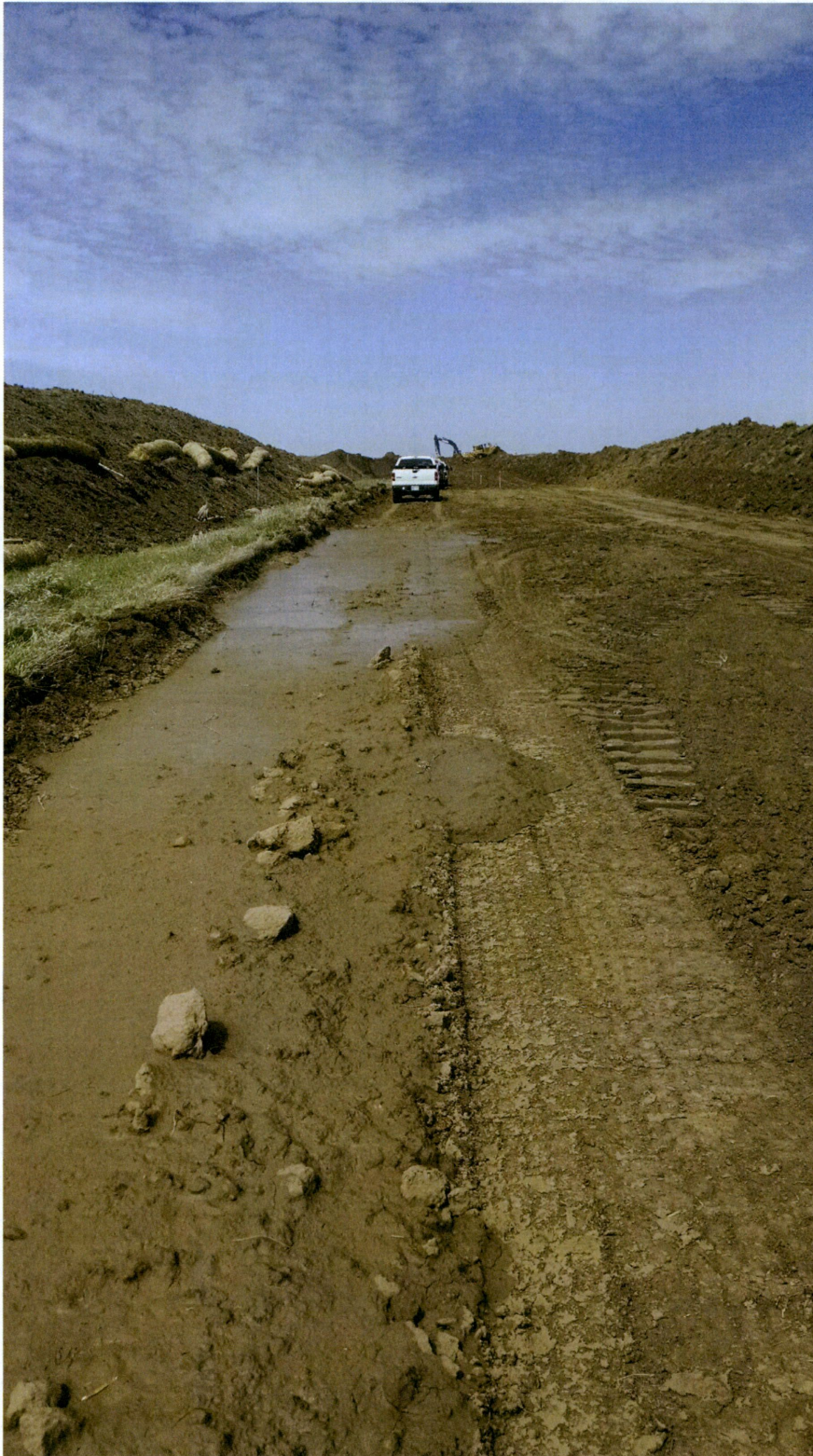
Photo 21: Station 1731+75, hydrovac dump area, looking north
