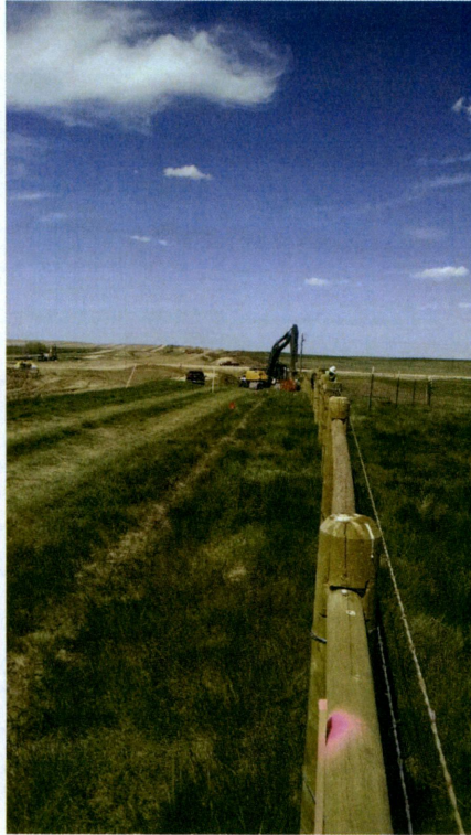
Photo 47: Station 1741+75, replacing old wood fence with steel fence east of centerline
