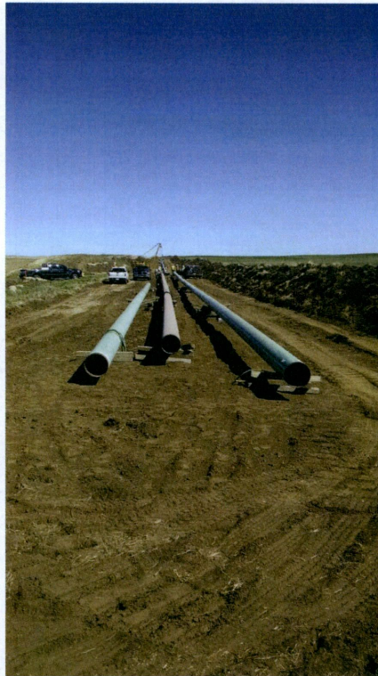
Photo 69: Station 1733+93.41, looking North at pipes to be installed
