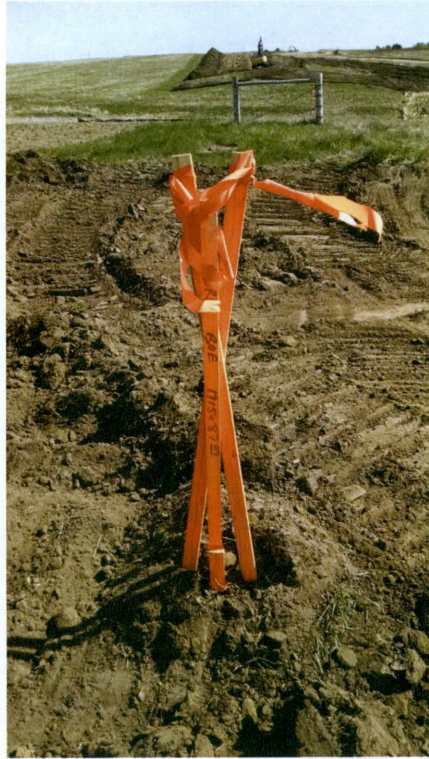
Photo 49: Station 1715+87.29, stake for centerline of pipeline, begin bore
