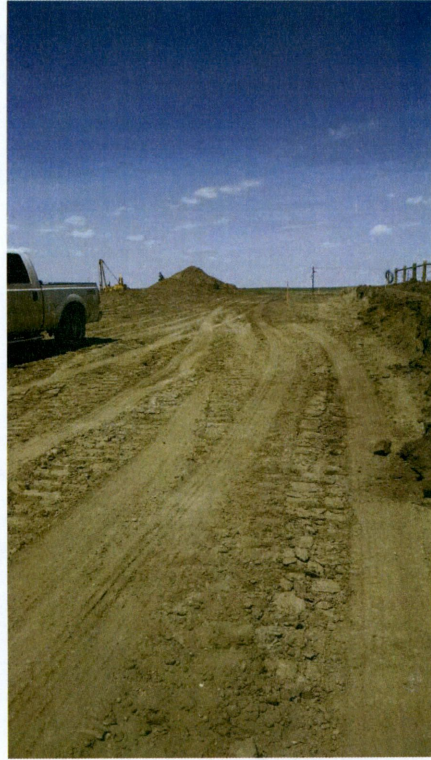
Photo 61: Station 1742+75.10, looking North at right-of-way being stripped
