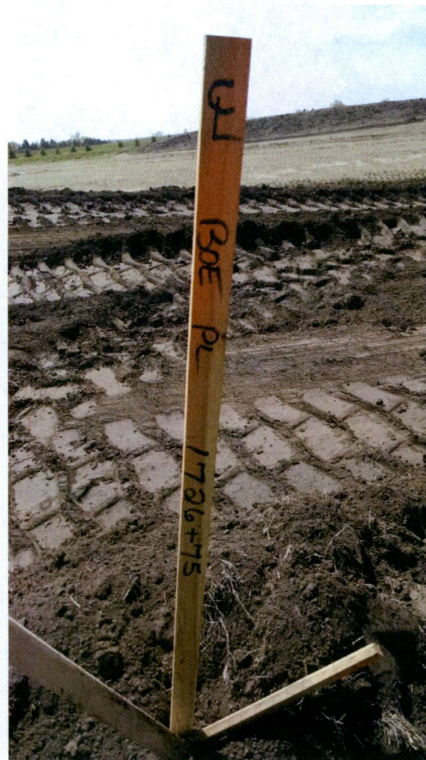
Photo 25: Station 1726+75, stake for centerline of pipeline
