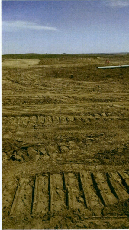
Photo 116: Station 0+00, Looking East at completed right-of-way over tie-in to mainline
