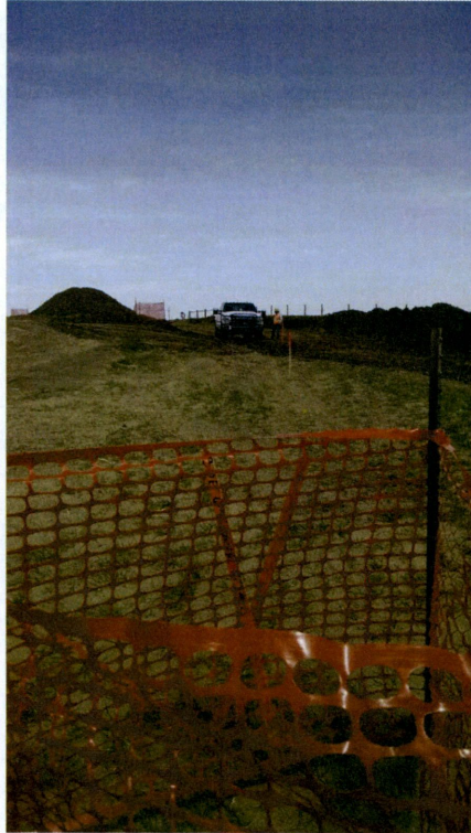
Photo 55: Station 1742+75.10, looking North, topsoil pile on left
