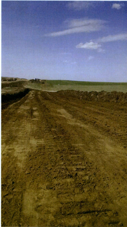
Photo 29: Station 1723+50, looking North at right-of-way being stripped and topsoil pile right
