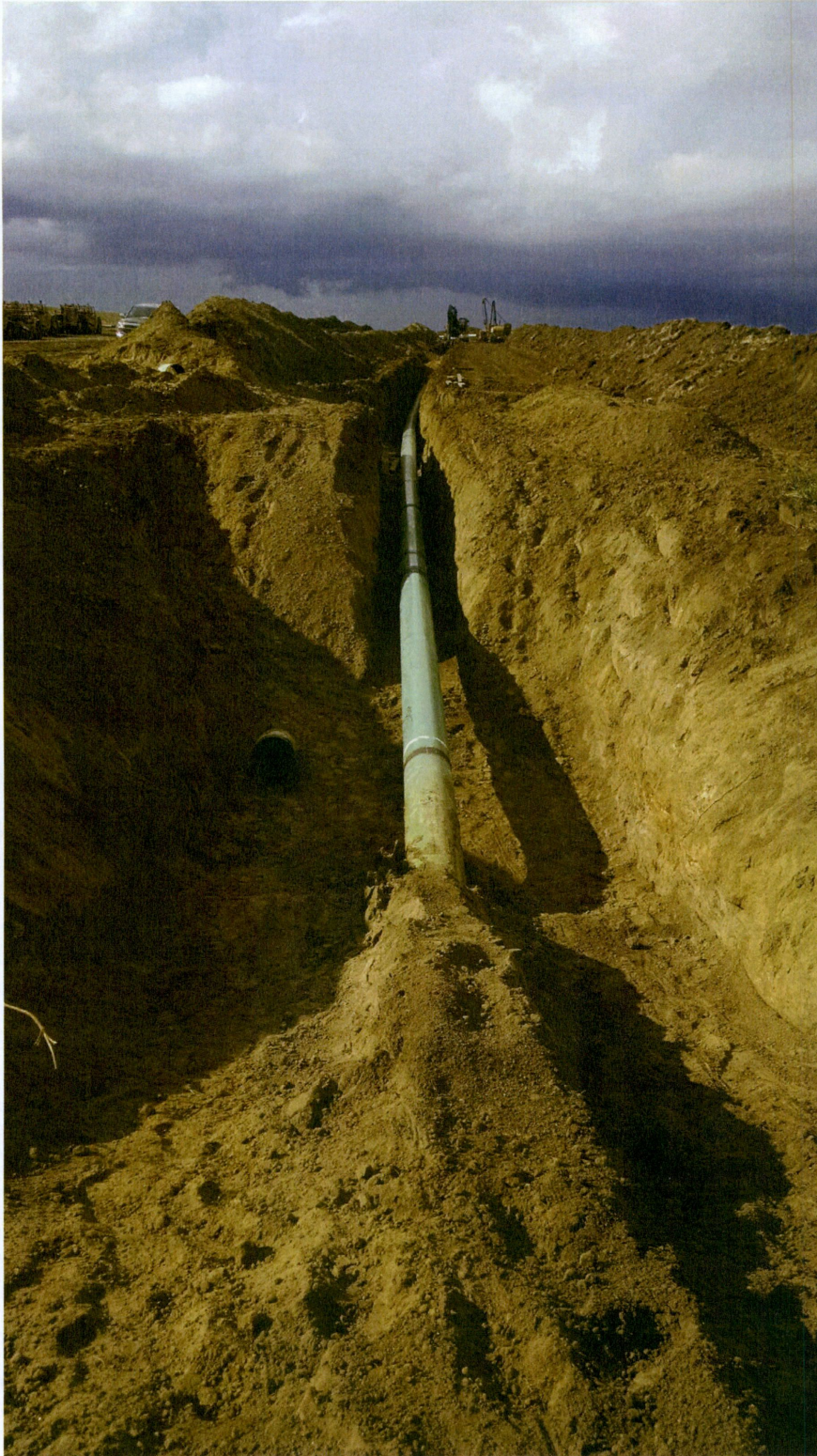
Photo 106: Station 8+91, looking North at bore pipe at creek crossing
