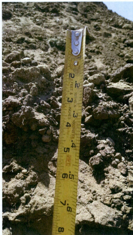
Photo 67: Station 1741+75, topsoil stripped, approximate depth of 12"
