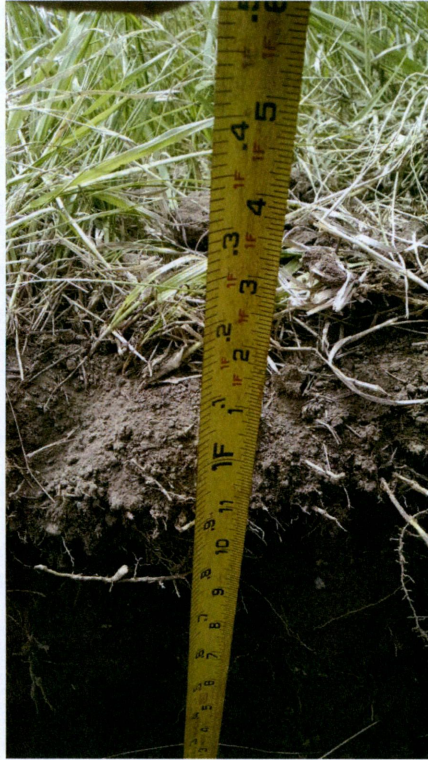
Photo 17: Station 1730+75, topsoil stripped, approximate depth of 12"
