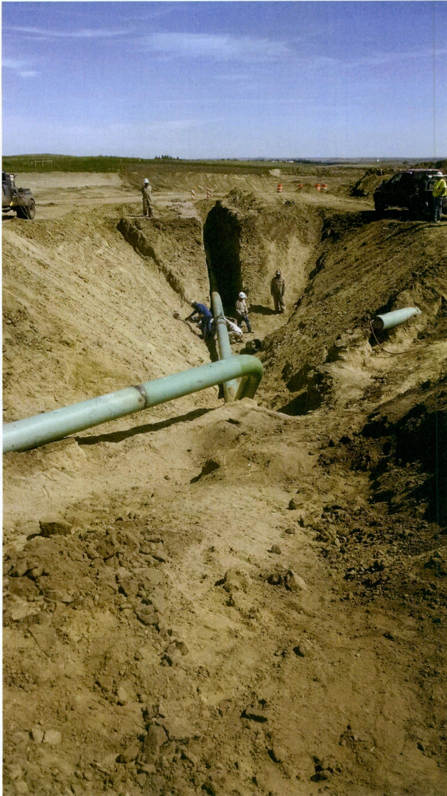
Photo 110: Station 0+00, Reroute tied in to mainline, looking East
