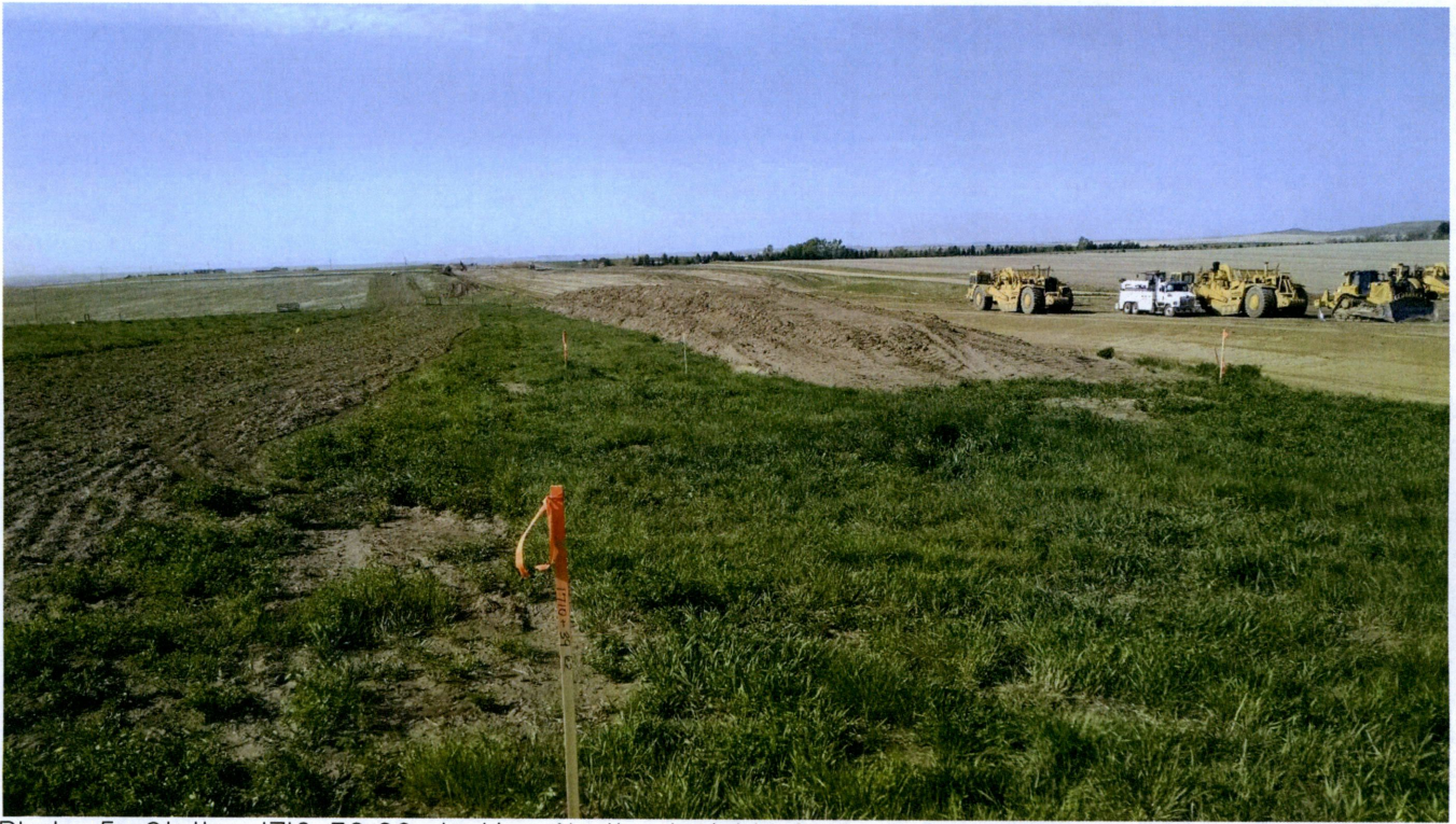
Photo 5: Station 1710+39.62, looking North at right-of-way being stripped and topsoil pile
