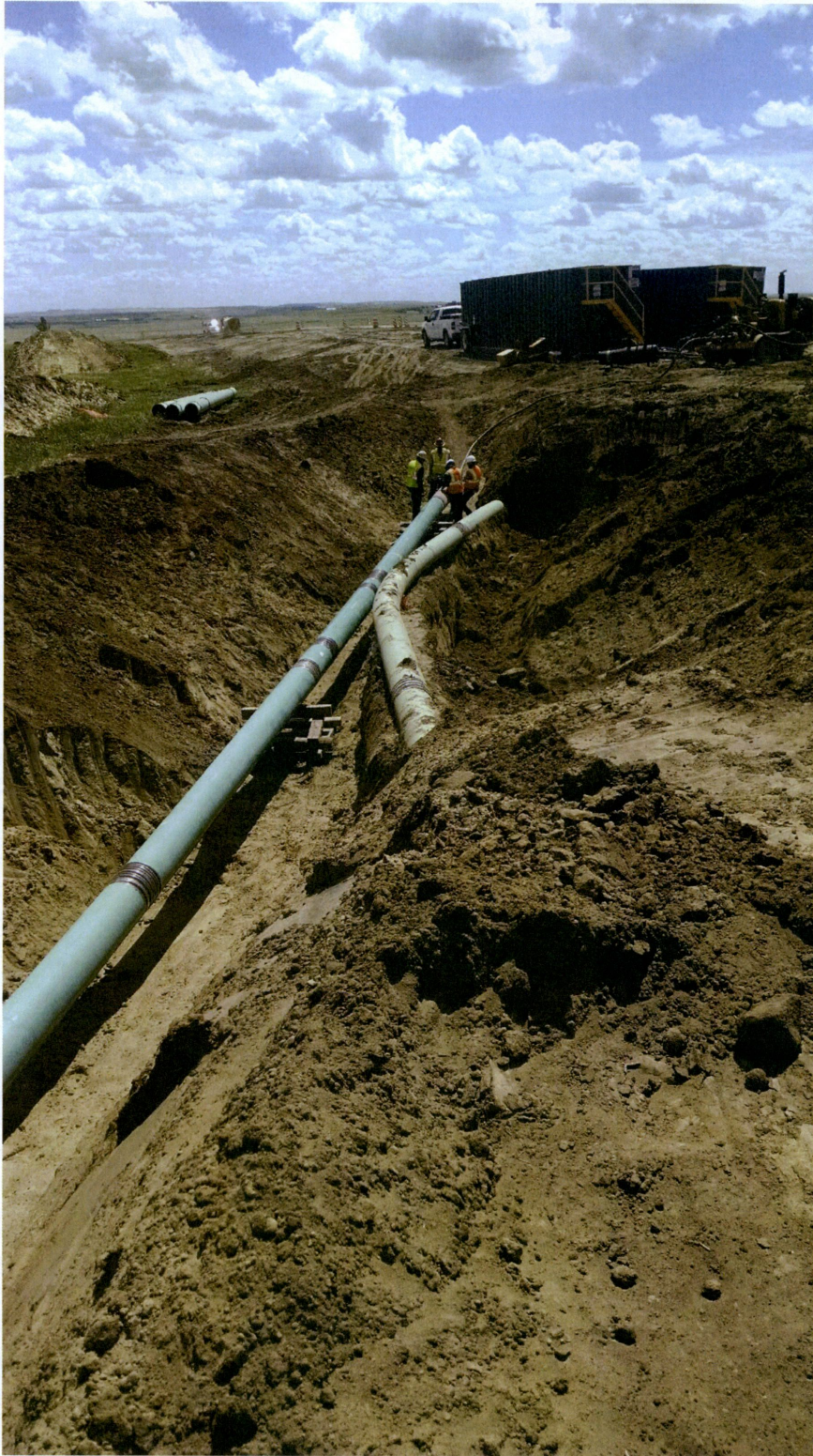
Photo 109: Tie-in at end of project, looking Southeast
