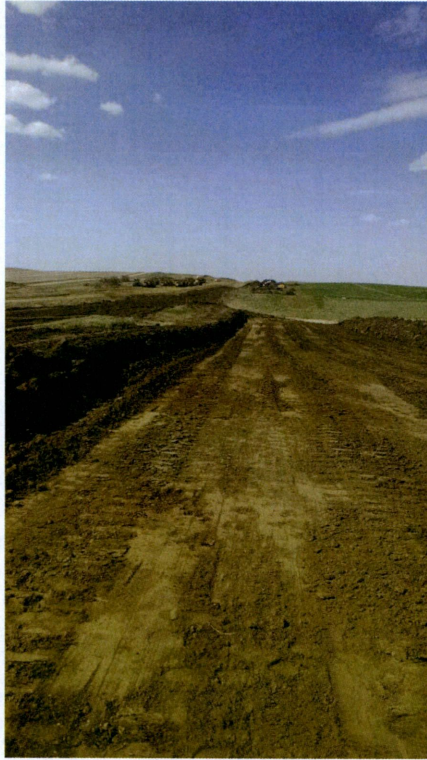
Photo 28: Station 1723+50, looking North at right-of-way being stripped
