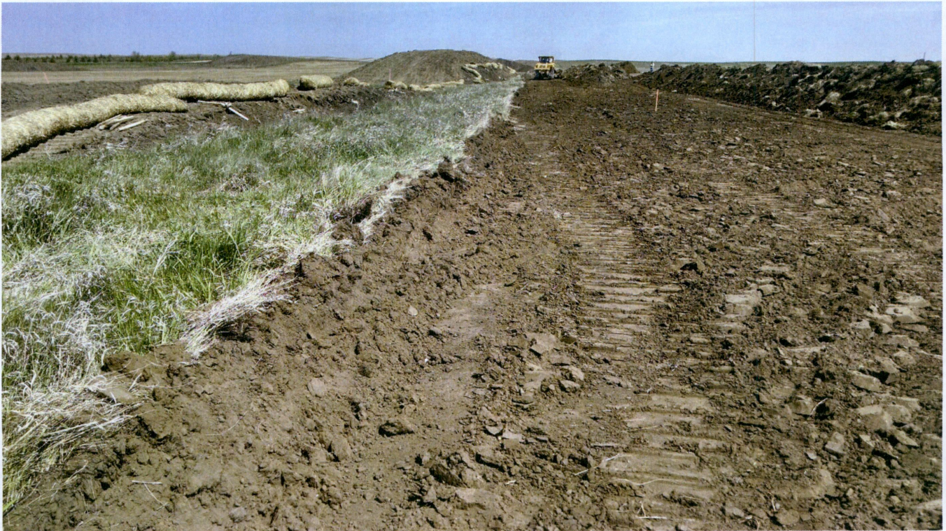
Photo 7: Station 1710+39.62, topsoil stripped, topsoil pile to the right
