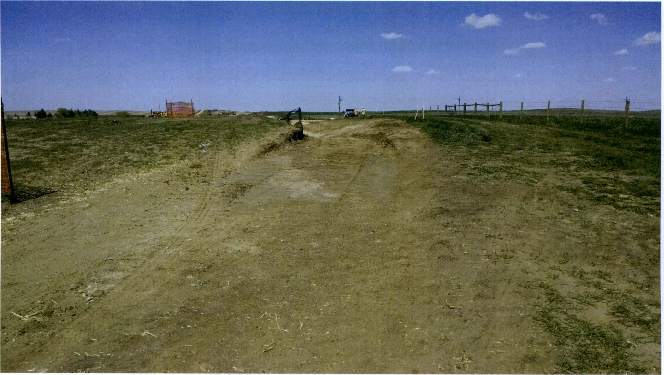
Photo 43: Station 1742+75.10, looking North at right-of-way being stripped
