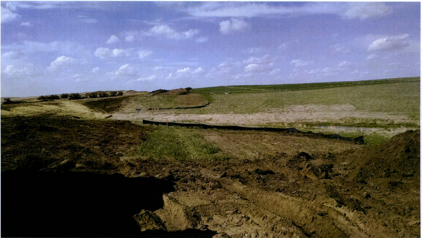
Photo 52: Station 1720+74.08, looking North at silt fence
