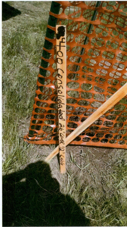
Photo 15: Station 4+00, stake next to pot hole
