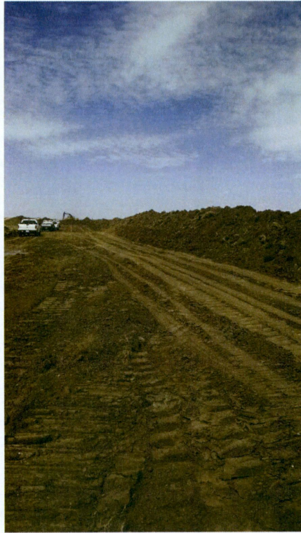
Photo 22: Station 1726+75, looking North at right-of-way being stripped and topsoil pile right
