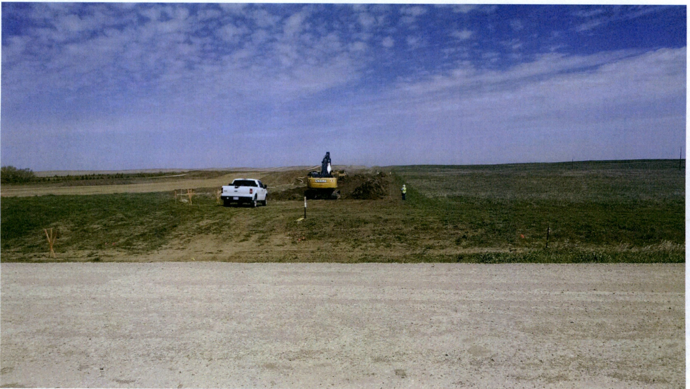
Photo 6: Station 1710+39.62, right-of-way being stripped
