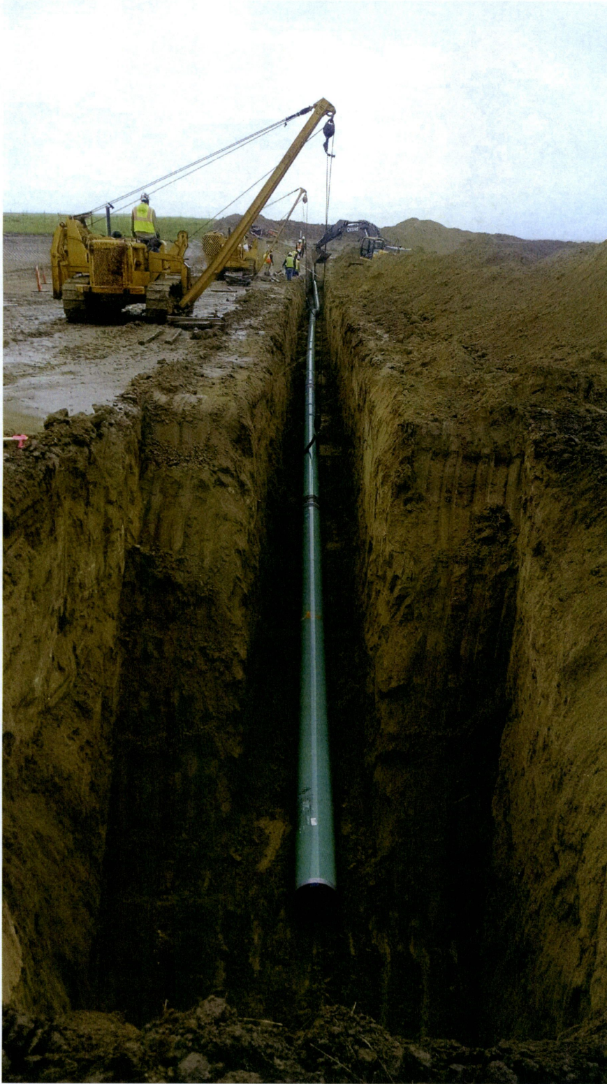
Photo 107: Station 0+00, looking east at tie-in, 12 foot deep trench
