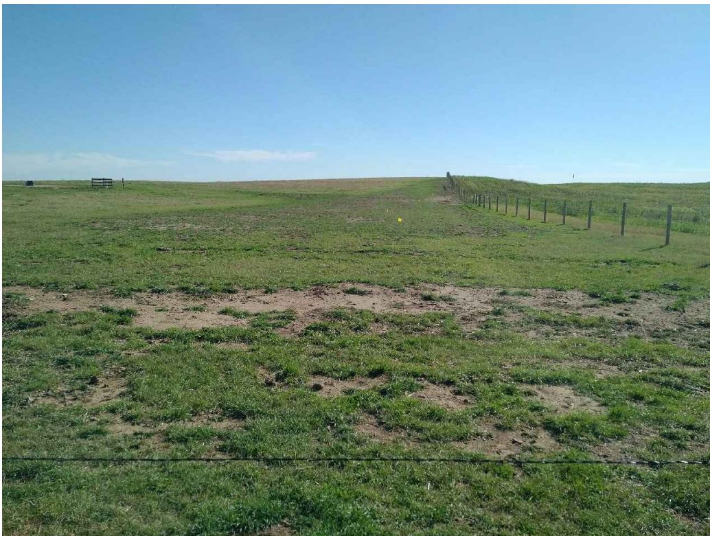
Photo 14: Station 30+00, Looking South
