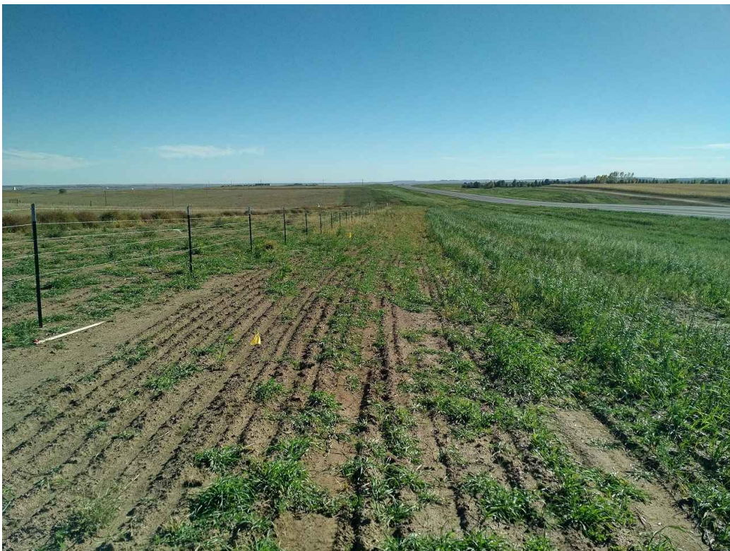
Photo 6: Station 5+00, Looking South
