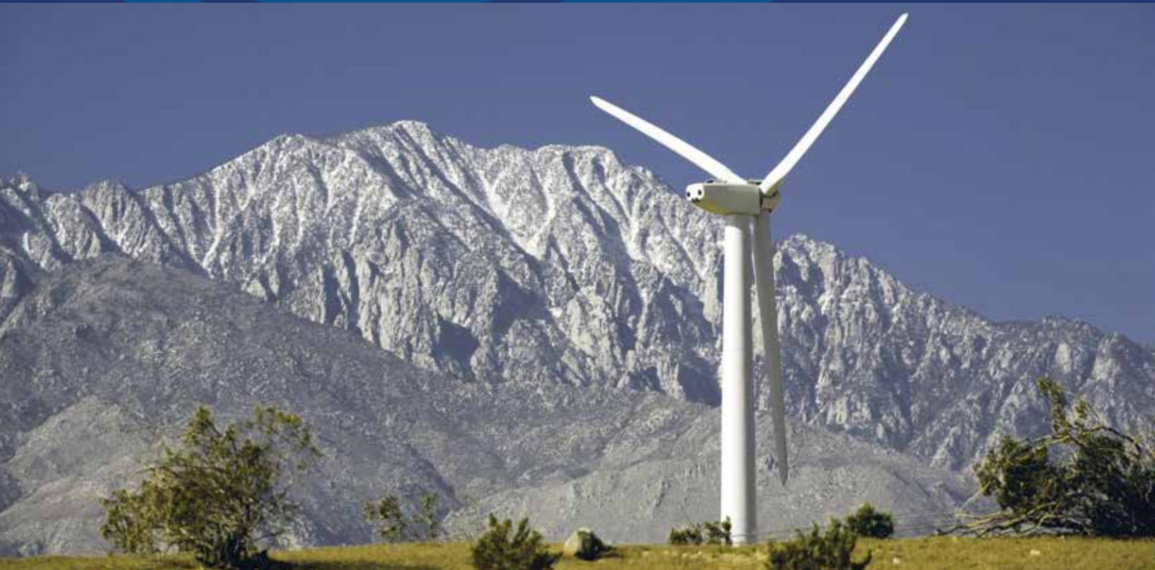
DILLON WIND POWER PROJECT, PHOTO BY IBERDROLA RENEWABLES, INC., NREL 16105
