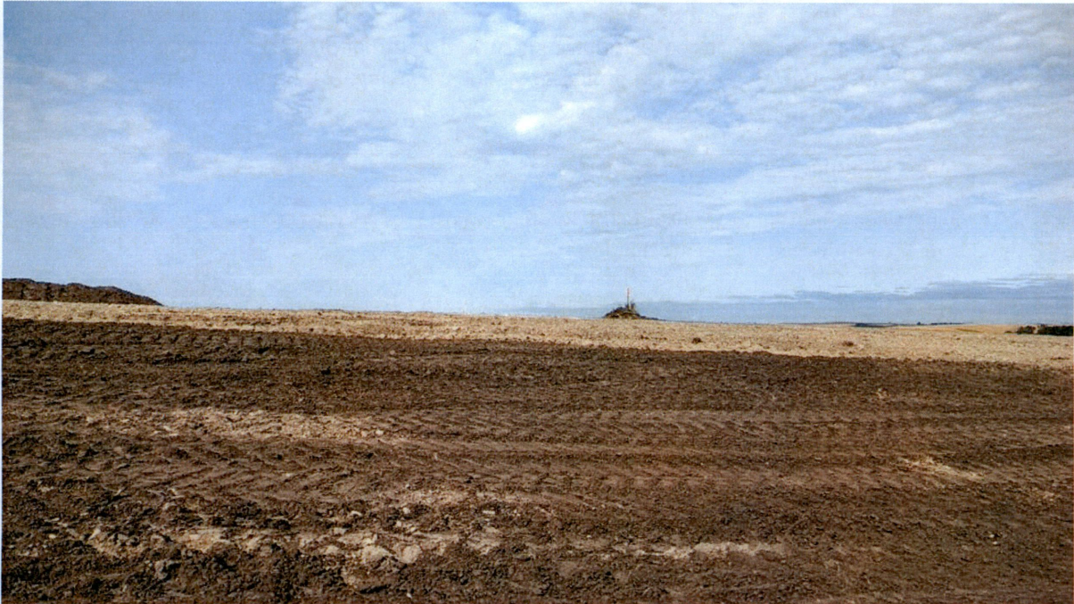
Report Photo #1 "Lighter Subsoil Visible After Scraper Pass" (Coordinates: 46.945262, -101.18663)
