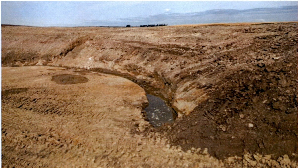
Report Photo #2 "Ground Water Encountered While Excavating on Turbine Pad" (Coordinates: 46.961692, -101.232544)
