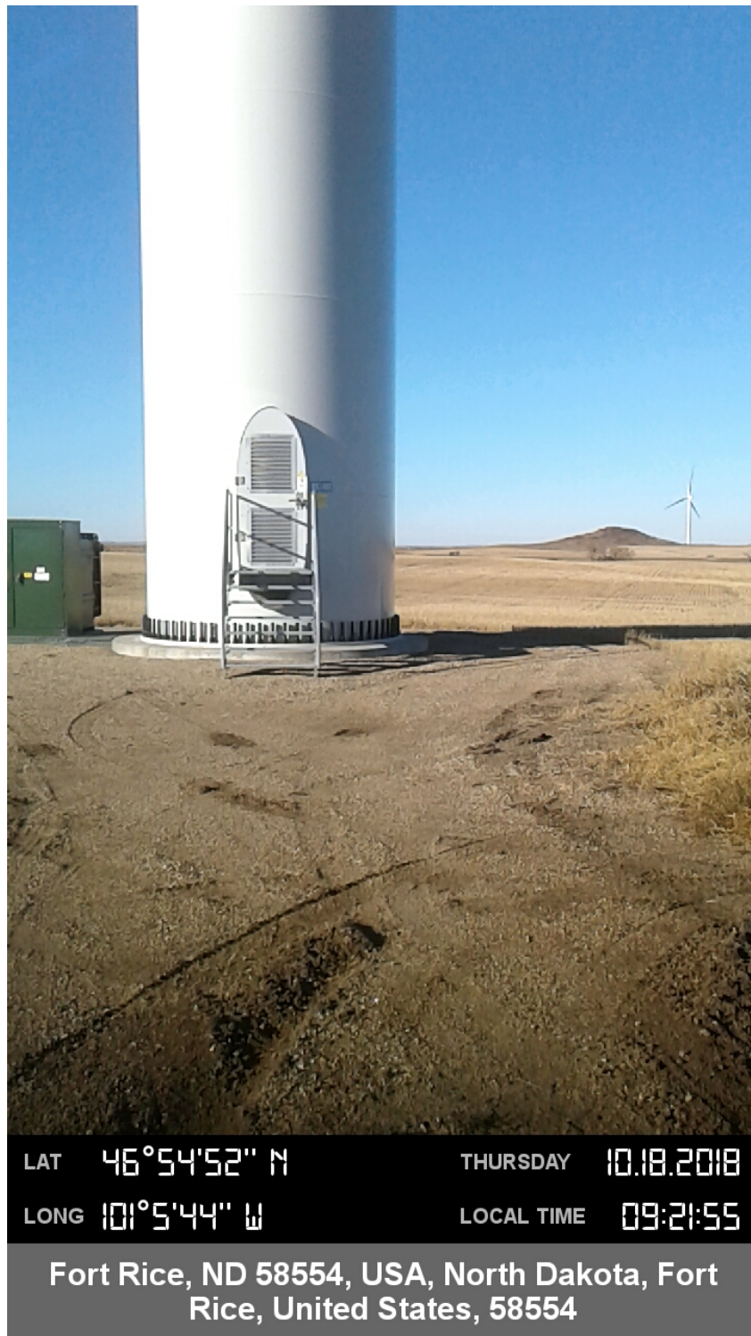
Report Photo #5: Overview of turbine construction block (T1) from South to North.
