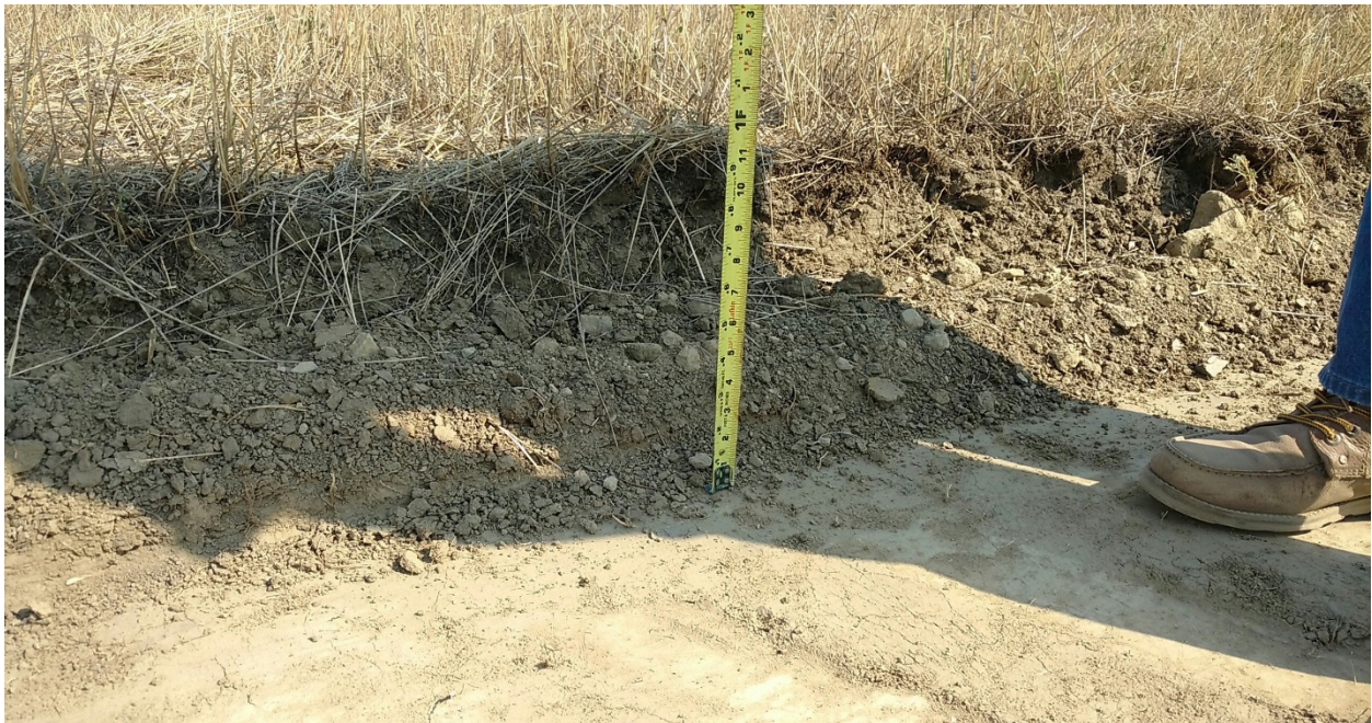
Photo 19: Located at station 81+00, showing stripped Right of Way with approximate topsoil depth of 12 inches. Photo is showing north side of Right of Way.
