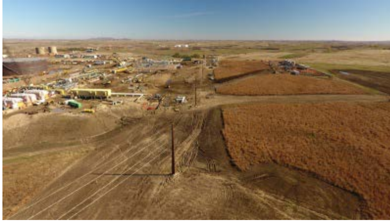
Photo 1: Station 11+45; Latitude: 47°47'53.19"N Longitude: 102°55'33.03"
