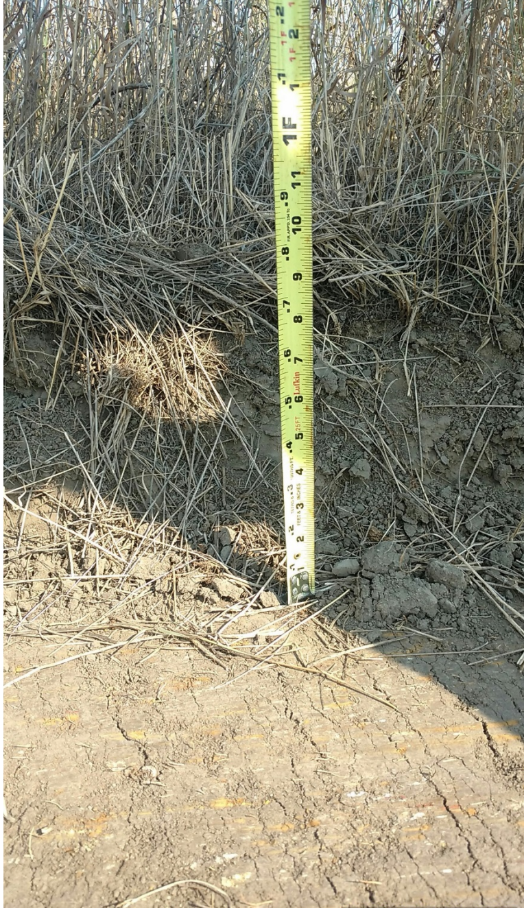
Photo 10: Located at station 40+00, photo showing stripped Right of Way at approximate topsoil depth of 12 inches. Photo is showing south side of Right of Way.
