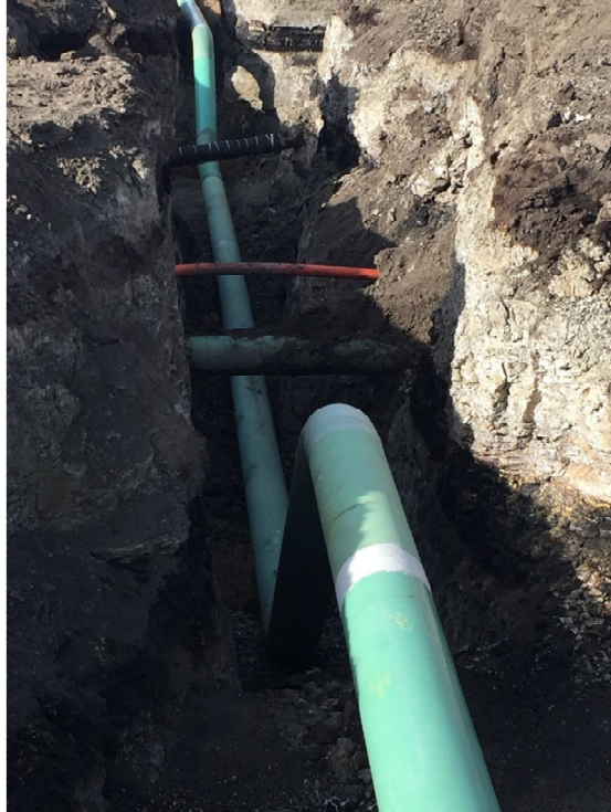
Picture 28: Utility crossing completed west of PI near station 60+00
