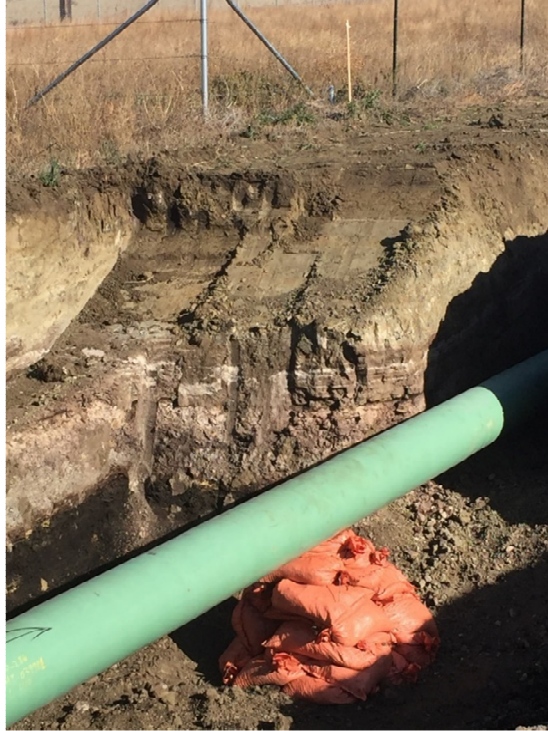
Picture 21: Pipe leveled on sandbags to make connection at PI
