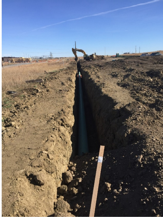
Picture 19: Backfill in progress
