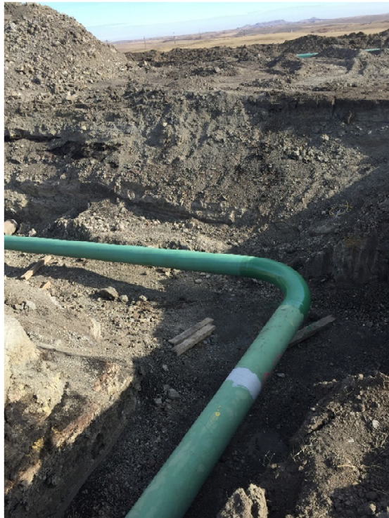
Picture 25: Point of intersect west of Johnsons Corner Terminal
