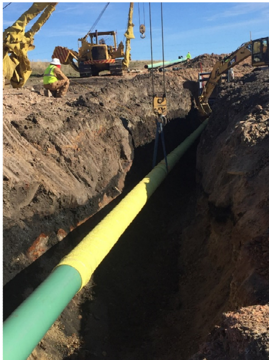
Picture 8: Placing pipe near utility crossing
