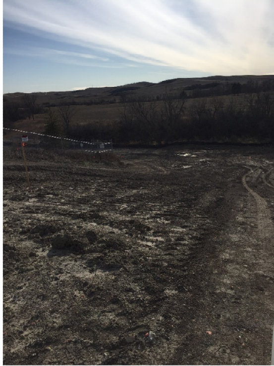
Picture 24: PI near Johnsons Corner Terminal backfilled
