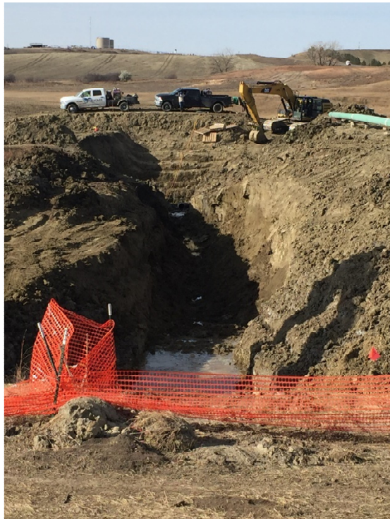
Picture 27: Excavating for trench near Highway 73 bore
