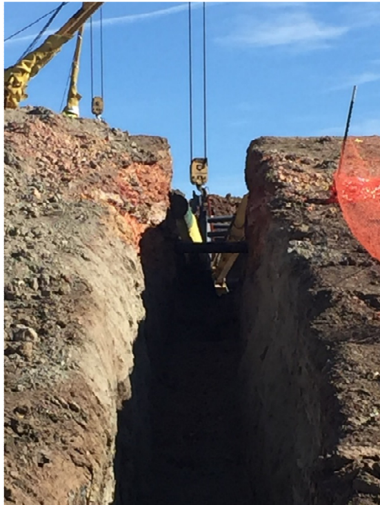
Picture 10: Installing pipe at utility crossing
