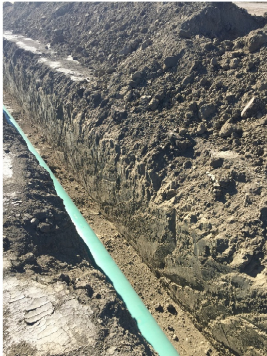
Picture 4: Laying pipe, cover verified greater than 4 feet.
