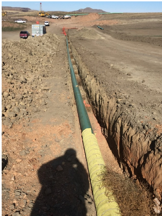
Picture 12: Pipe laid in trench, preparing for backfill
