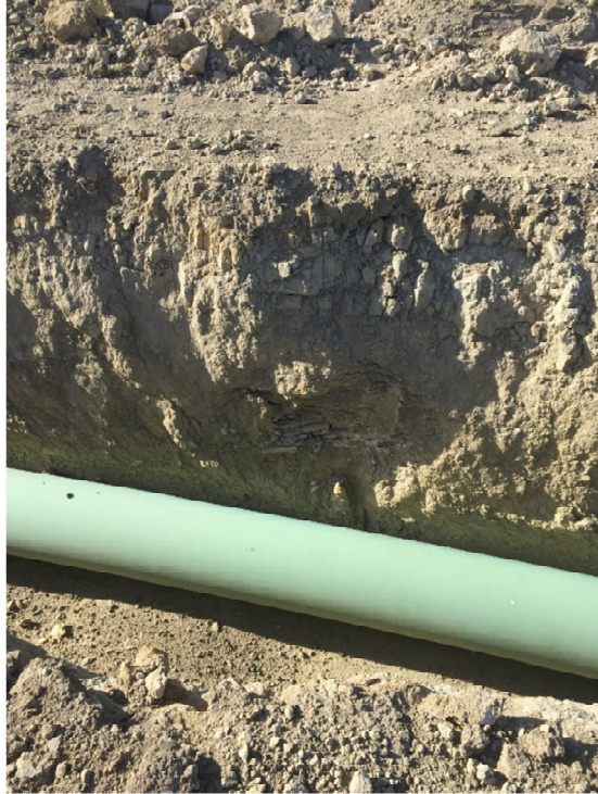
Picture 13: Pipe recently placed in trench
