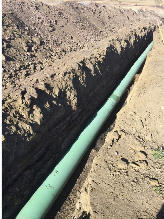
Picture 17: Pipe ready for backfill, minimum depth requirements verified
