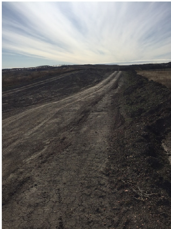
Picture 29: Backfill completed, prior to topsoil placement
