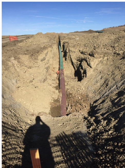
Picture 2: Pipe bore/trench. Depths checked at 4 feet or greater cover in trench.
