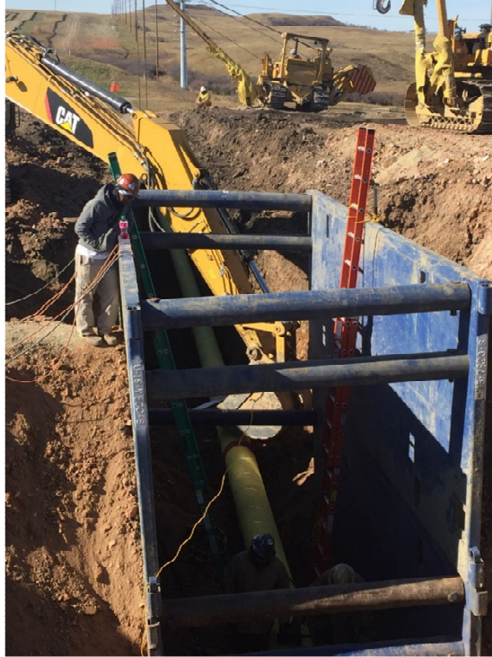
Picture 7: Utility crossing
