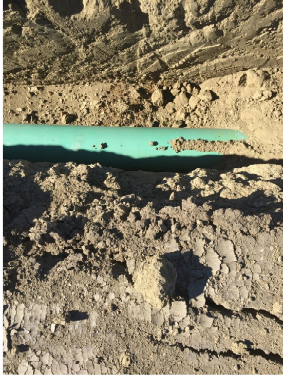
Picture 3: Pipe backfill
