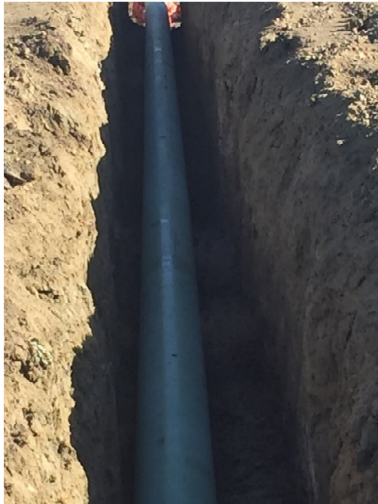
Picture 20: Backfill in progress
