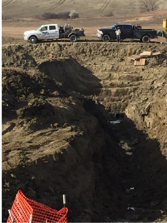
Picture 26: Excavating for trench near Highway 73 bore
