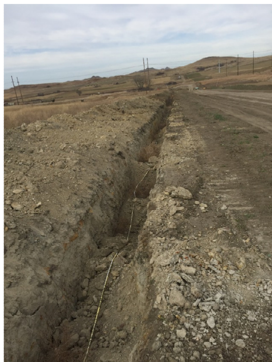
Picture 23: Backfilling, warning tape placed in trench
