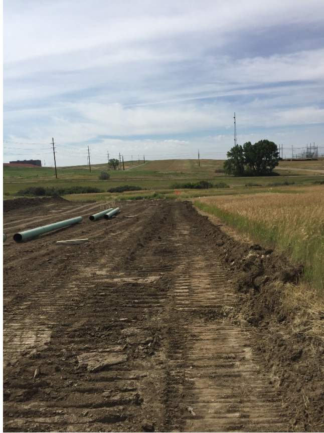
Photo 32: Sta. 147+00 looking south.
