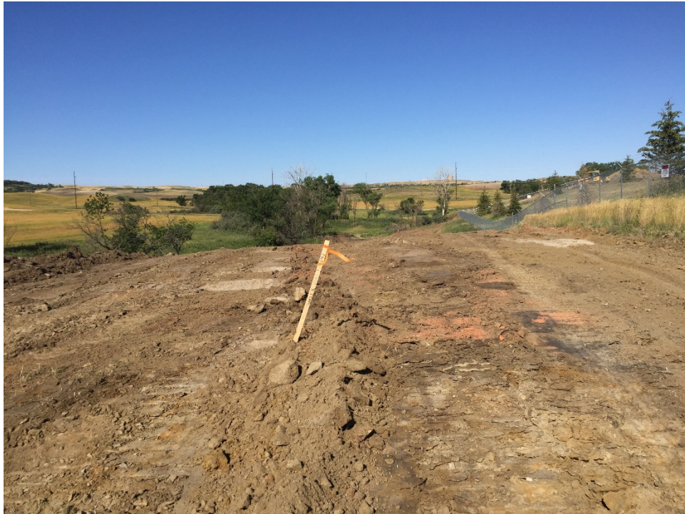
Photo 4: Sta. 4+00 looking west
