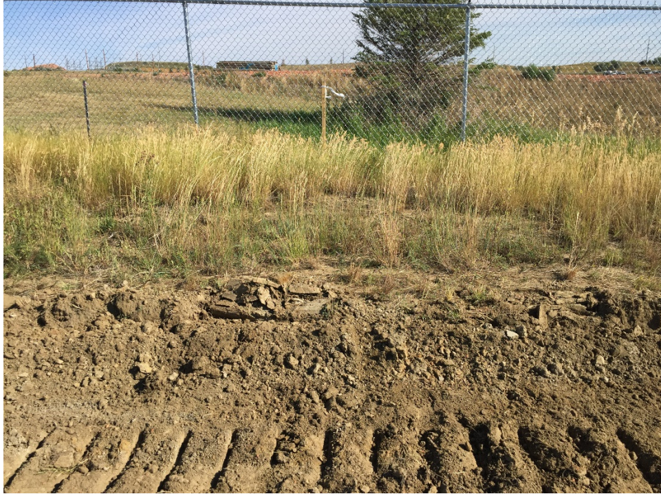
Photo 5: Sta. 4+00 showing top soil removal depth
