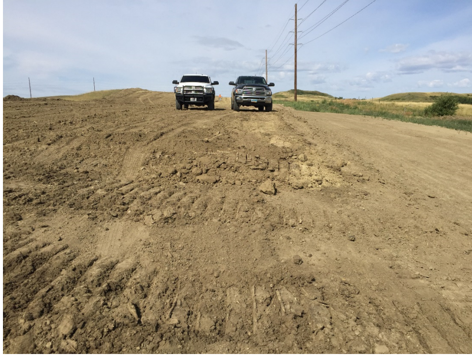
Photo 16: Sta. 92+00 looking west
