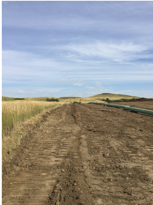
Photo 31: Sta. 146+00 looking north.
