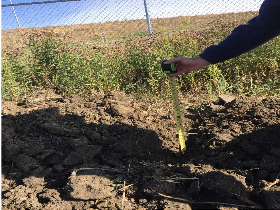
Photo 3: Sta. 3+00 showing 8 inches topsoil removal
