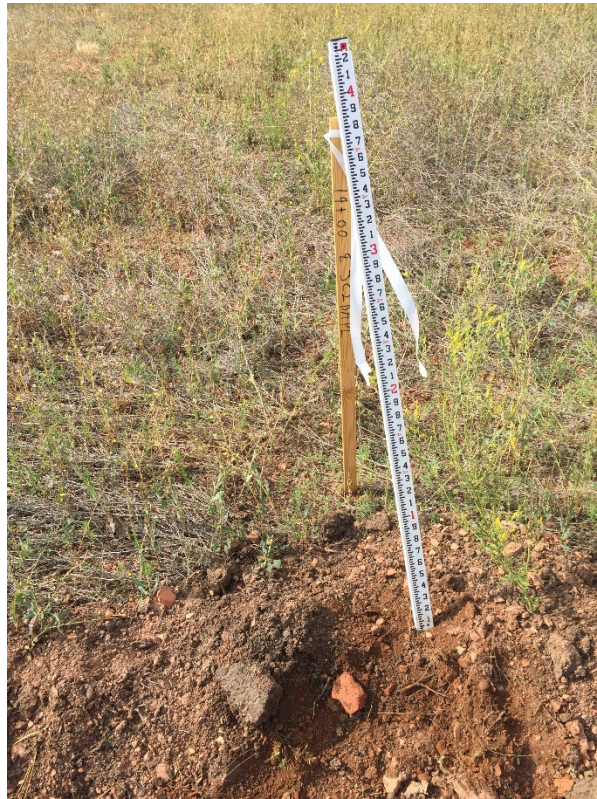
Photo 11: Sta. 14+00, 7 inches topsoil removed.
