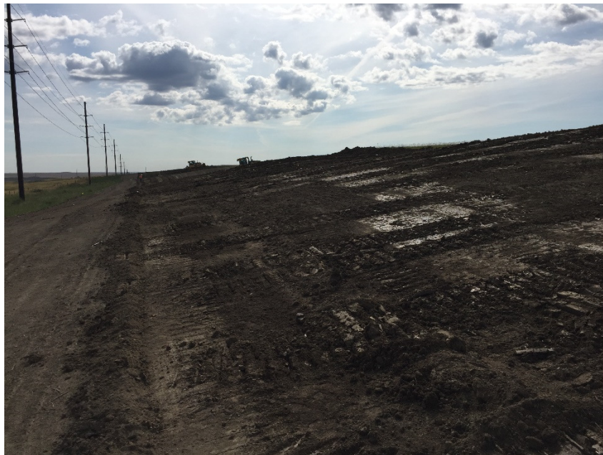
Photo 15: Sta. 92+00 looking east.
