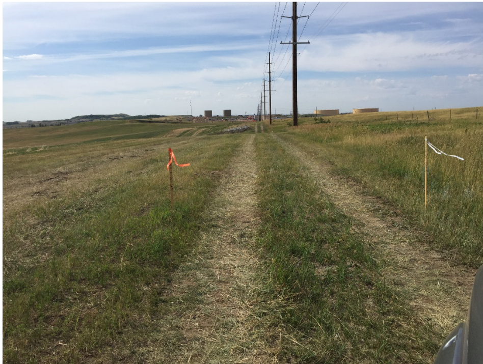
Photo 23: Sta. 113+00 area to be bored.
