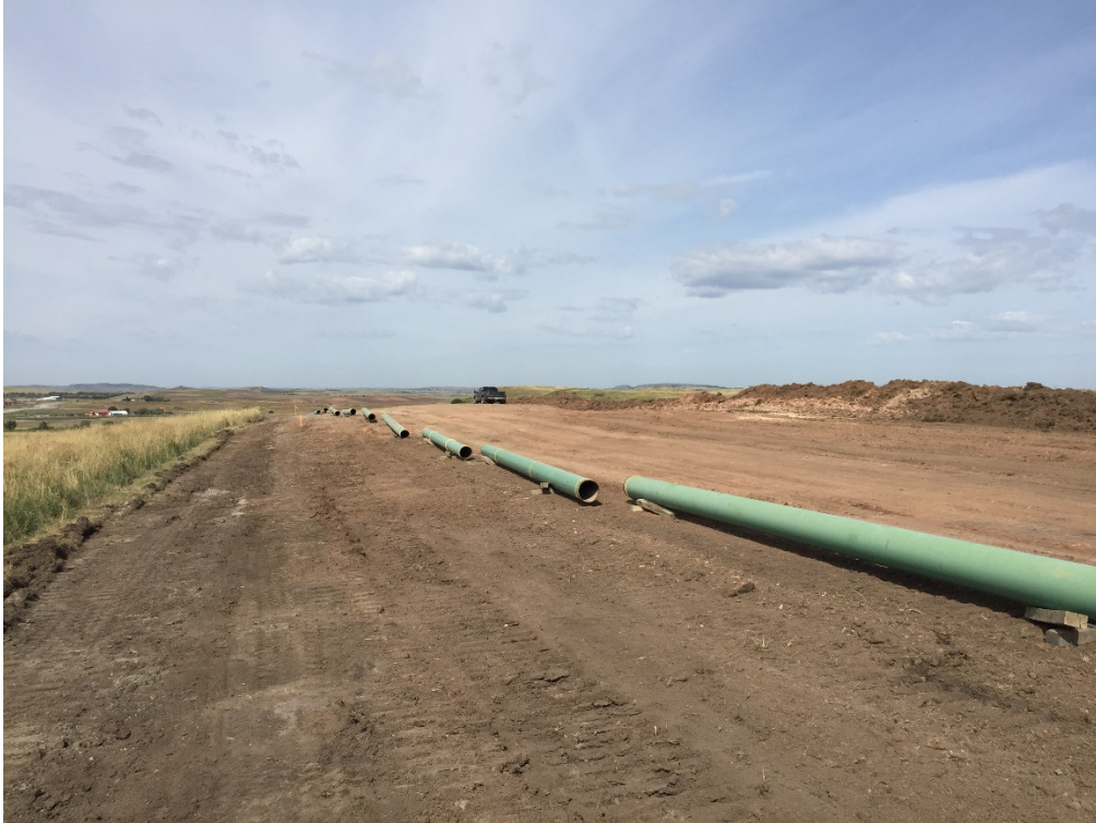
Photo 26: Sta. 130+00 looking west.
