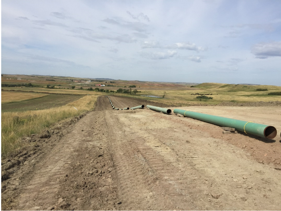
Photo 28: Sta. 142+00 Looking west.
