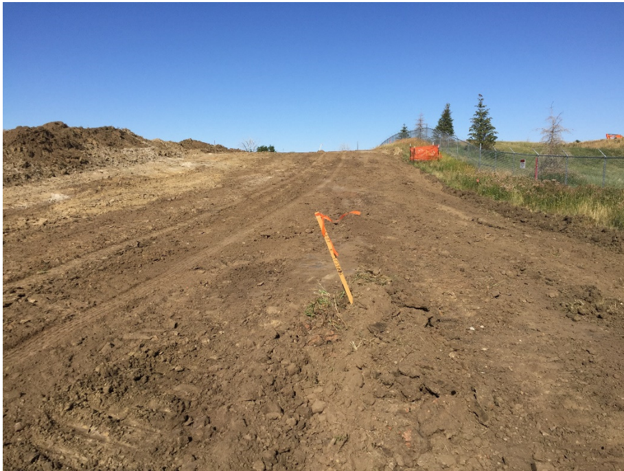
Photo 2: Sta. 3+00 looking west
