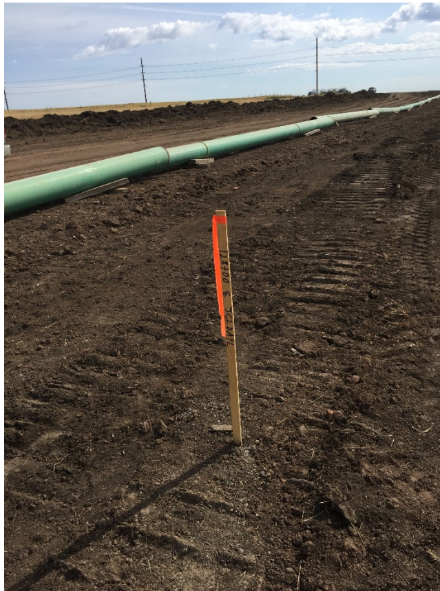
Photo 25: Sta. 128+00 pipe staged, preparing to weld.
