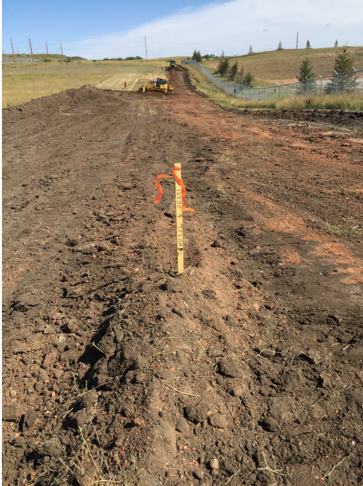
Photo 9: Sta. 12+00 looking north showing an old road under the stripping of limited top soil
