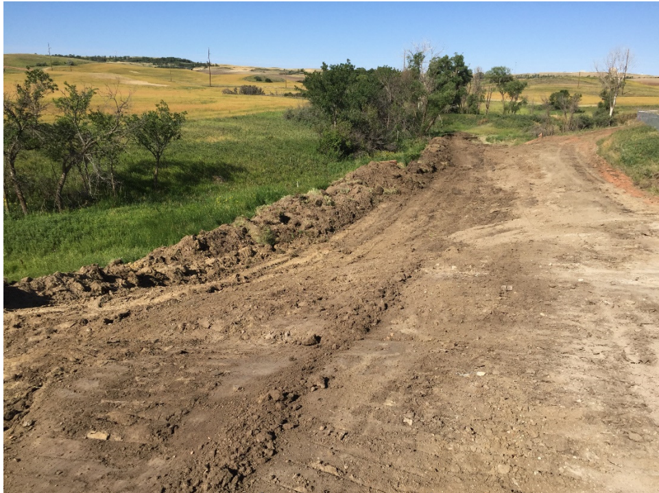
Photo 6: Sta. 5+50 looking west showing top soil pile along drainage area. See photo 10 on August 8 showing replacement of topsoil stockpile with silt fence.
