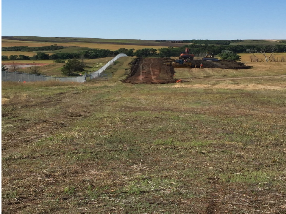
Photo 7: Sta. 13+00 looking south showing stripping operation and equipment
