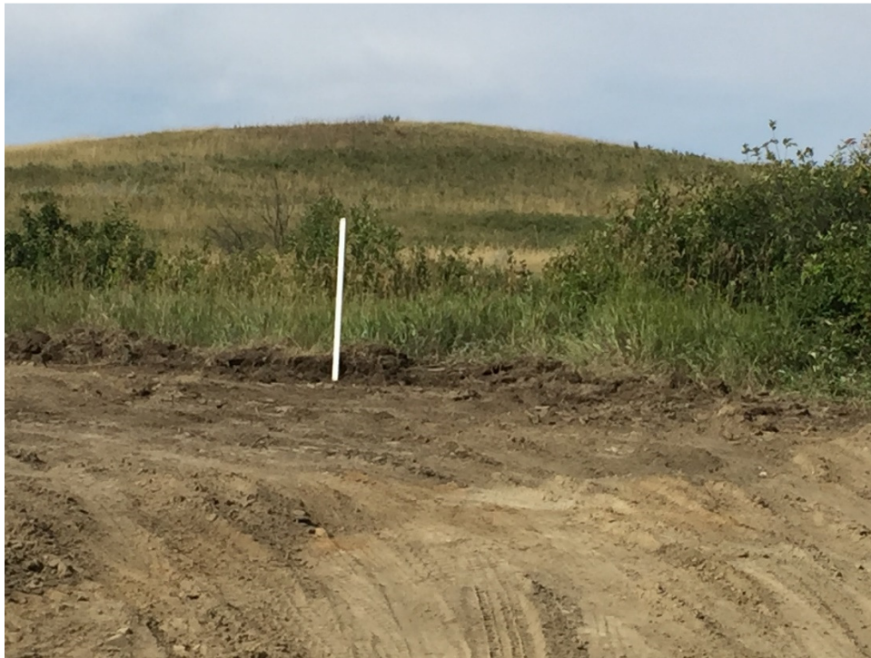
Photo 21: Sta. 108+00, 8-10 inches of topsoil.
