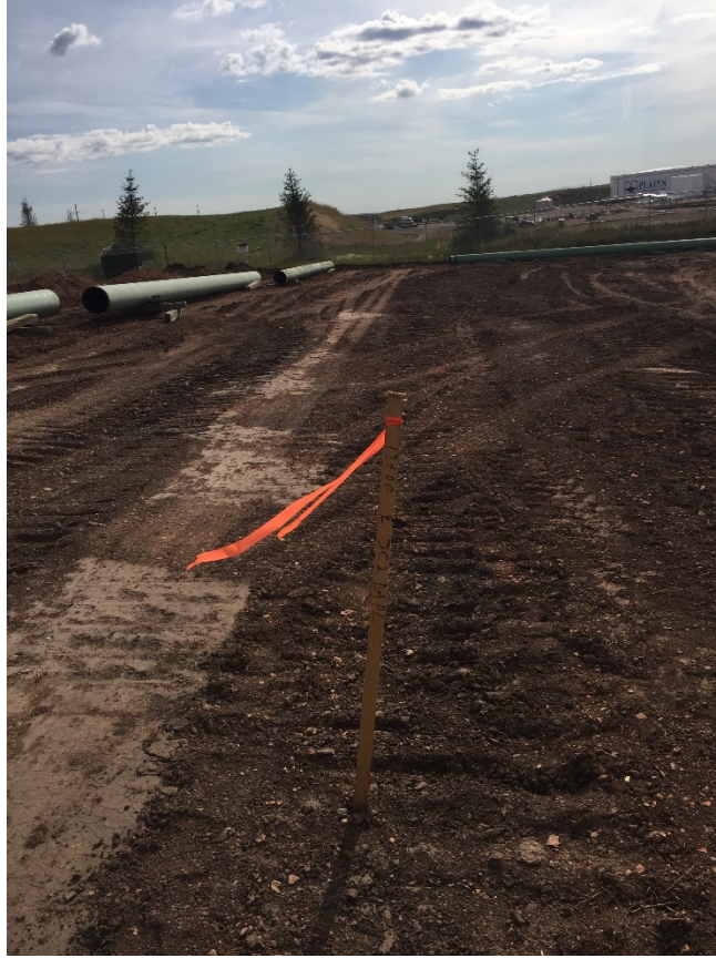
Photo 12: Sta. 19+00 looking east, pipe being delivered.
