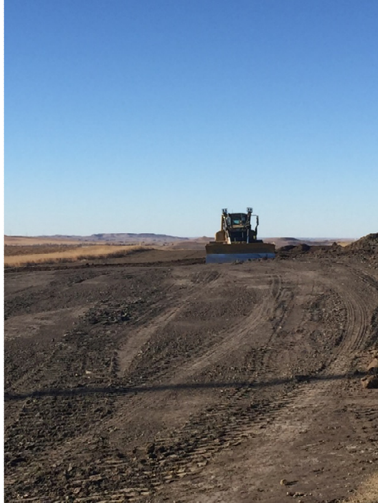
Picture 30: Topsoil spreading in progress, looking west
