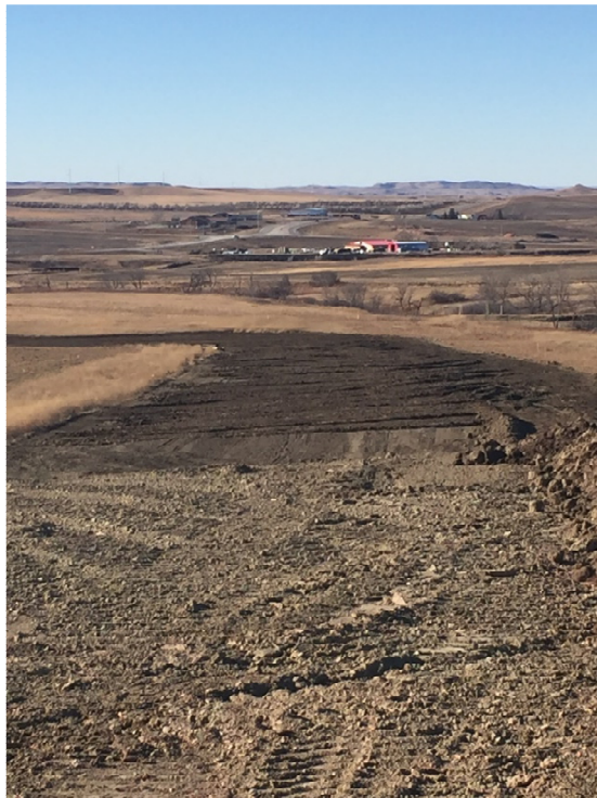
Picture 33: Topsoil spreading completed, looking west
