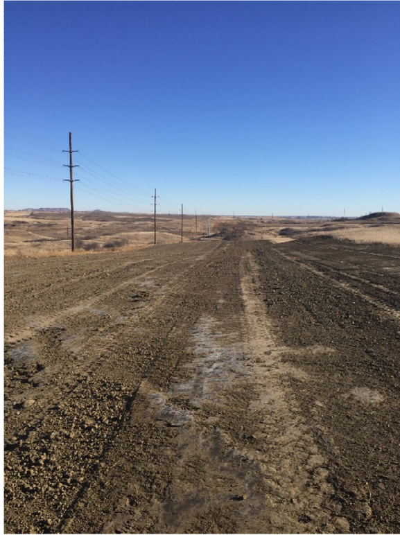
Picture 22: Topsoil spreading completed, looking east
