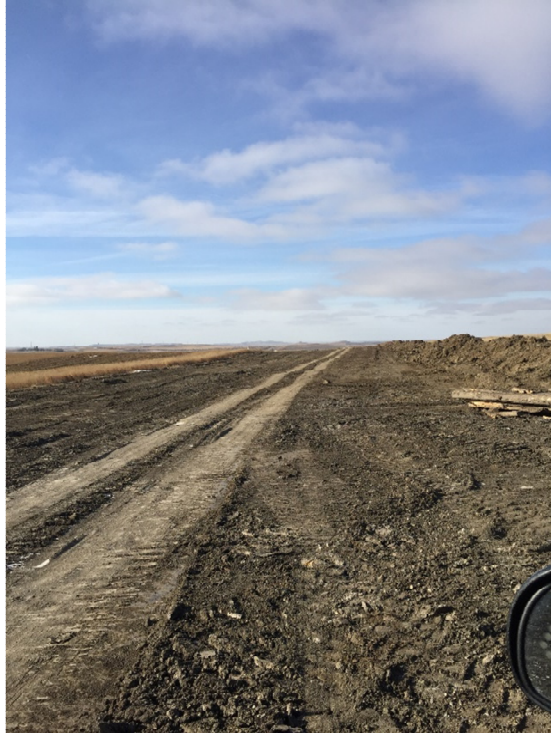
Picture 3: Grading completed prior to topsoil spreading
