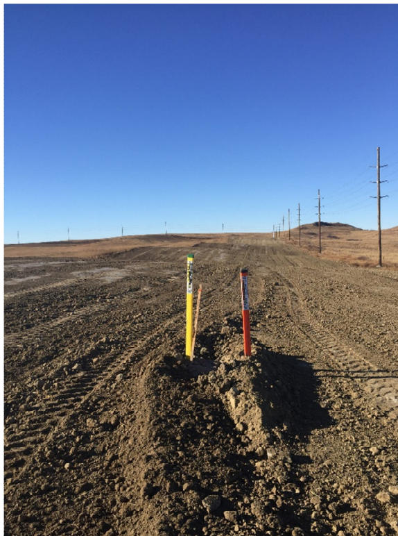
Picture 21: Topsoil spreading completed, looking west
