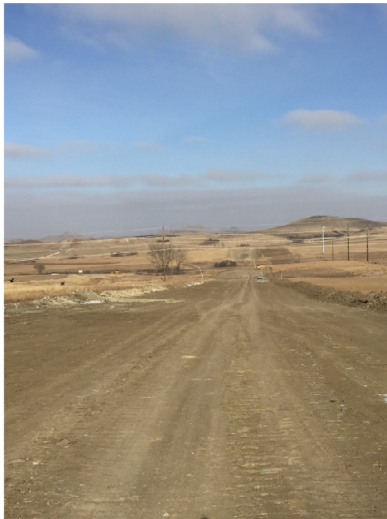
Picture 2: Finish grading subgrade, looking north
