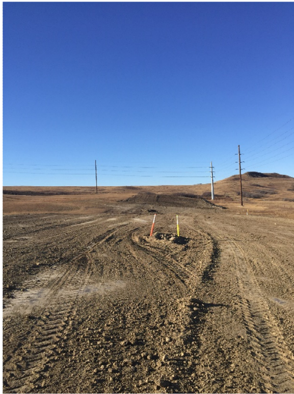
Picture 23: Topsoil spreading recently completed in background, looking west
