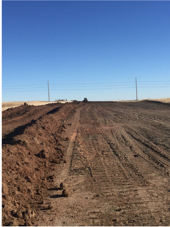
Picture 32: Begin spreading topsoil berm, looking east
