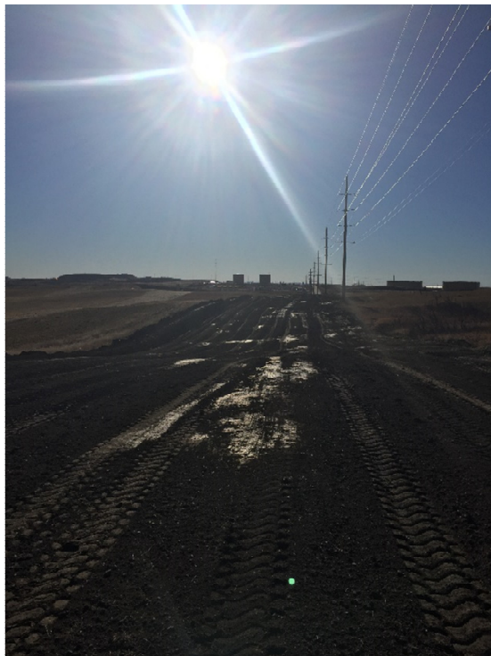
Picture 27: Topsoil spreading completed
