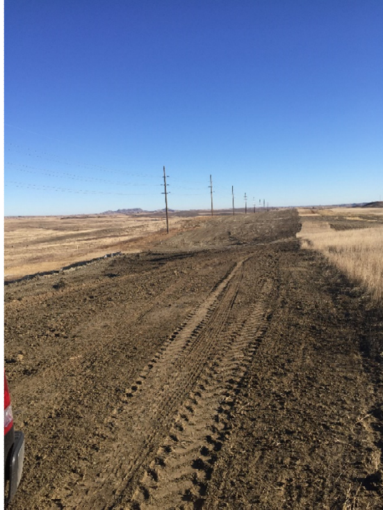
Picture 26: Topsoil spreading completed, looking east
