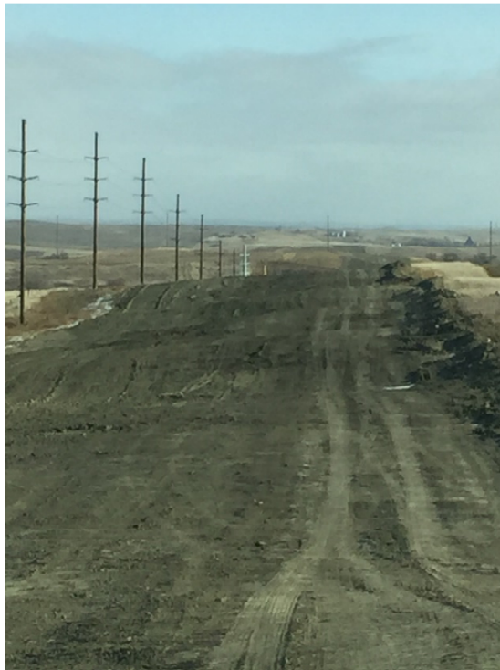
Picture 8: Grade restored to original contours prior to placing topsoil
