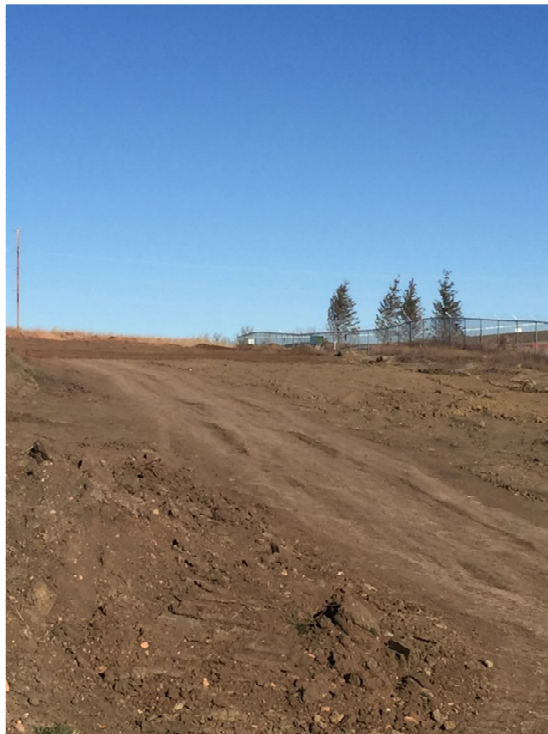
Picture 15: Topsoil spreading beginning near Johnsons Corner Terminal
