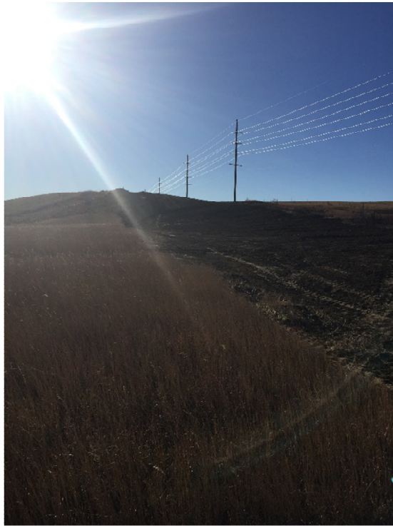
Picture 25: Topsoil spreading completed
