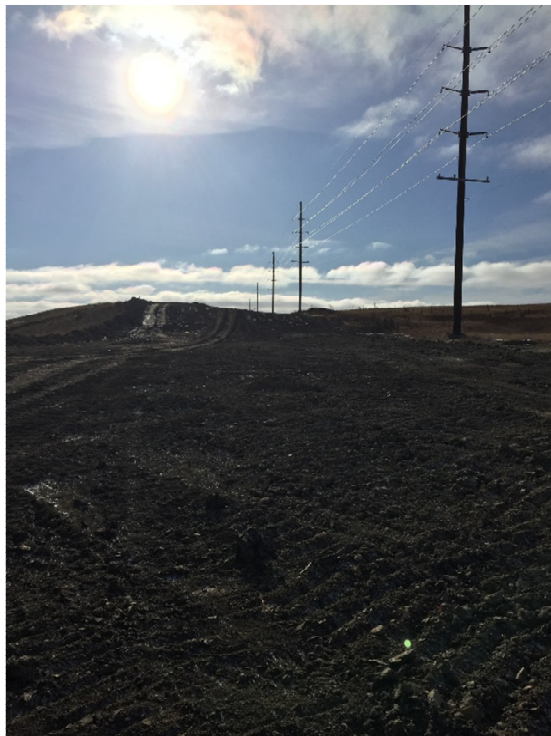
Picture 4: Grade returned to previous contours
