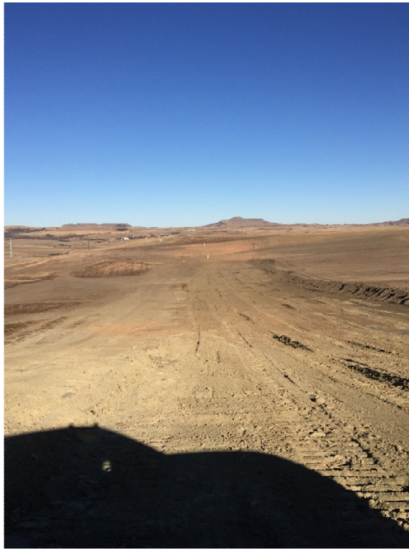
Picture 19: Grading in progress, looking north
