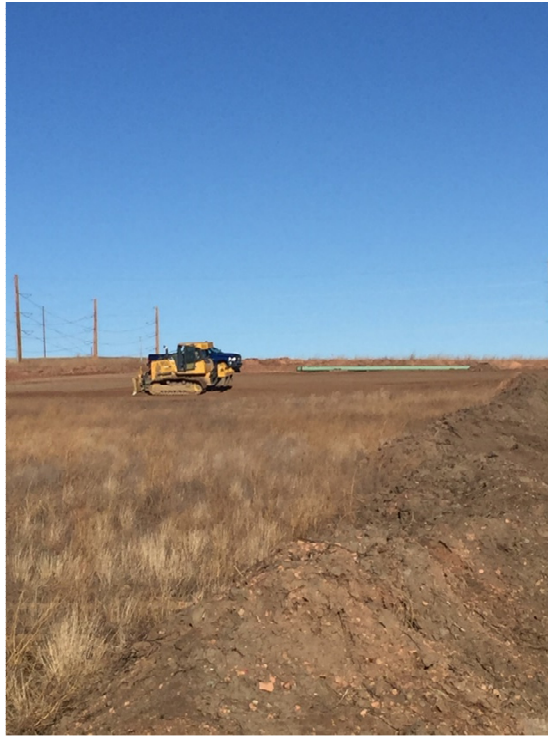
Picture 14: Equipment working on restoring grade
