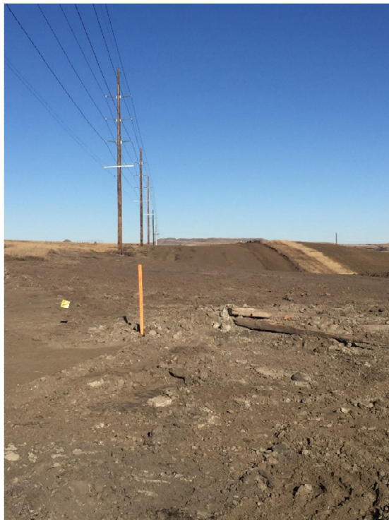
Picture 29: Grading and cleanup in progress
