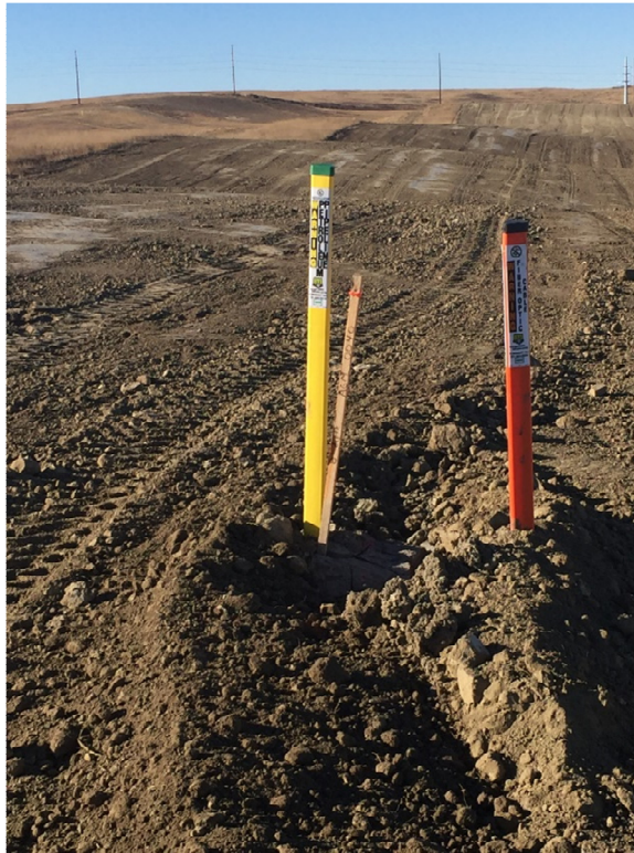
Picture 20: Topsoil completed, looking west
