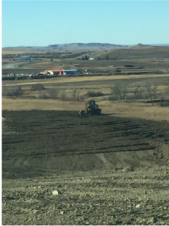
Picture 34: Finish grading of topsoil in progress, looking west
