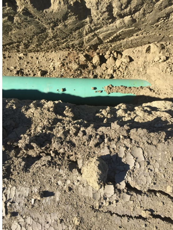
Picture 3: Pipe backfill
