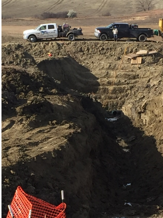
Picture 26: Excavating for trench near Highway 73 bore
