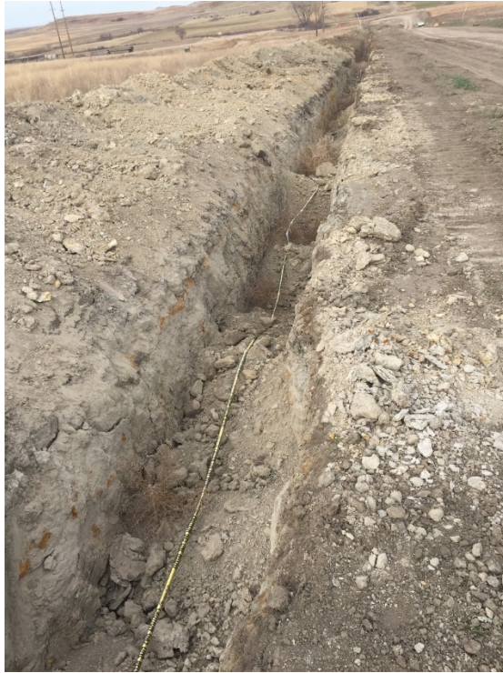
Picture 22: Backfill pipe trench, warning tape placed in trench
