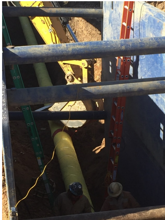
Picture 6: Trench box and installation of pipe at utility crossing
