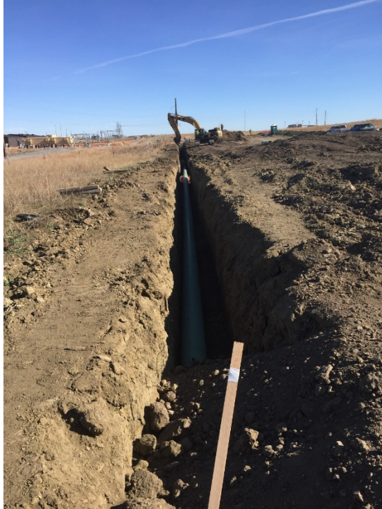
Picture 19: Backfill in progress
