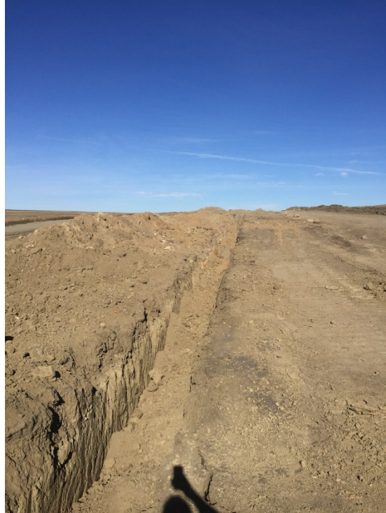
Picture 5: Backfilling pipe
