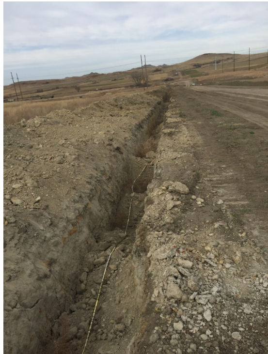
Picture 23: Backfilling, warning tape placed in trench
