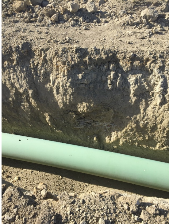
Picture 13: Pipe recently placed in trench
