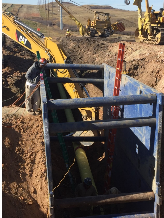
Picture 7: Utility crossing
