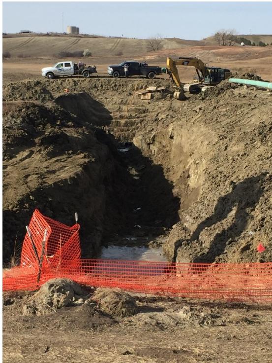
Picture 27: Excavating for trench near Highway 73 bore
