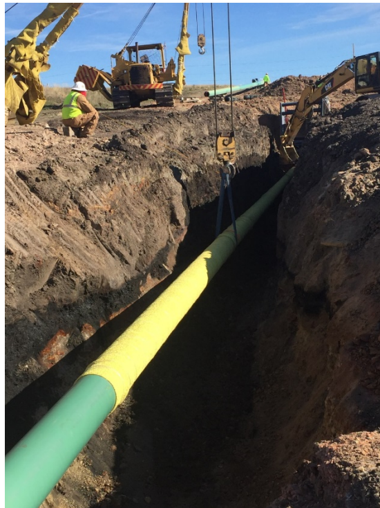
Picture 8: Placing pipe near utility crossing
