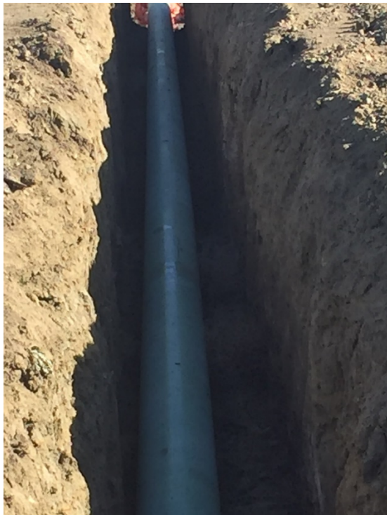
Picture 20: Backfill in progress
