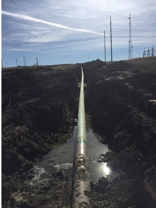
Picture 15: Pipe placed in trench, some water collecting in low area
