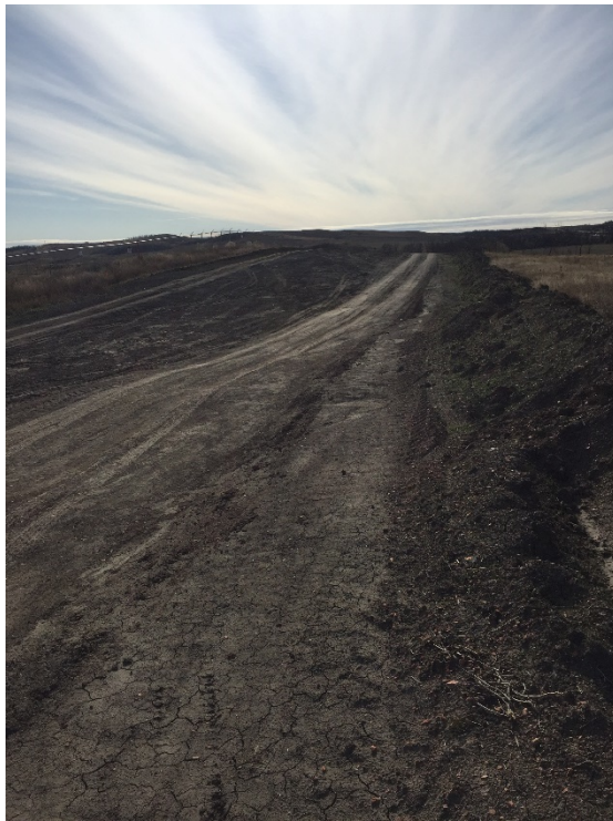
Picture 29: Backfill completed, prior to topsoil placement
