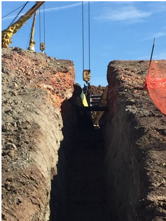
Picture 10: Installing pipe at utility crossing
