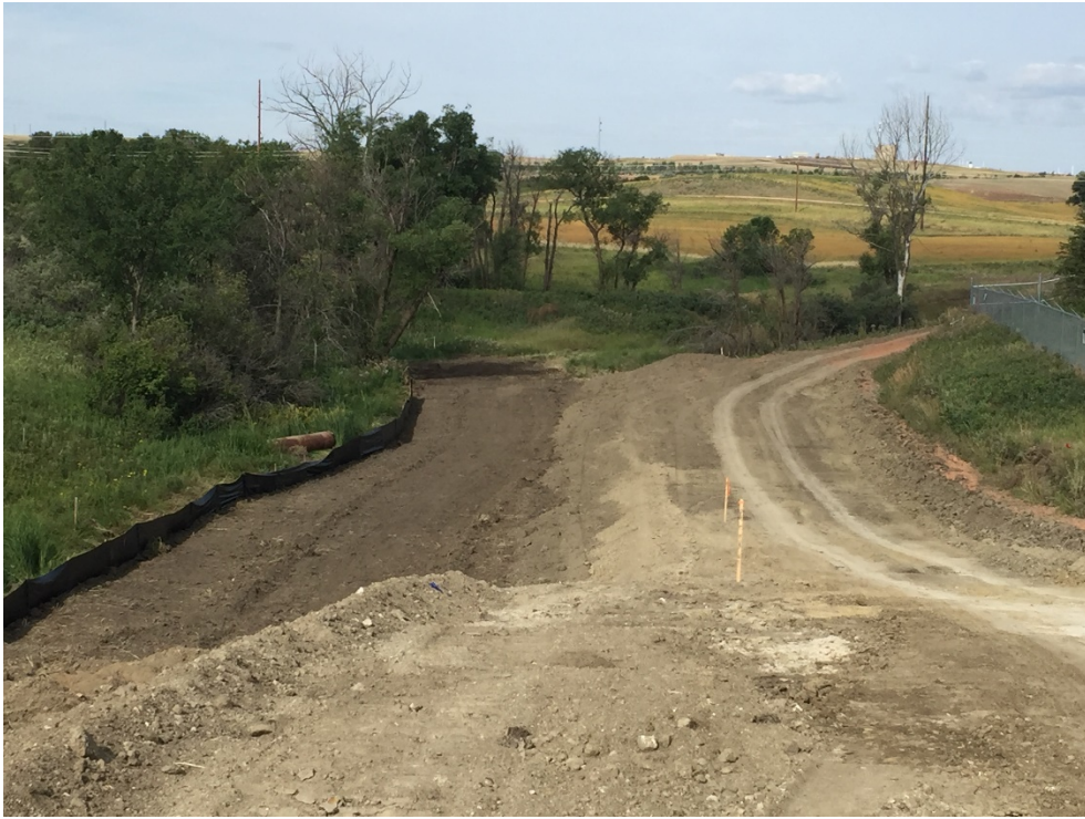
Photo 10: Sta. 7+00 looking west at the channel with topsoil removed to safe location and silt fence installed as previously committed to on site.
