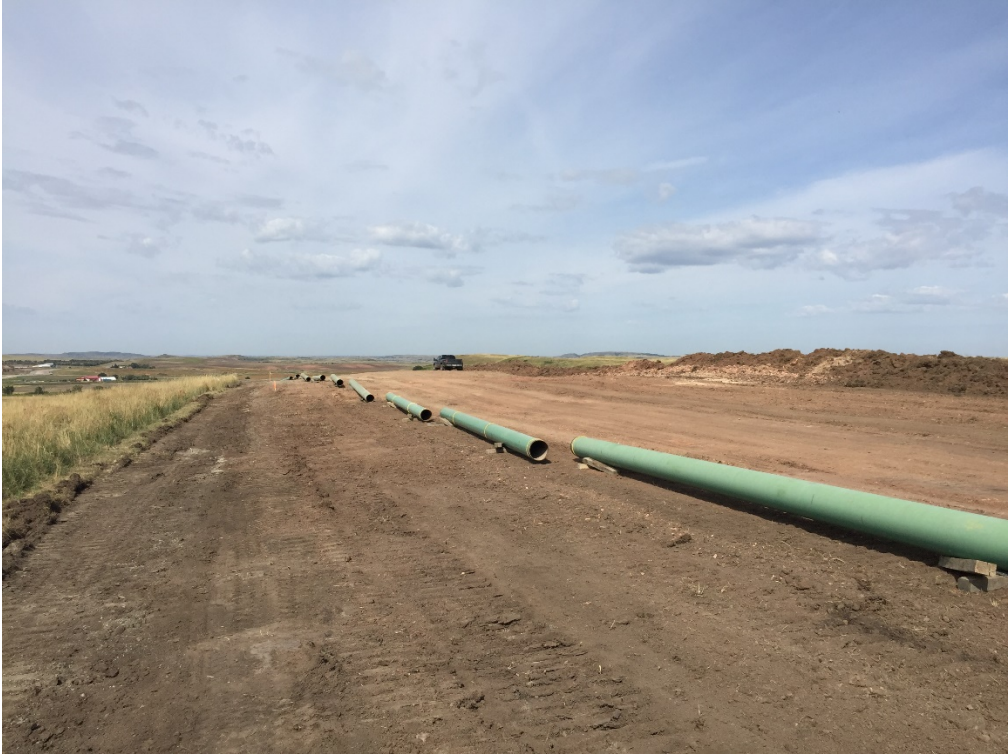
Photo 26: Sta. 130+00 looking west.
