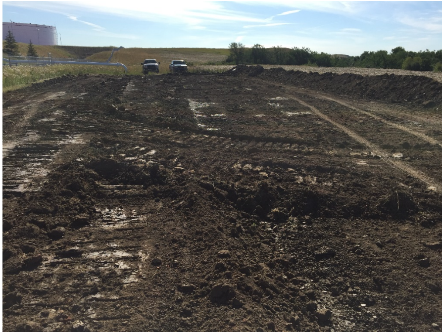
Photo 1: Sta. 3+00 looking east to start of project at 0+00
