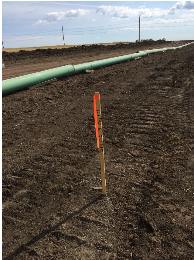
Photo 25: Sta. 128+00 pipe staged, preparing to weld.
