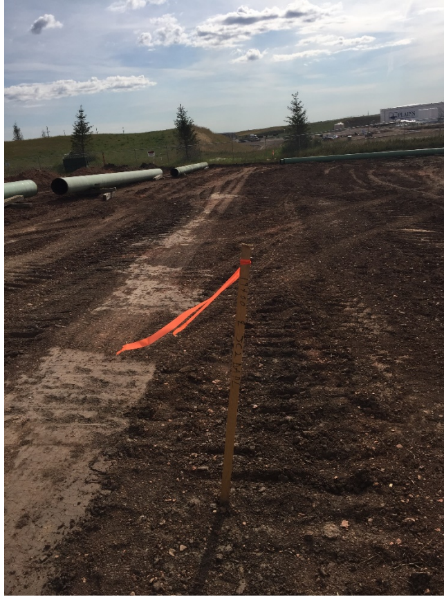
Photo 12: Sta. 19+00 looking east, pipe being delivered.
