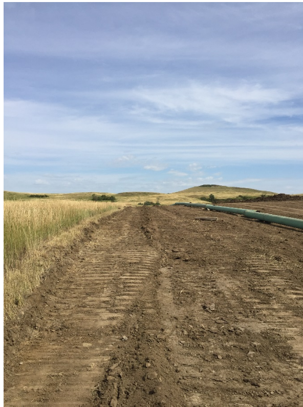
Photo 31: Sta. 146+00 looking north.
