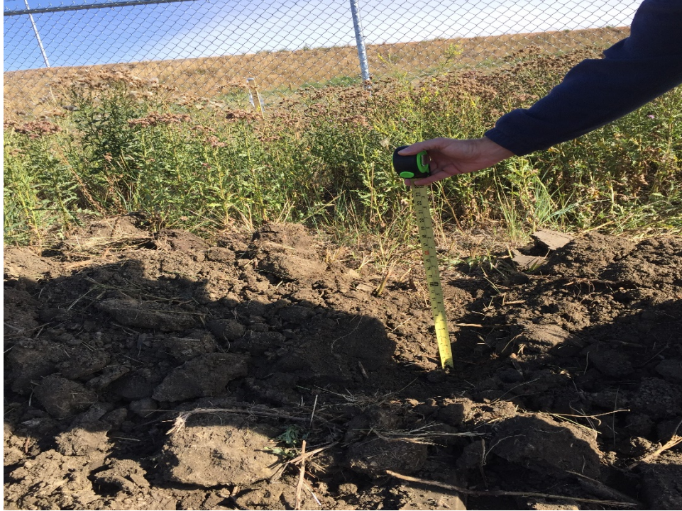
Photo 3: Sta. 3+00 showing 8 inches topsoil removal
