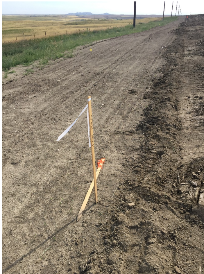
Photo 14: Sta. 92+00 showing back side of topsoil pile along R/W. The previous pipe installation is visible to the north or left with no vegetation.
