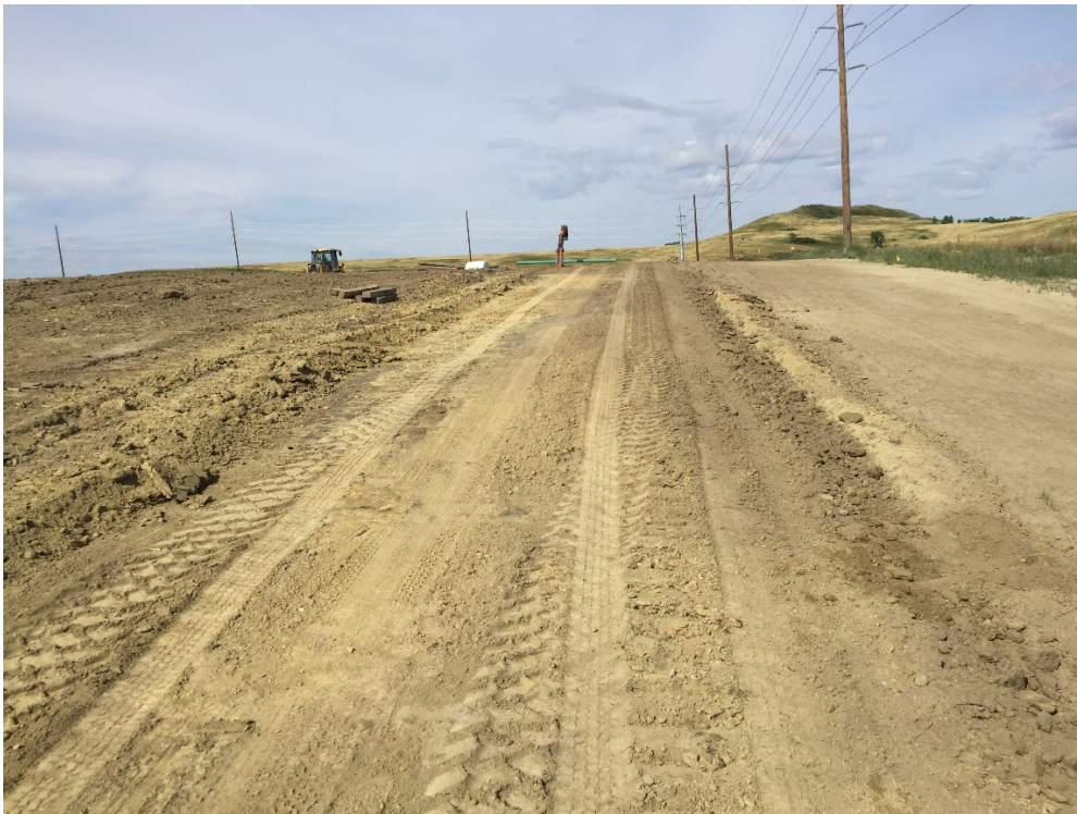
Photo 19: Facing west, Sta. 100+00. Area to right is previously installed pipeline. Area on the left side is the current project.
