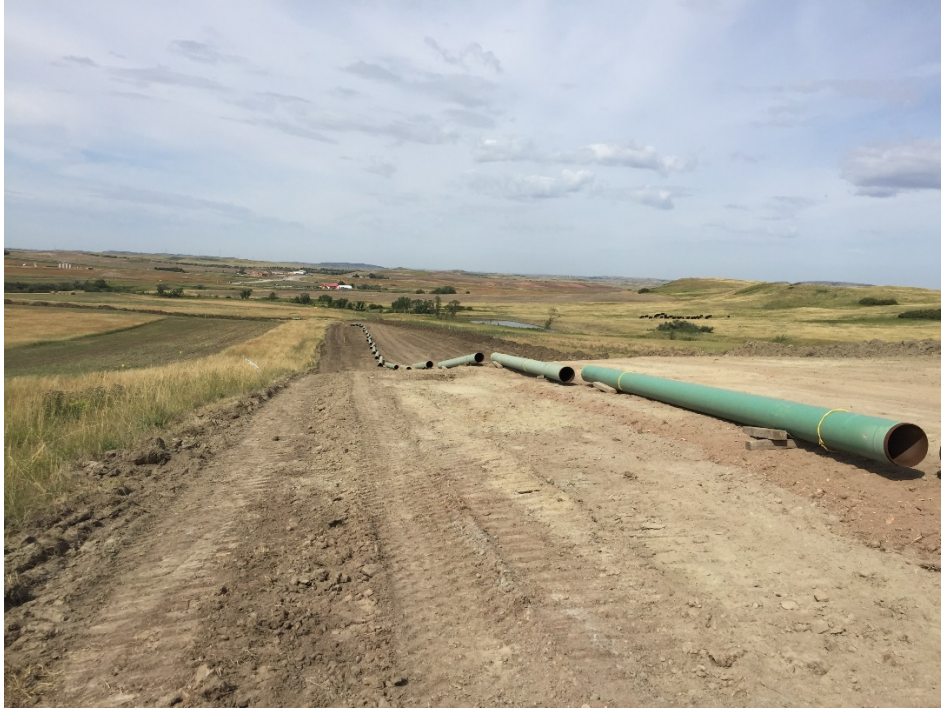
Photo 28: Sta. 142+00 Looking west.
