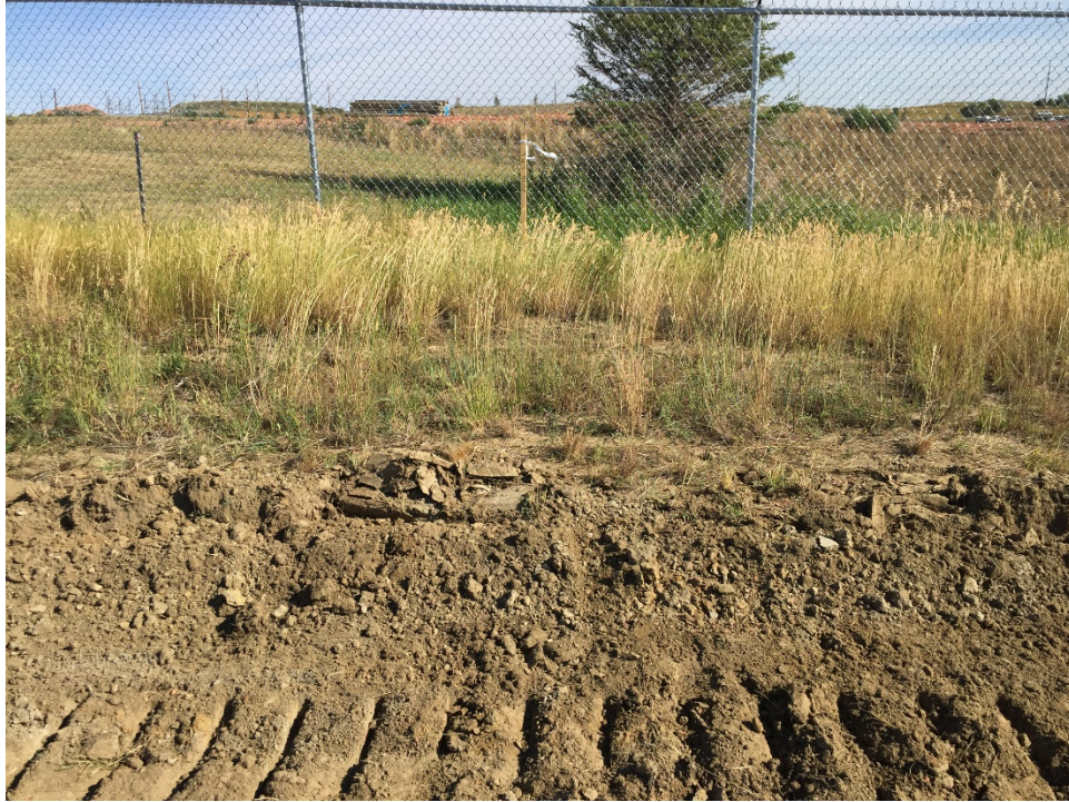
Photo 5: Sta. 4+00 showing top soil removal depth
