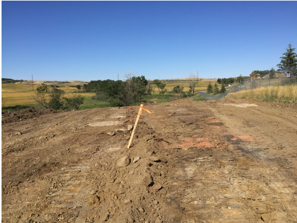
Photo 4: Sta. 4+00 looking west
