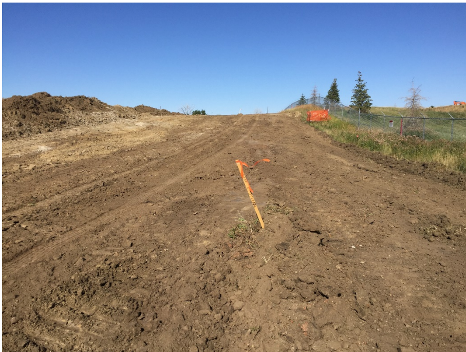
Photo 2: Sta. 3+00 looking west
