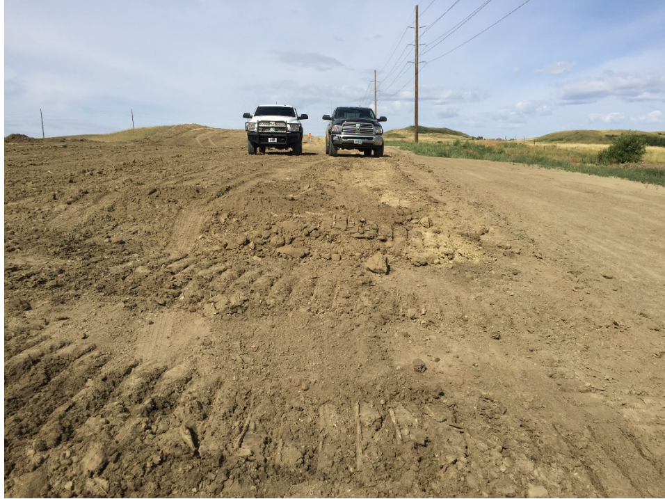
Photo 16: Sta. 92+00 looking west
