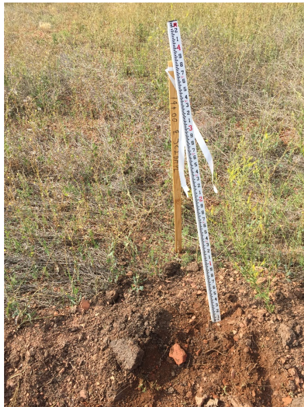
Photo 11: Sta. 14+00, 7 inches topsoil removed.
