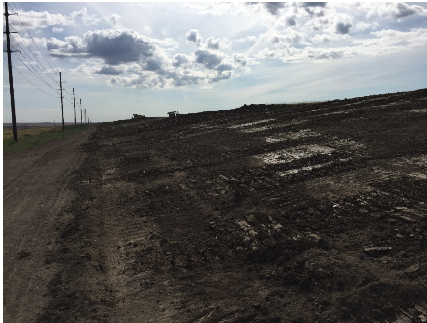
Photo 15: Sta. 92+00 looking east.
