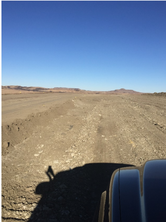
Picture 18: Grading in progress, looking north. Beginning to spread topsoil from berm
