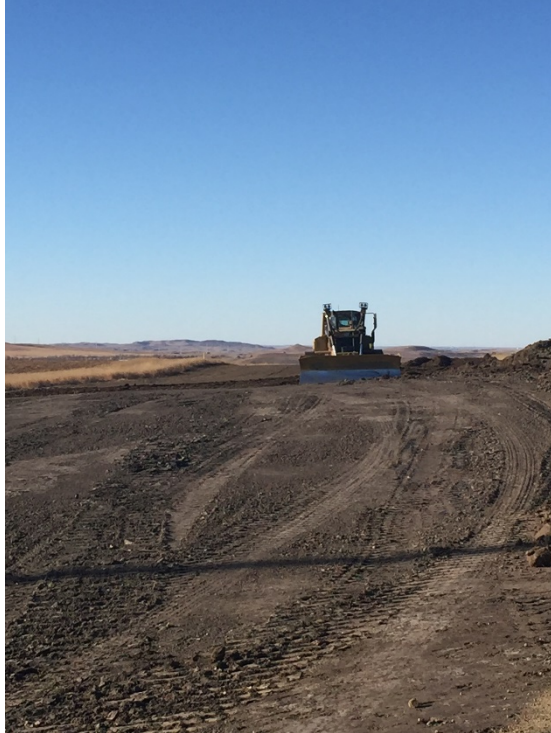
Picture 30: Topsoil spreading in progress, looking west
