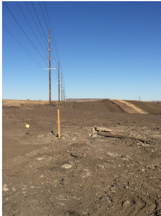
Picture 29: Grading and cleanup in progress
