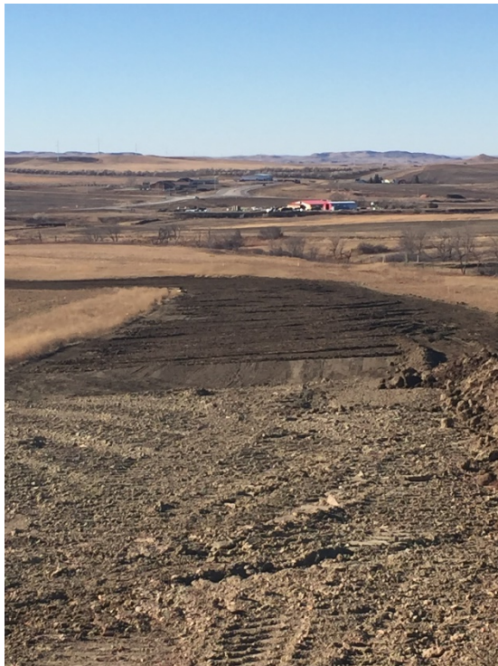
Picture 33: Topsoil spreading completed, looking west
