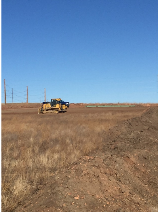
Picture 14: Equipment working on restoring grade
