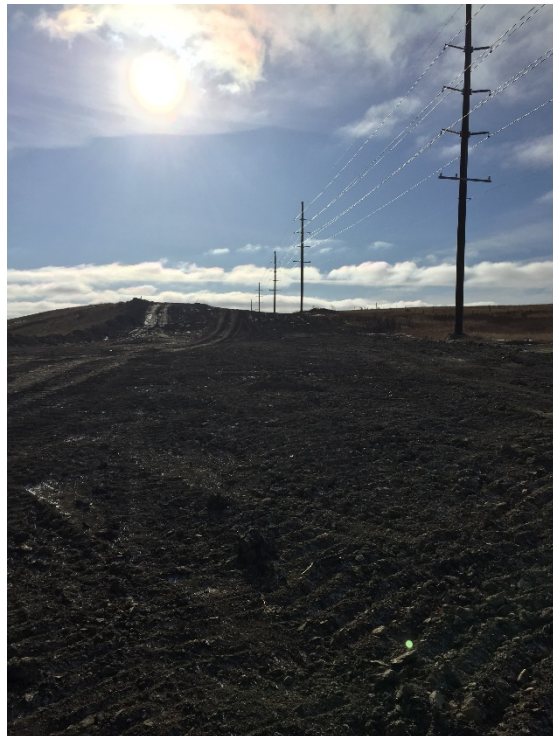
Picture 4: Grade returned to previous contours
