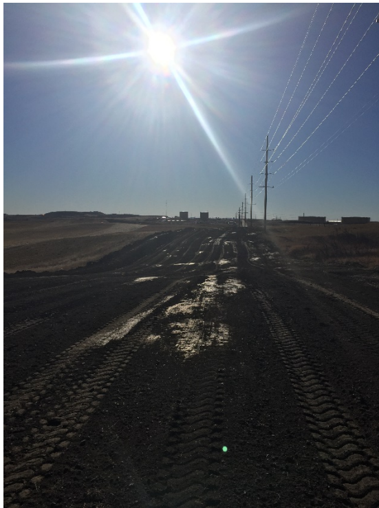
Picture 27: Topsoil spreading completed
