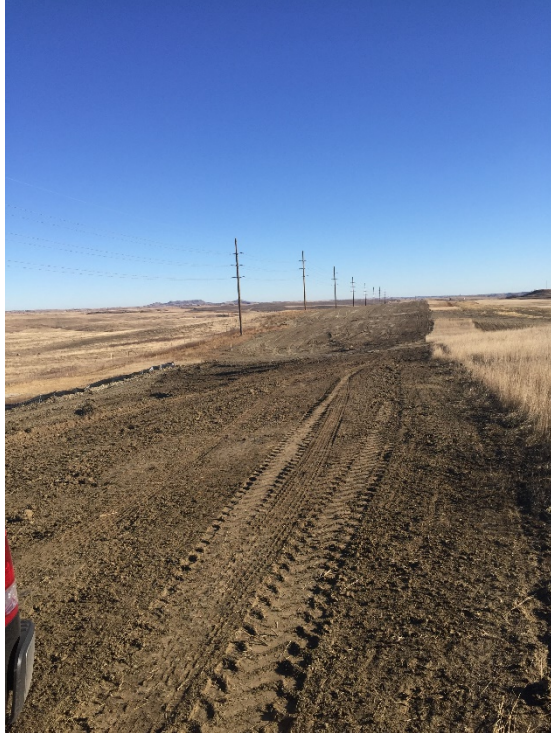
Picture 26: Topsoil spreading completed, looking east
