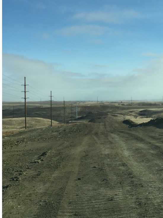
Picture 11: Ready for topsoil to be spread, showing grade returned to existing contours
