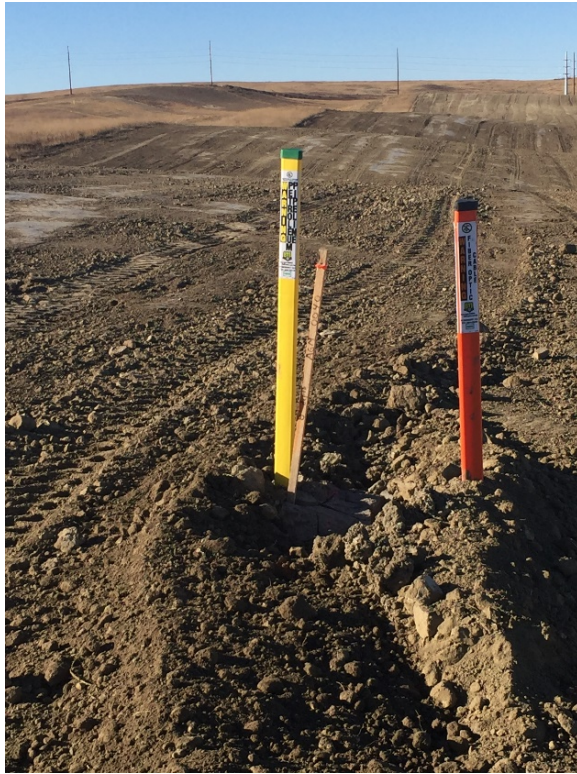
Picture 20: Topsoil completed, looking west
