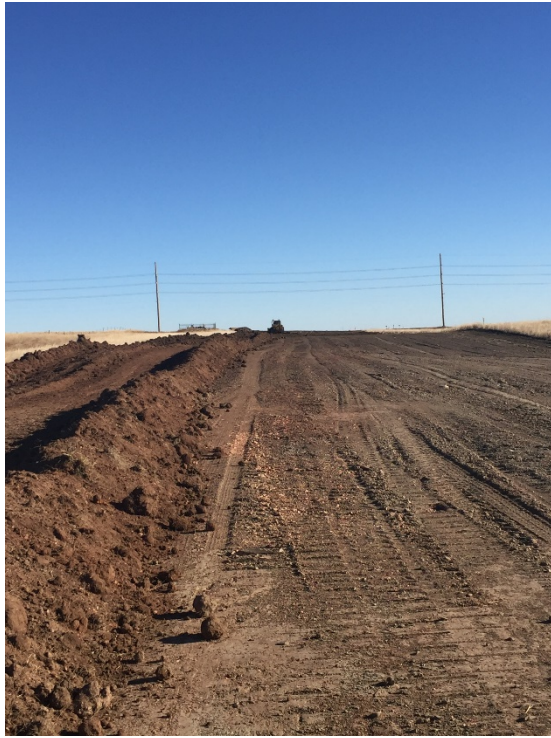
Picture 32: Begin spreading topsoil berm, looking east
