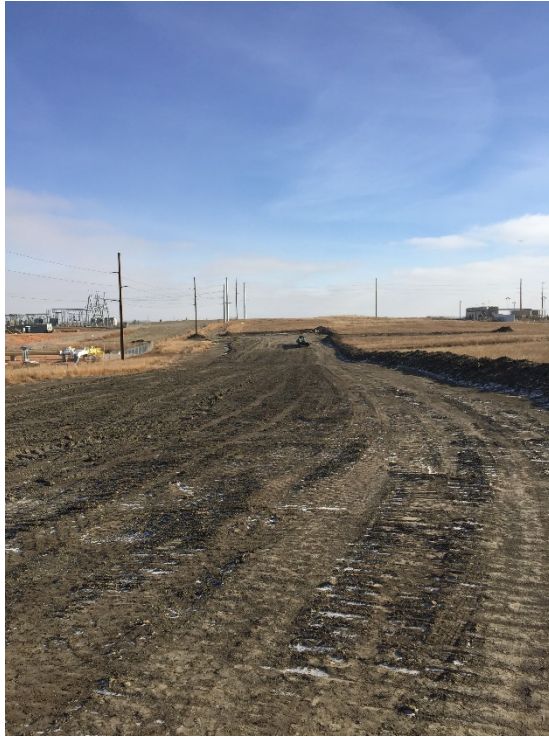
Picture 1: Finish grading, some topsoil remaining to be spread
