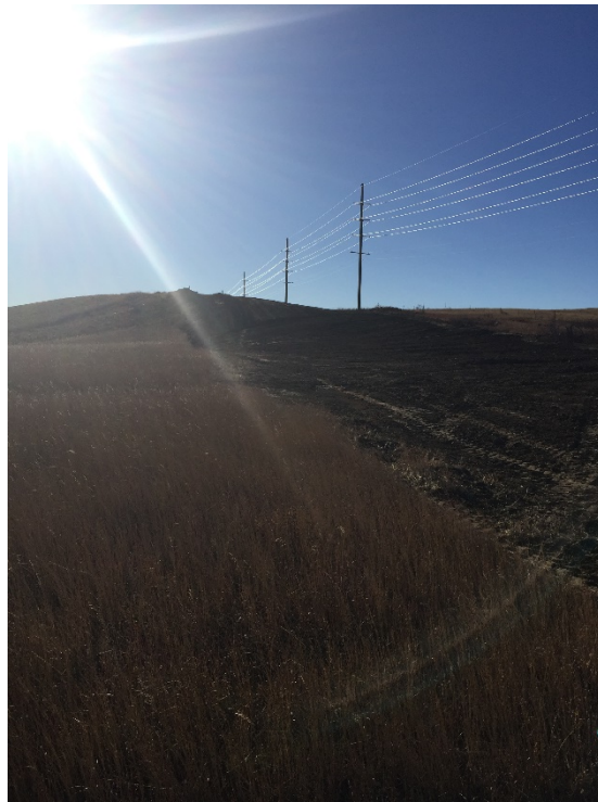
Picture 25: Topsoil spreading completed
