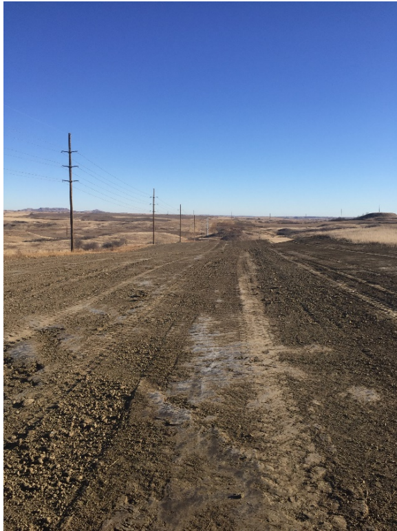
Picture 22: Topsoil spreading completed, looking east
