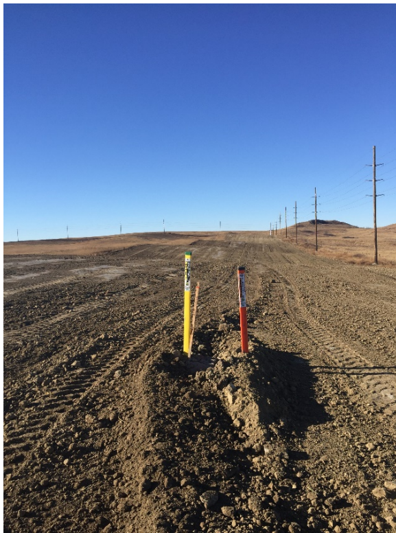
Picture 21: Topsoil spreading completed, looking west
