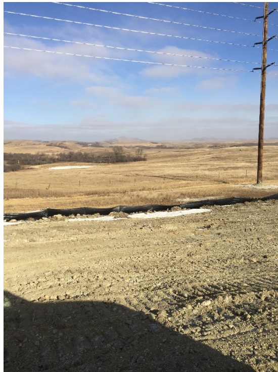
Picture 6: Silt fence at drainage area, finish grading completed
