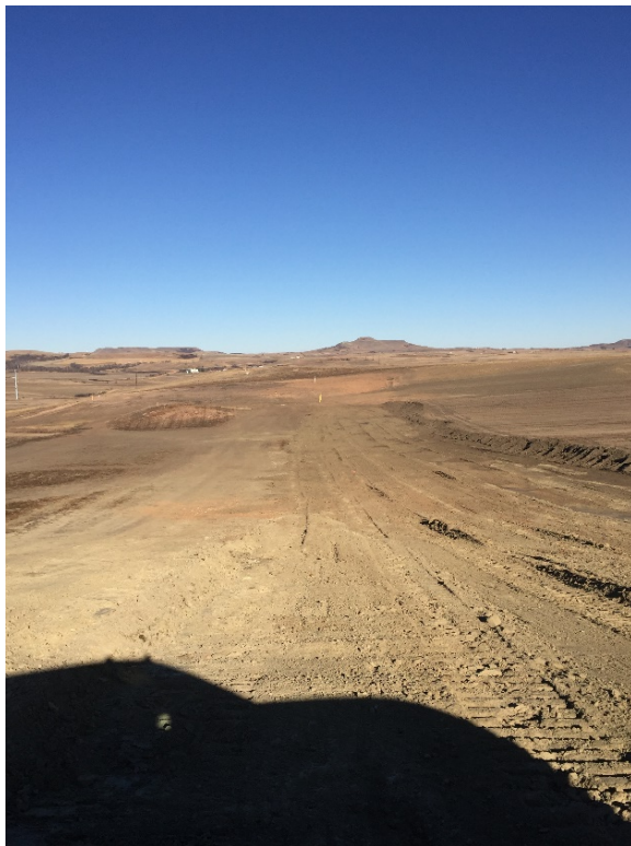
Picture 19: Grading in progress, looking north
