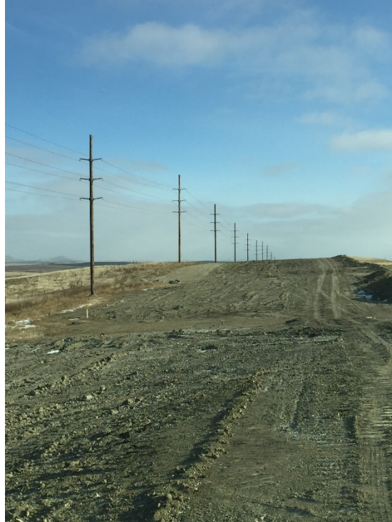
Picture 5: Low area to be graded before topsoil is spread, looking east
