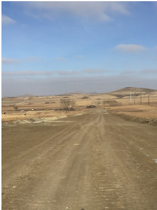
Picture 2: Finish grading subgrade, looking north
