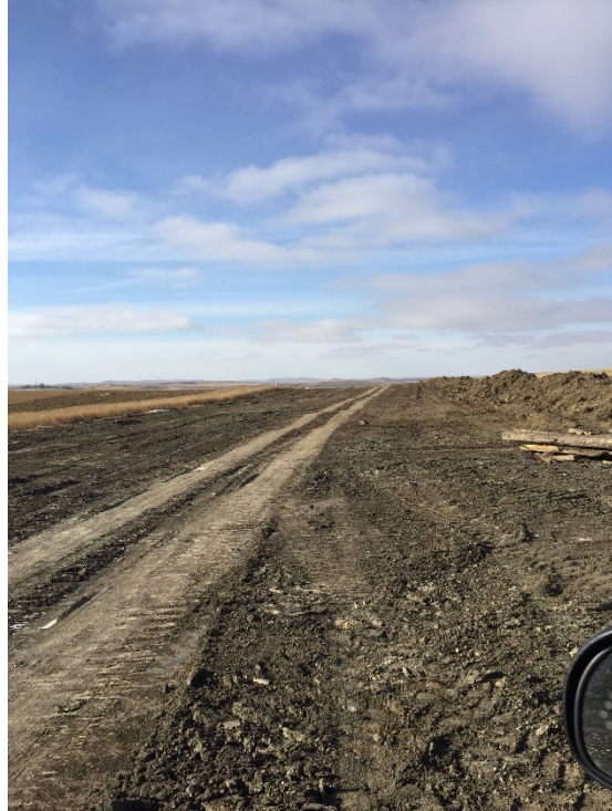
Picture 3: Grading completed prior to topsoil spreading
