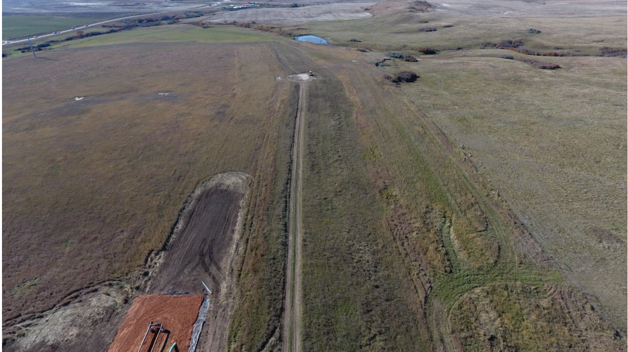
Location 23 - Looking west, vegetation well established, and blending into surrounding conditions
