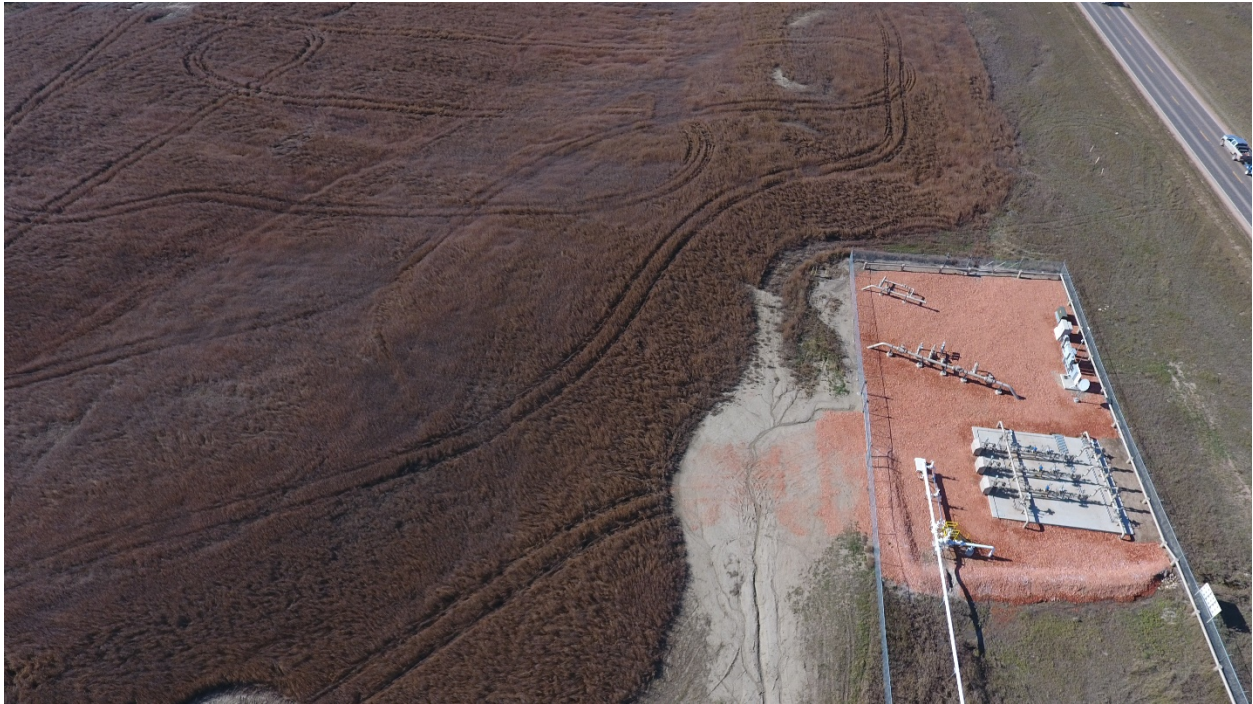
Location 9 - Looking west. Pipeline not detectable in farmland
