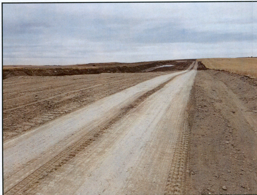
Figure 5. View looking east down the pipeline corridor.
