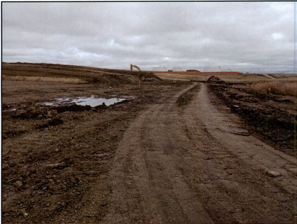
Figure 4. Photo taken looking northeast. Pipeline has been installed and backfilled.
