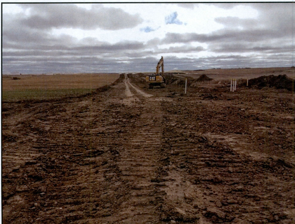
Figure 5. View looking south down the pipeline corridor.
