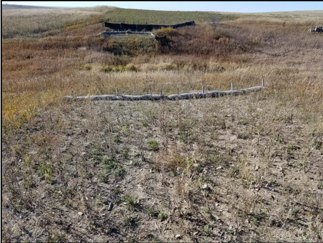
Figure 4. Photo taken looking west at the wetland/waterbody crossing. Vegetation is poorly established with noxious weeds present.
