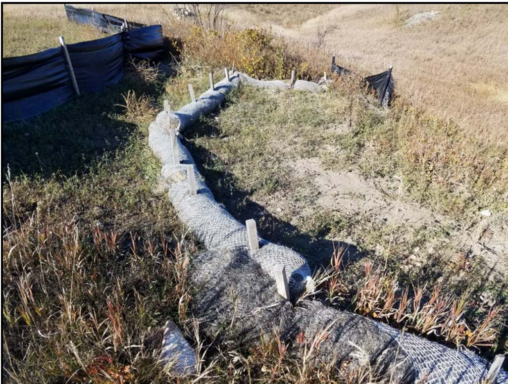
Figure 5. View of ECD's in place and functioning on the west side of the wetland/waterbody crossing.
