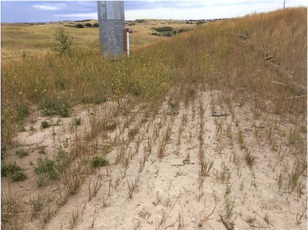
Structure 298-133, View West – July 27, 2017
