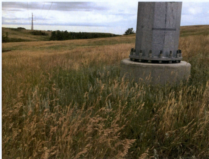
Structure 298-132, View East – July 27, 2017
