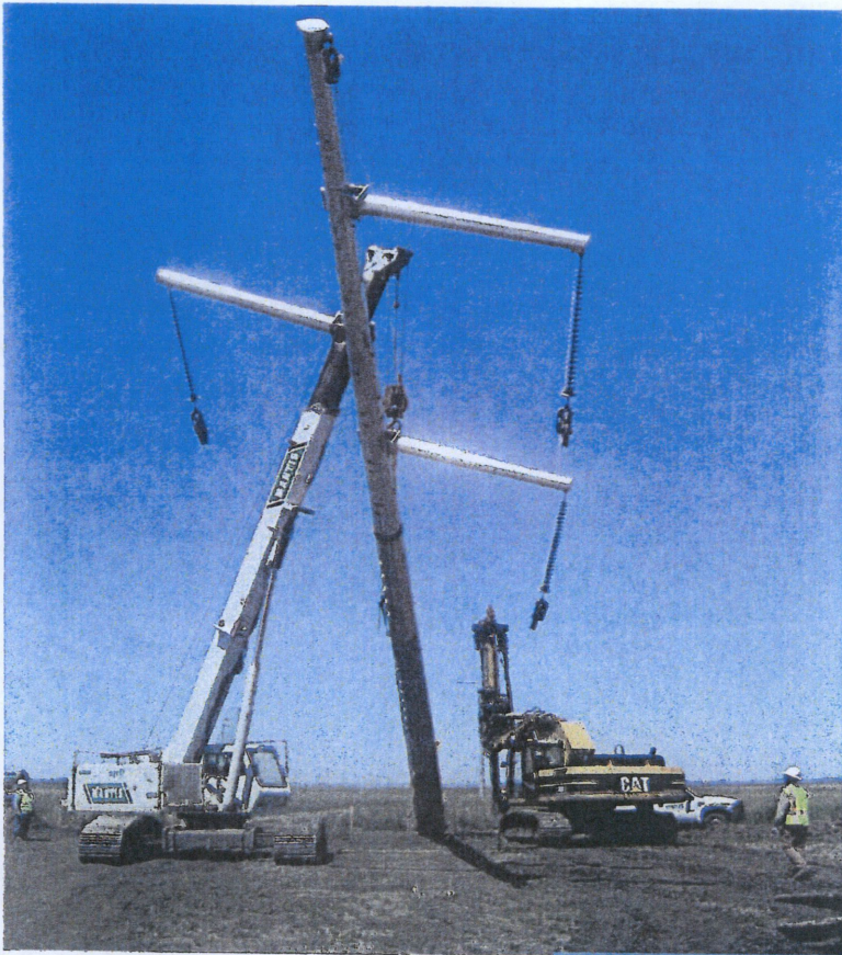
Structures are lifted into place and 'set' on the foundations
