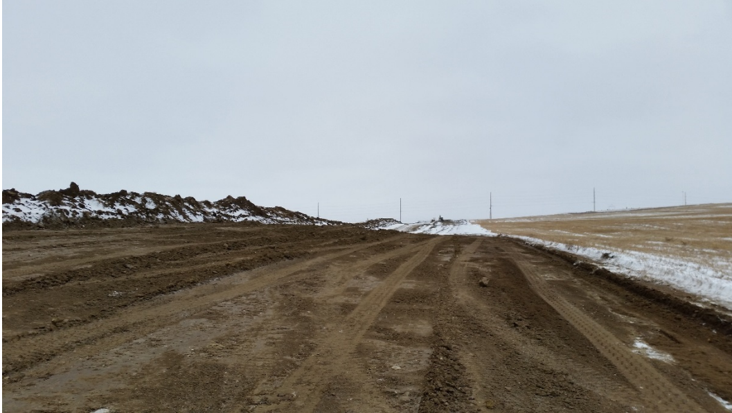
Above: Photo 11 (pt. 2) – Pipe has been buried. Topsoil to the left. Direction: South.
