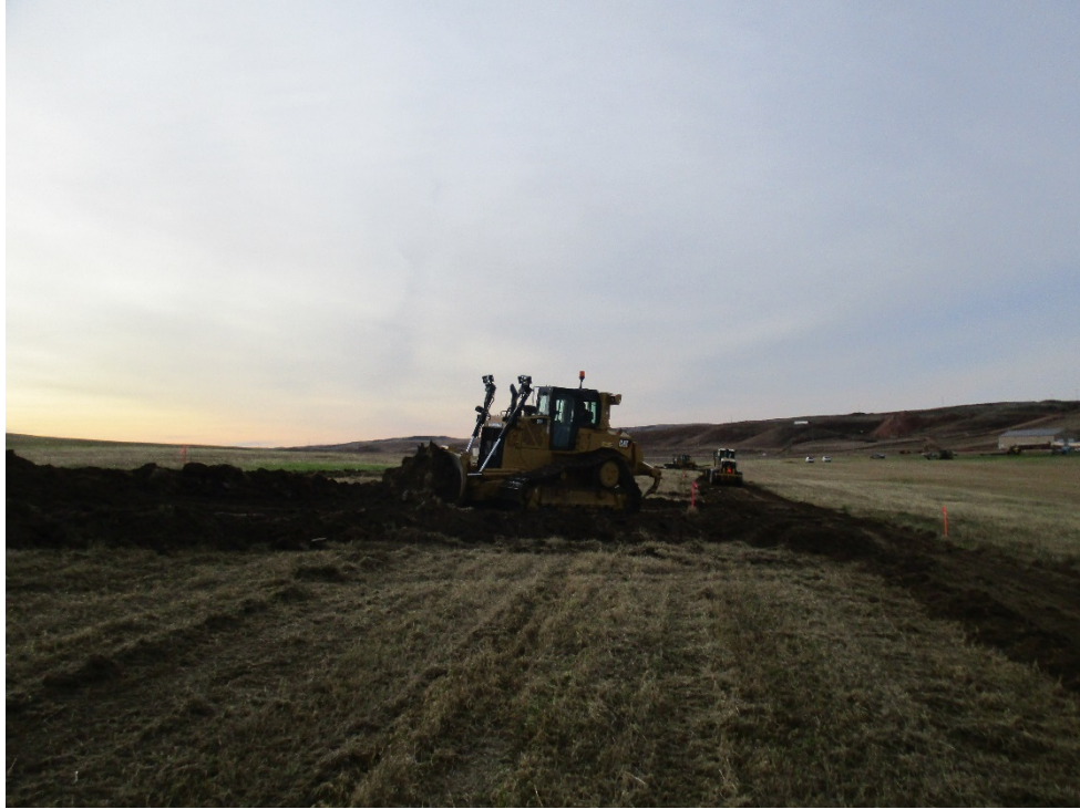
Above: Photo 3 (pt. 491) – Topsoil is being stripped. Direction: South.
