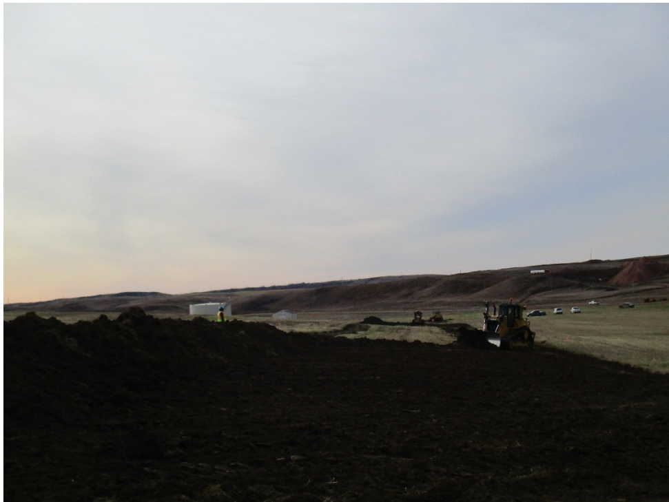
Below: Photo 2 (Point 491) – Start of topsoil stripping. A spotter (to the left of photo) was used to help the dozer operator make sure the topsoil pile was staying within the ROW. Direction: South.
