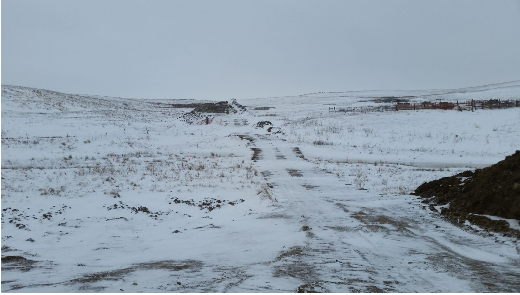
Above: Photo 15 (near pt. 3) – Drainage/creek area. Mats through creek area. Topsoil on the right side of the ROW. Direction: West-northwest.
