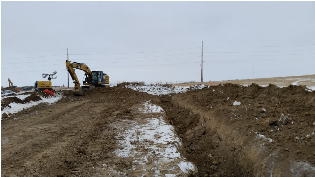
Below: Photo 12 (near pt. 1, north of the road) – Track hoe is covering up the trench (replacing subsoil). Direction: South.
