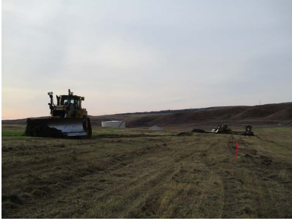
Above: Photo 1 (Point 491) – Start of topsoil stripping. The dozer and grader are marking the edge of the ROW. Another dozer is in the background stripping topsoil. Direction: South.
