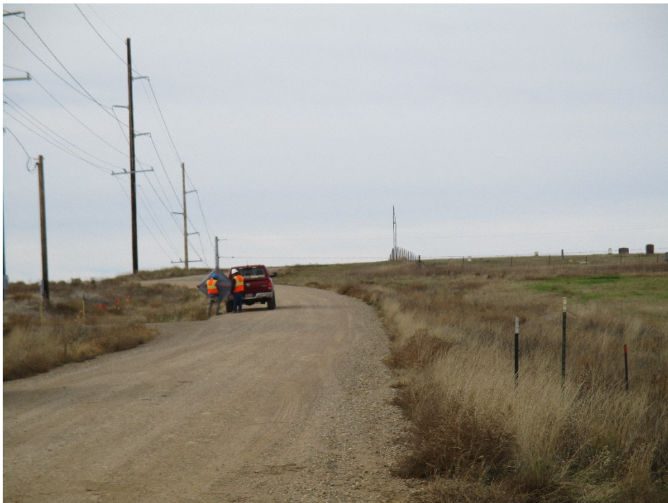
Below: Photo 8 (pt. 493) – Crew installing warning signs for construction area.
