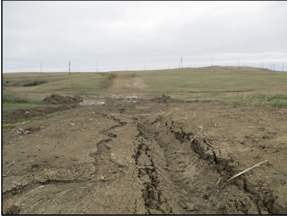
Photo 5. (Near GPS Point #510) – There is soil subsidence along the trench and some erosion forming near it. This is leading to a wetland area that was double ditched. Direction: East.
