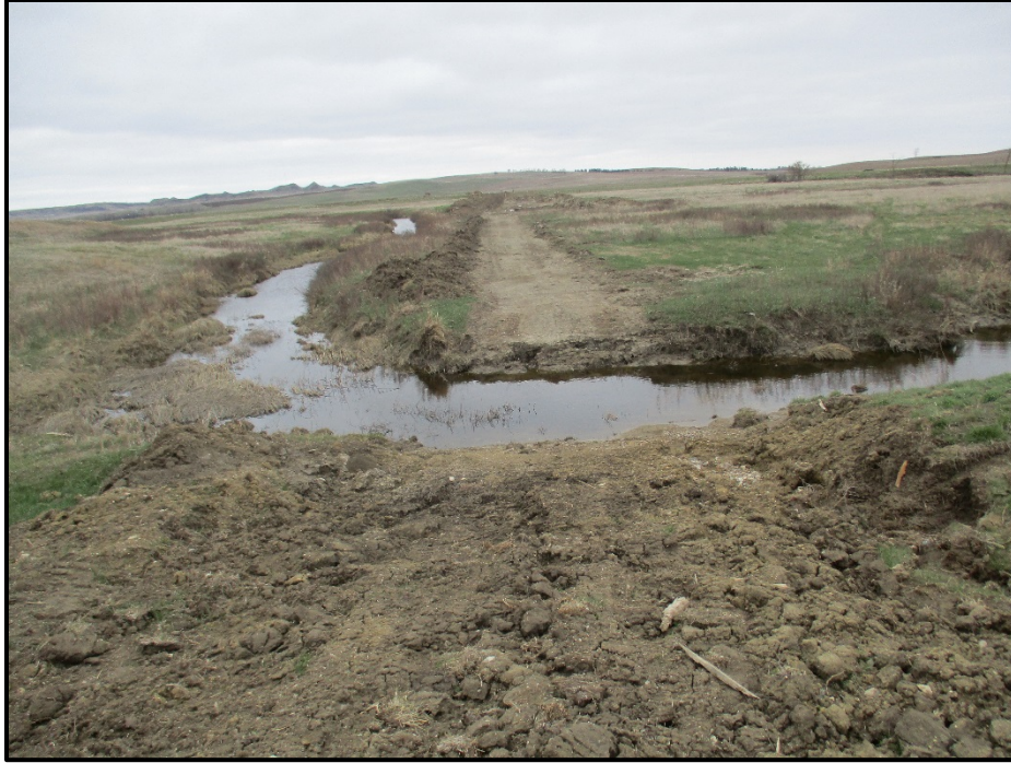
Photo 15. (GPS Point #517) – The stream crossing along the ROW was bored. There were mats along this area which were used by vehicles to cross the stream, but they have since been removed. Direction: Southwest.
