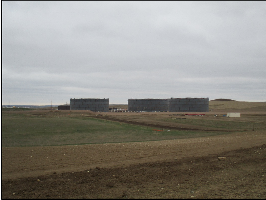
Photo 13. (GPS Point #513) – View shows northern portion of the pipeline where it connects to DAPL. Direction: Northwest.
