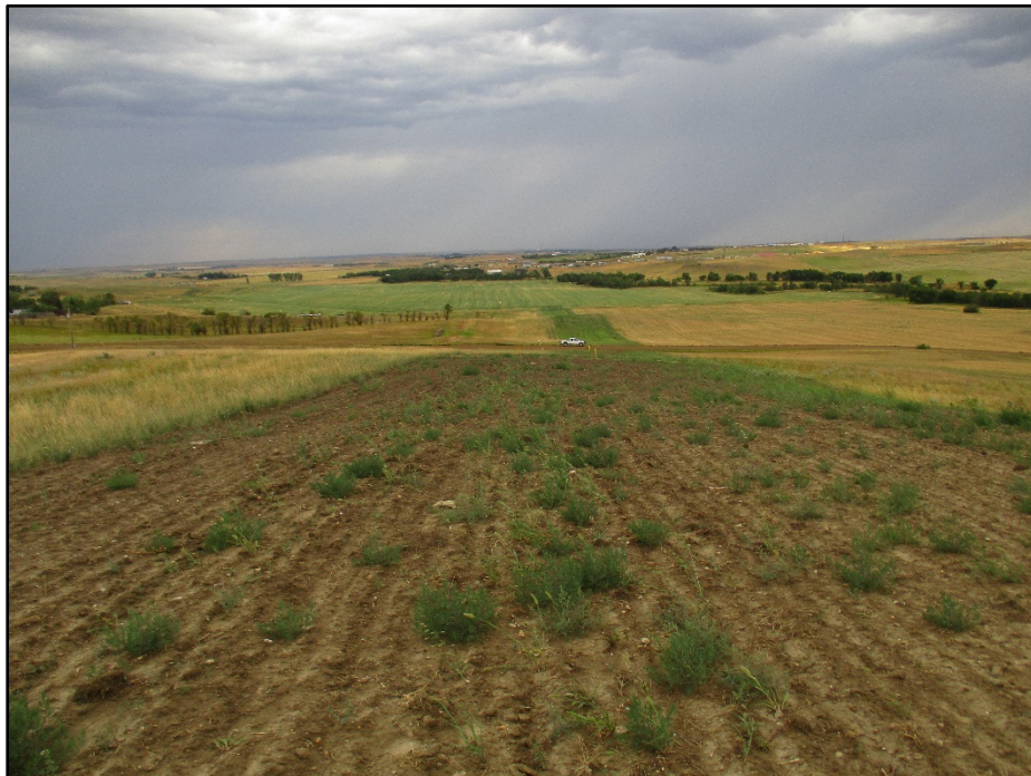
Photo 10. (GPS Point #528) – Pipeline ROW with bare ground, mostly annual weeds growing and few grasses. Vegetation growth from re-seeding was poor most likely due to drought conditions. Direction: North.
