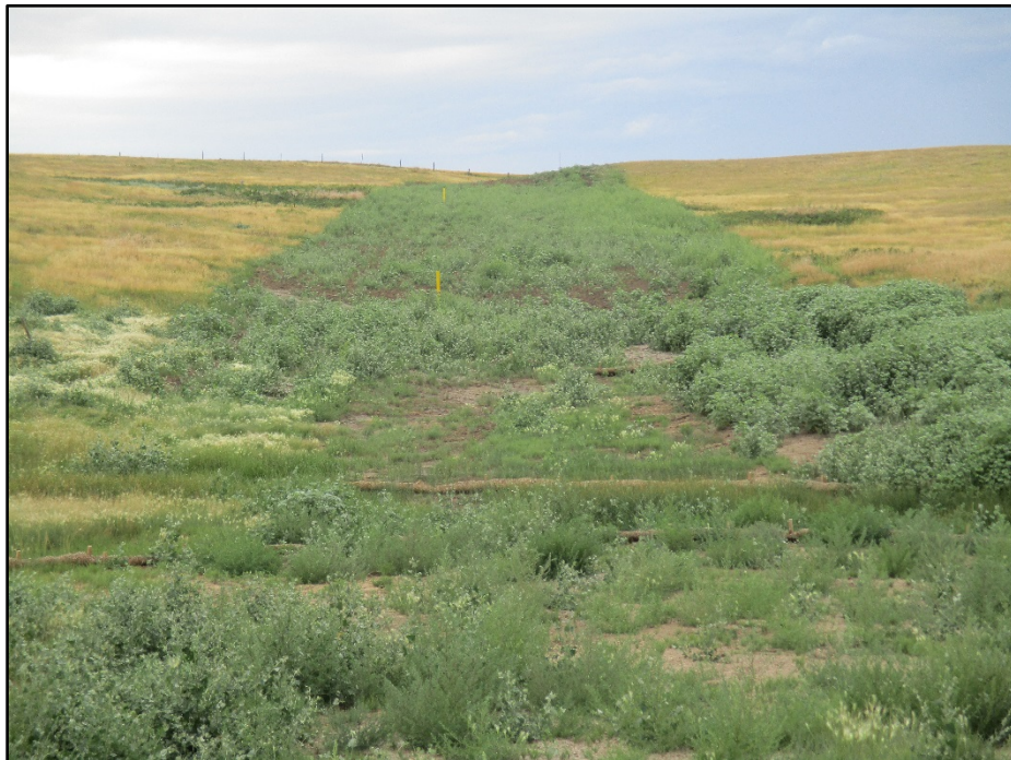
Photo 12. (GPS Point #529) – View of wetland area that was double ditched. Width of pipeline disturbance was necked down to cross wetland. Straw wattles were observed. Pipeline markers are along the ROW. Direction: West.
