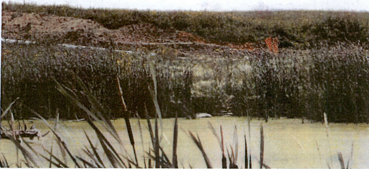
The next two photos, taken at a location east of 87 th Avenue on an unnamed road in Mountrail County, show an area where silt fence was installed but then evidently run over and neglected.
