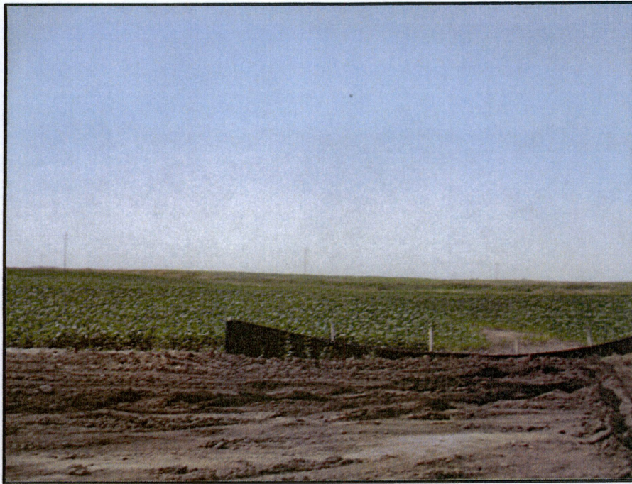
Photo 7. (GPS Point #448) - Silt fence observed in drainage area near crop field, which needs maintenance. The area was rutted up and needs to be smoothed out again. Topsoil had been replaced back on the ROW.
