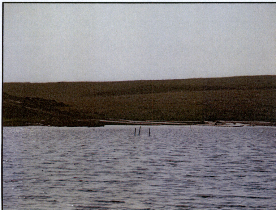
Photo 20. (GPS Point #483) - Swamp mats floating in wetland. Dirt pile in water seen to left of photo on wetland edge. No erosion control devices observed. Direction: South
