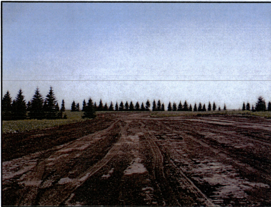
Photo 6. (GPS Point #448) – ROW necked down to 50 ft width through tree rows. Unknown if or how many trees were taken out in this area. Topsoil replaced back on the ROW. Direction: East.
