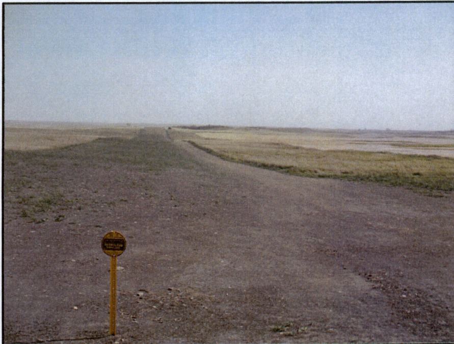
Photo 24. (GPS Point #490) - Pipeline ROW has vegetation growing. Looks like the right side of the ROW, where no vegetation is growing, has been/or is being used as a travel lane. Direction: East
