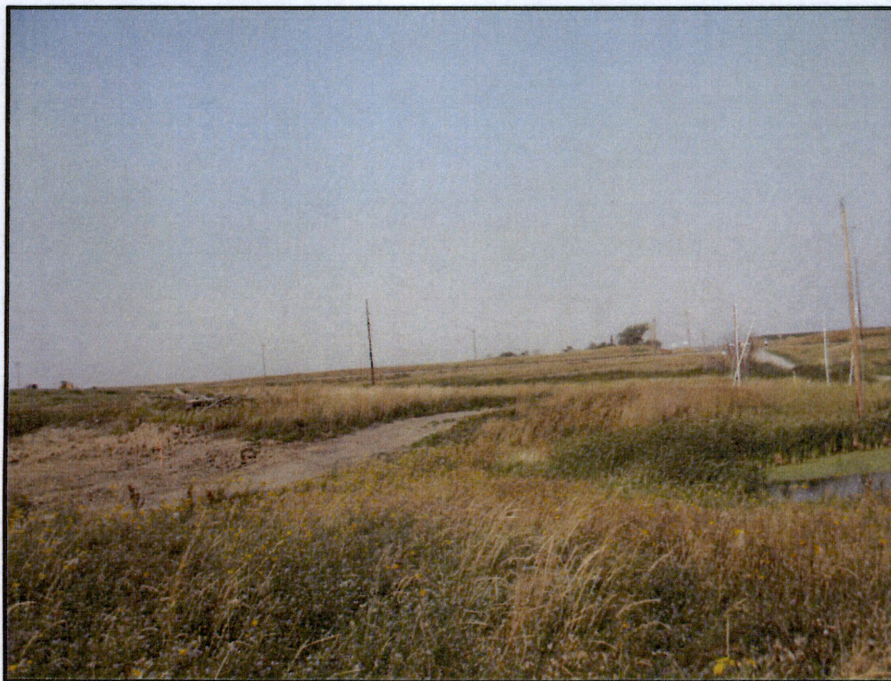
Photo 16. (GPS Point #481) - ROW and access road next to wetland. No erosion control devices observed. Site visit 9/1/2016. Direction: West
