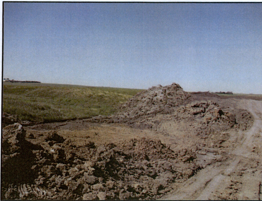
Photo 3. (GPS Point #446) - Drainage area along ROW, which appeared to be a potential wetland based on the topography, moist soil (along ROW edge) and change in vegetation. Topsoil pile along the left of photo. Drainage area looks like a potential wetland area.
