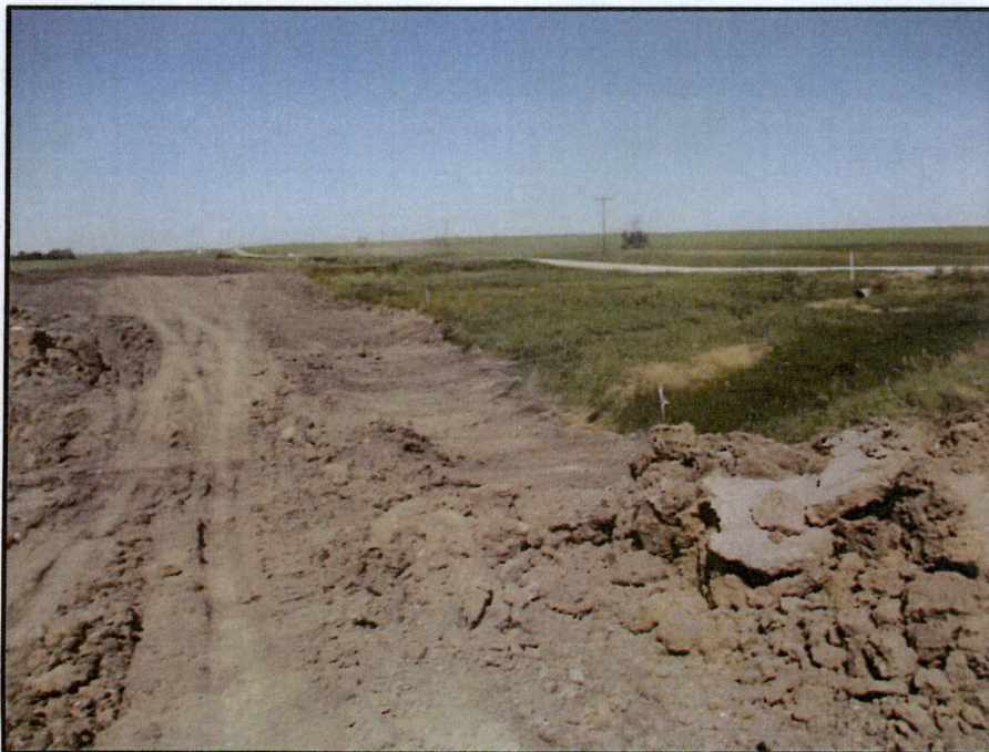
Photo 4. (GPS Point #446) - Drainage area intersected by ROW. Pipe trenched and backfilled along the edge of the ROW. The drainage area appeared to be a potential wetland. Notice the vegetation change. However, the environmental inspector stated it was not a wetland. No erosion control devices were observed. The PSC was informed of this site the day after the inspection.
