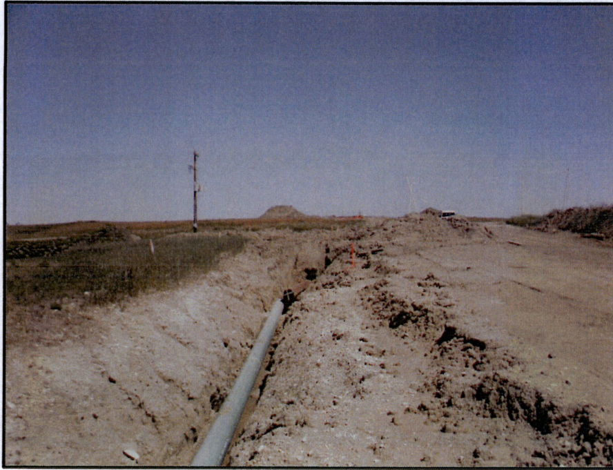
Photo 13. (GPS Point #444) - Area near rural water line break. Open trench to the left of photo. No standing safety fence observed. Environmental inspector thought they hit the rural water line while they were doing boring activities. Direction: North
