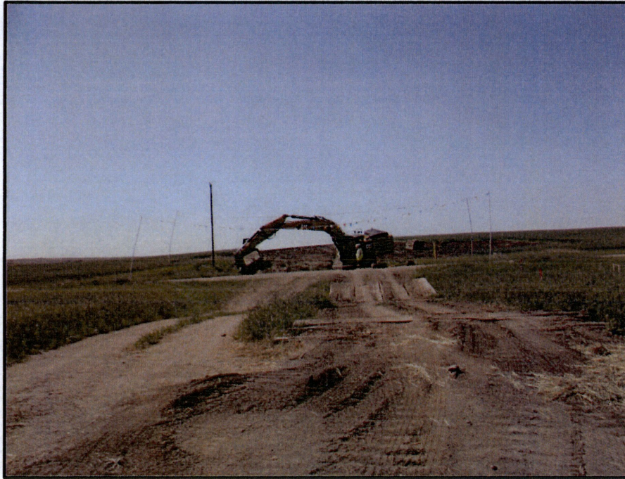
Photo 5. (GPS Point #447) – Excavator removing mats from road ditch (far side of the road), which was used for access to the ROW. Most of the topsoil had been replaced in this area. Direction: South
