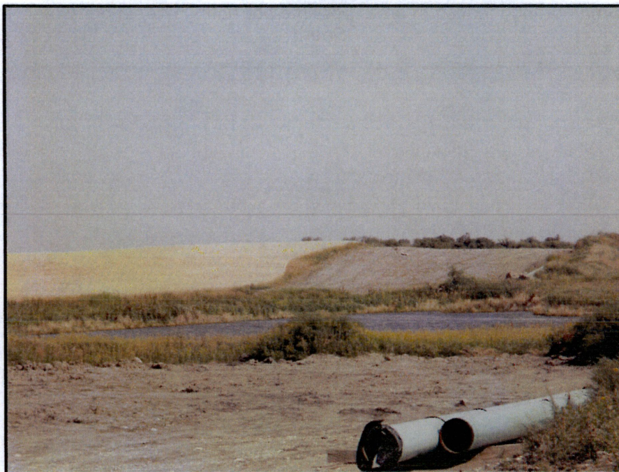
Photo 22. (GPS Point #485) - Pipeline ROW goes down the hill in the distance and wetland was bored under. No erosion control devices observed. Direction: North
