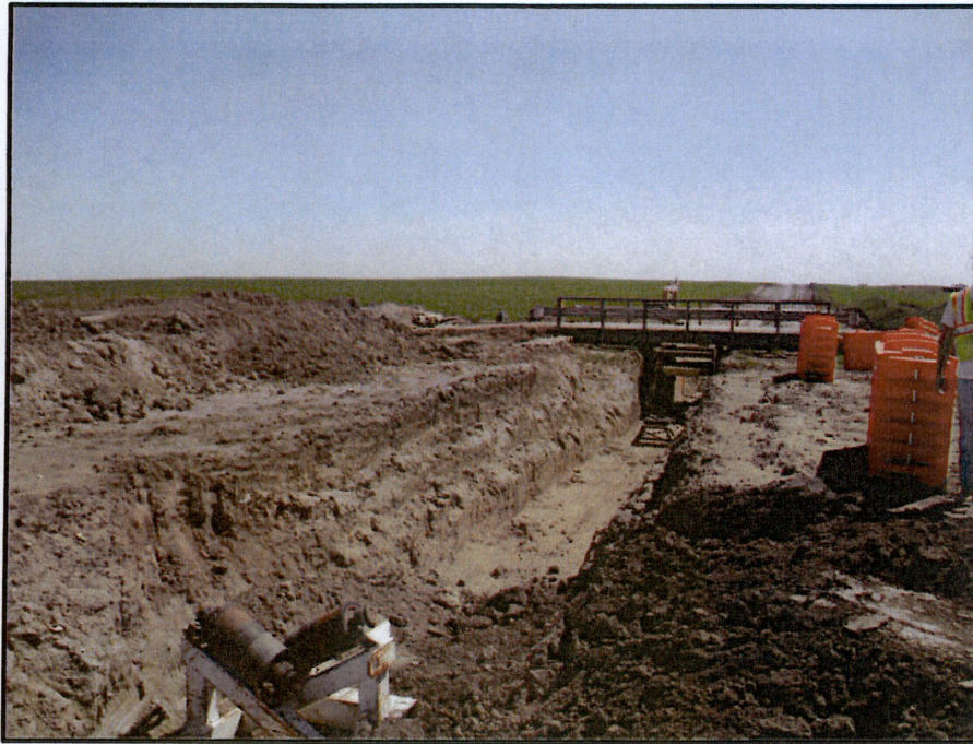
Photo 11. (GPS Point #450) - Open trench with orange blockades to the right of photo, trench spoil to the left. White and black pipe rollers in foreground were used to guide bore pipe. Bridge was used for a vehicle crossing to get to the bore area. Direction: East
