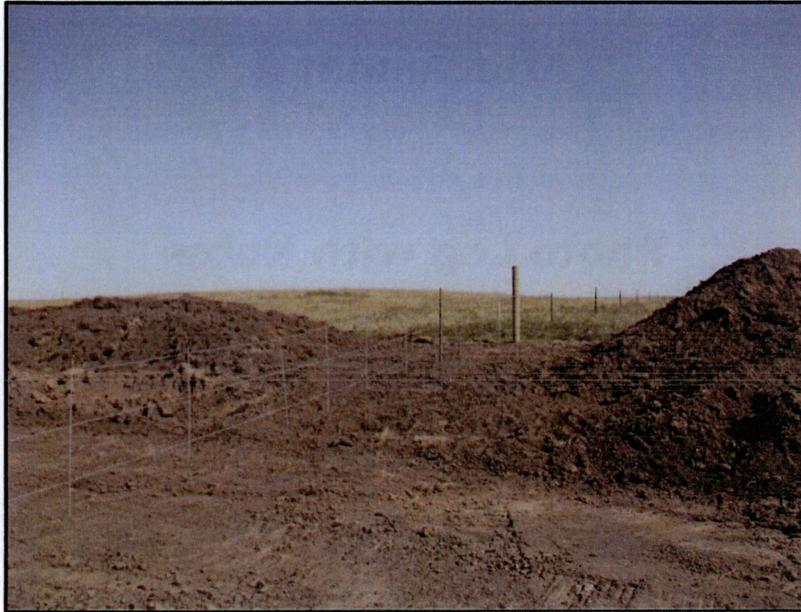
Photo 1. (GPS Point #443) – Temporary gate for fence put up across the ROW. Site visit 7/21/2016.
