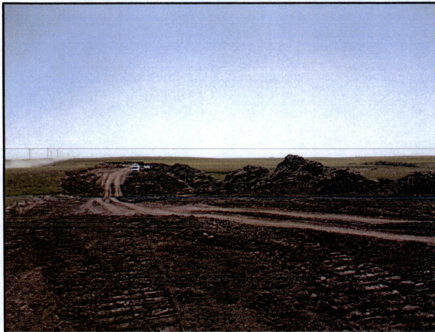
Photo 2. (GPS Point #446) – Drainage area intersected by ROW. No erosion control devices were in place and the corridor had not been necked down in this area to reduce disturbance. Direction: East.
