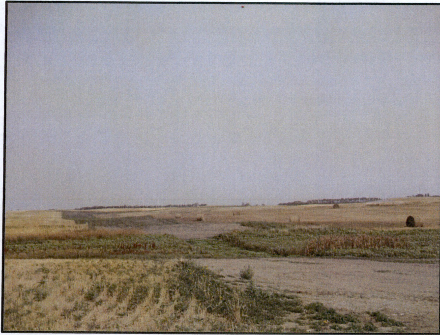
Photo 23. (GPS Point #488) - No erosion control devices observed. Area appears to have been bored but it looks like the wetland was driven through.
