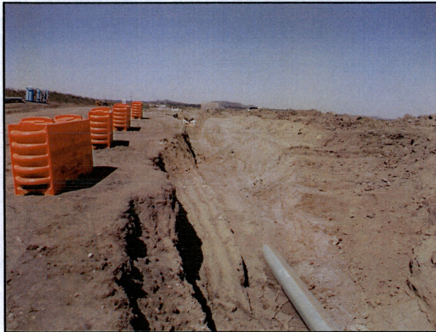
Photo 10. (GPS Point #450) - Open trench with partially covered pipe in trench. Orange safety blockades to the left of photo. White and black pipe rollers (visible in trench in far distance of photo) were used to guide the bore pipe into bore hole. Direction: West
