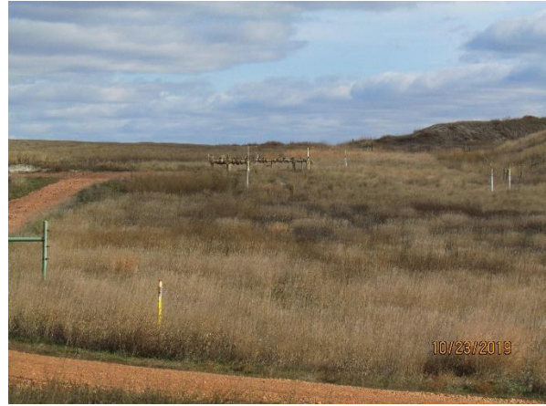
Photo 8: Pipeline restored corridor and Midway facility. (Section 7, T149N, R98W)
