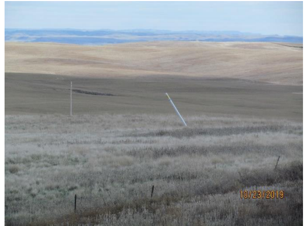
Photo 2: Leaning pipeline identification marker (Section 5, T150N, R99W)
