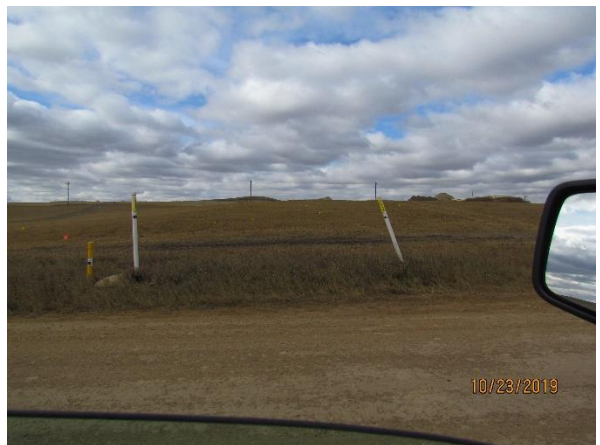
Photo 6: Leaning pipeline identification marker (Section 34, T150N, R97W)
