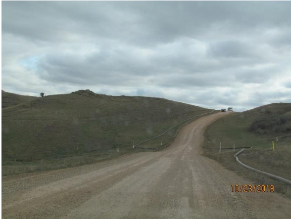
Photo 7: View of pipeline corridor (Section 33, T150N, R97W)
