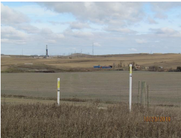
Photo 3: Pipeline corridor located south of Johnsons Corner facility; looking south. (Section 26, T150N, R96W)
