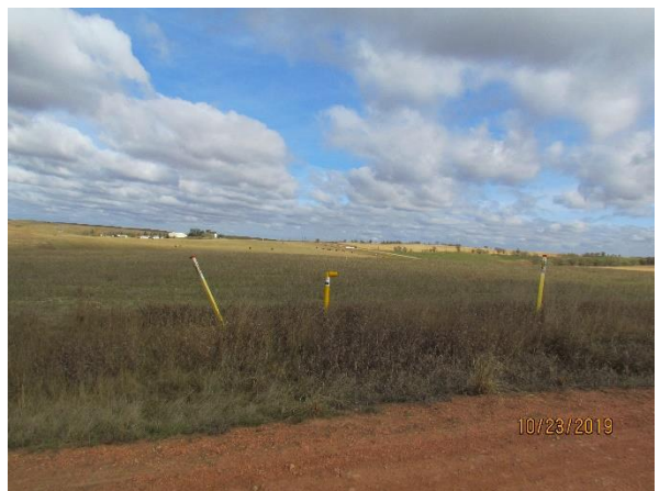
Photo 4: Leaning pipeline identification marker along restored pipeline corridor. (Section 34, T150N, R96W)
