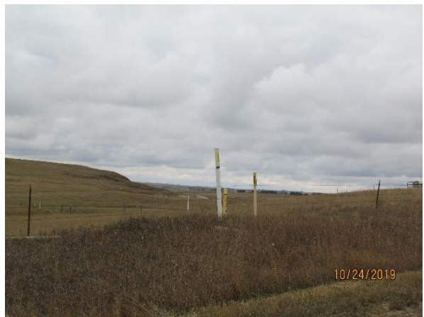
Photo 10: View of restored pipeline corridor (Section 35, T152N, R101W)
