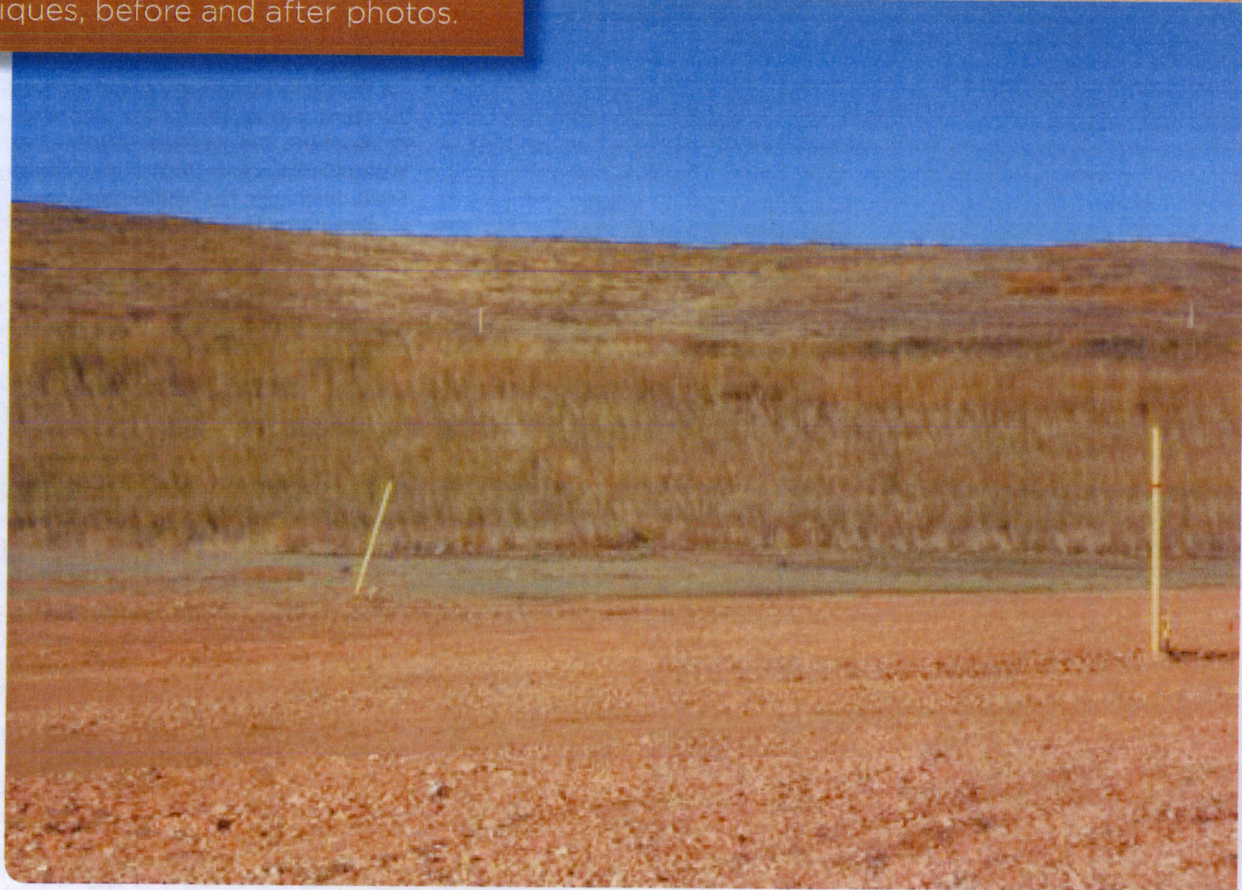
Final restoration with erosion control structures removed
